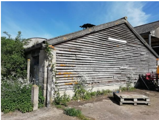
Plate 1: Barn 1 exterior with view of timber boarding on east gable
