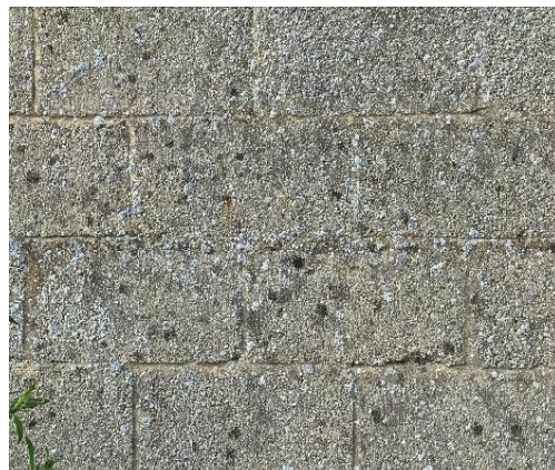
Typical existing concrete block detail (before repointing)
