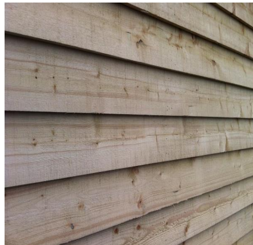
Typical square edged boarding detail
