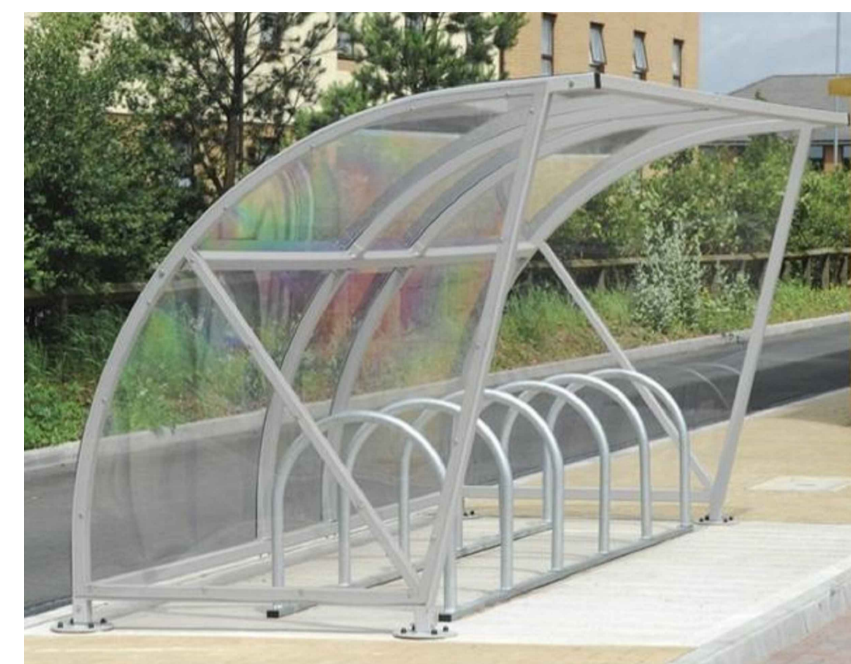
Photograph of Typical Cycle Shelter
