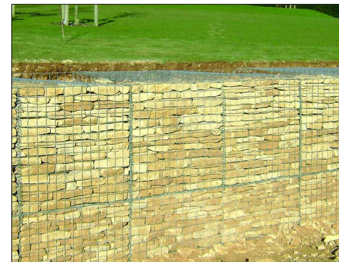
EXAMPLE OF GABION WALL SCALE: -
