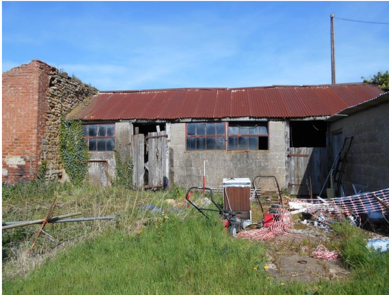
Fig 13: Building 7 of the 1970s, looking north; scale 1m. To the left is the ruinous Building 6 and to the right Building 8.
