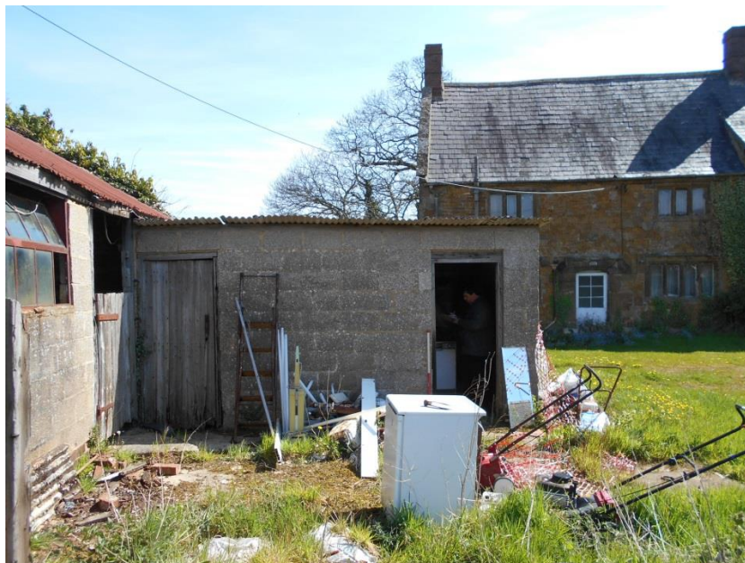
Fig 14: Building 8, looking east, the farmhouse beyond; to the left is Building 7
