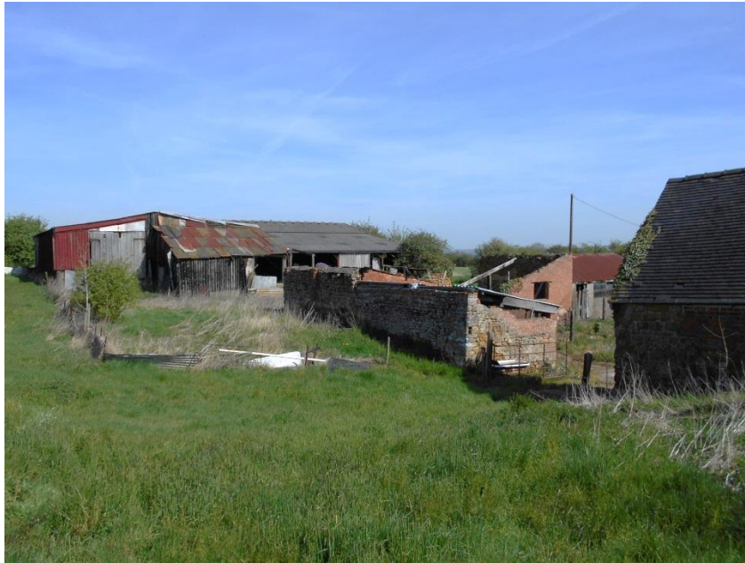
Fig 19: The public view of the farmyard from a footpath to the south-west; Building 5 is in the centre, Building 9 to the left; Building 4 to the right blocks views of the farmhouse.
