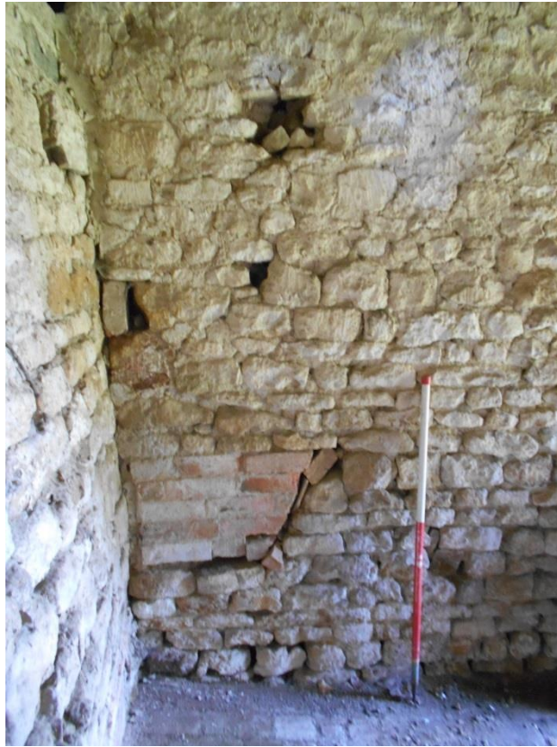
Fig 4: Scars of former manger and hay rack in Building 1 dividing wall; scale 1m
