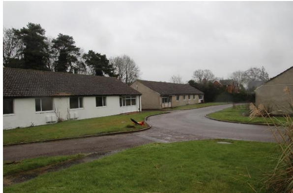
2. Northern end of site looking east
