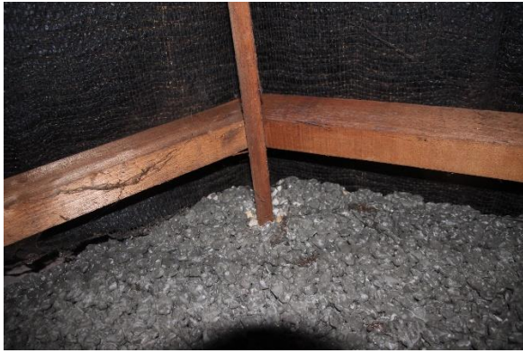
9. Ridge board under felt lining with sprayed concrete wall
