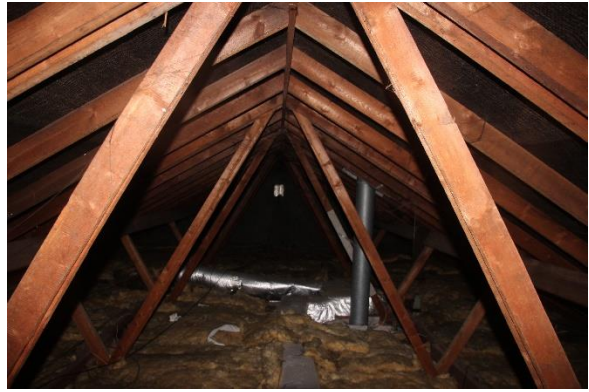
10. Collar roof space with well-spaced trusses
