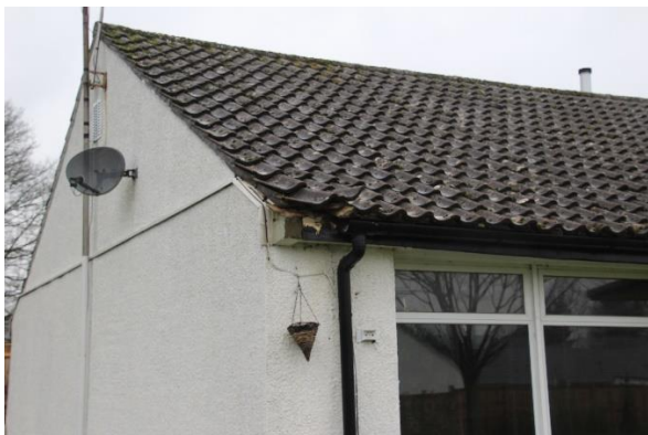
7. Gable end with grill above satellite dish
