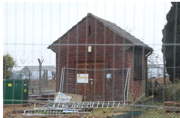
8. Detached single brick building with air hole
