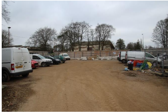
2. Hard standing in Phase 5D
