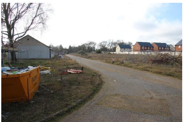
8. Looking south across Trenchard Circle
