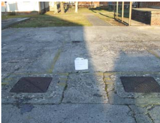
Photo 9 (left) showing tanks UGNSA 31-33
