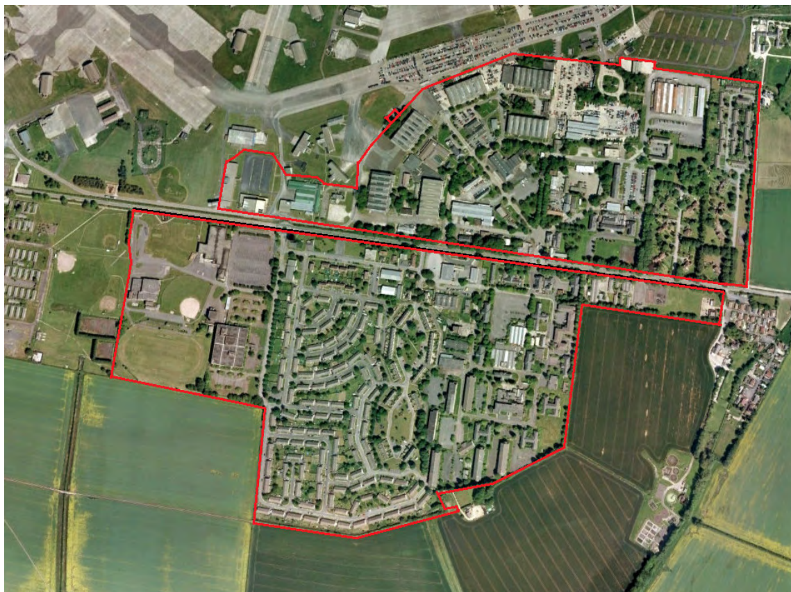
Figure 3.2. Recent Aerial Photograph
