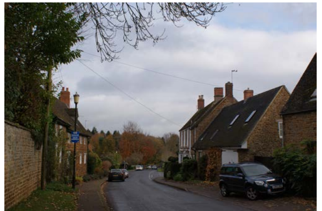
Traditional terraced properties along Cross Hill Road
