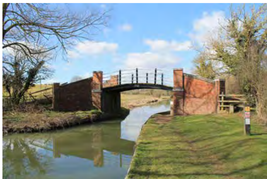
Listed Canal Structures
