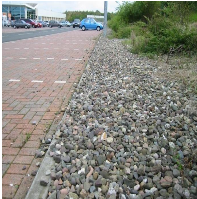
Figure 4a: Permeable paving
