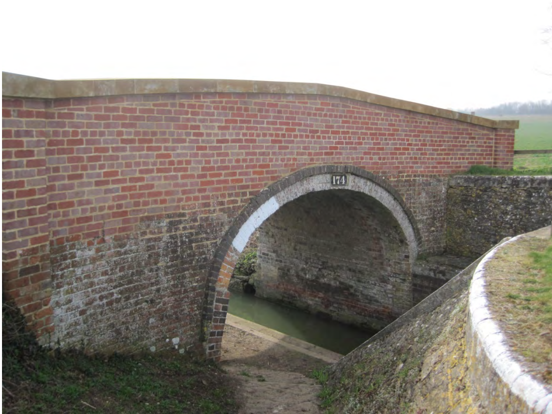
Plate 2: Bridge at Grant's Lock
