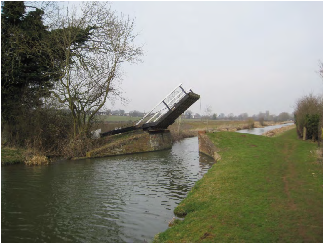
Plate 1: Typical lifting bridge on Oxford Canal
