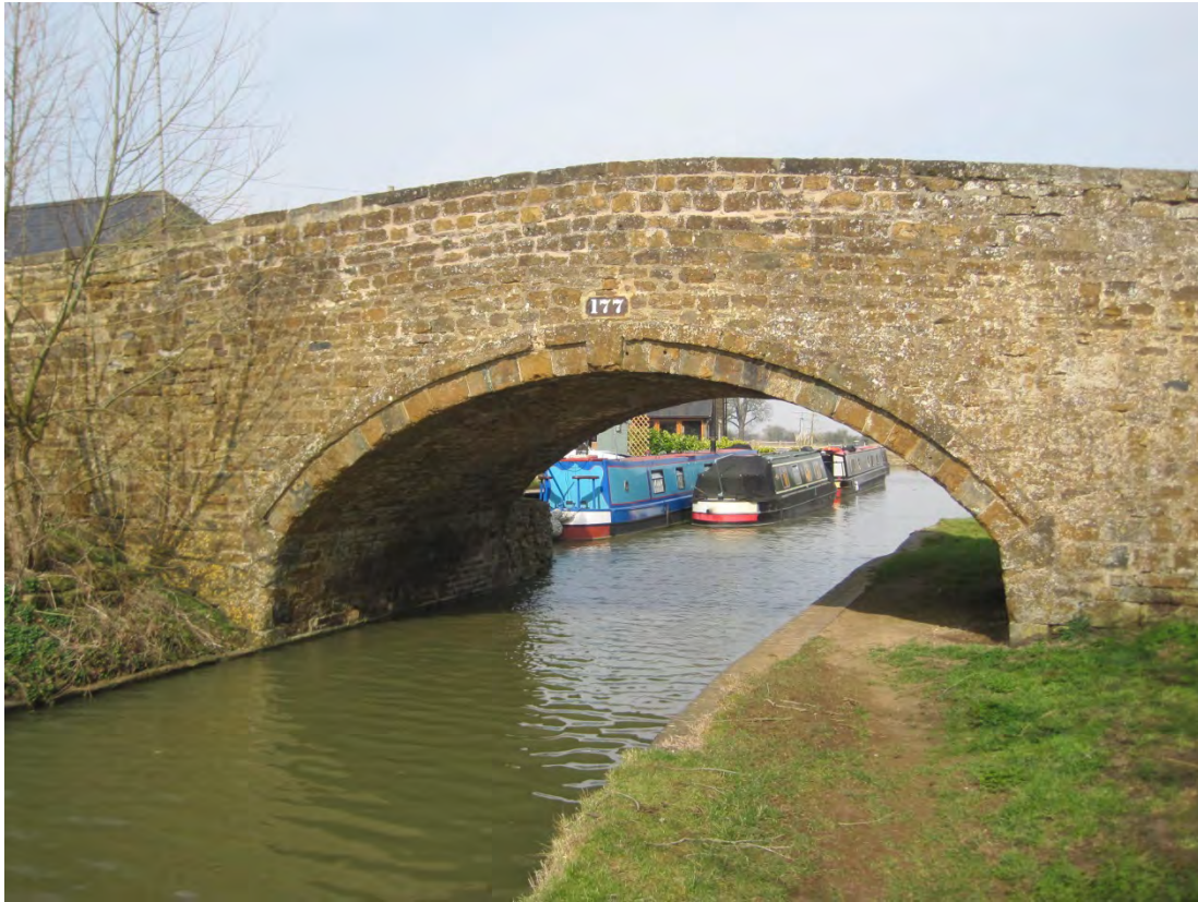
Plate 3: Bridge at Twyford Wharf
