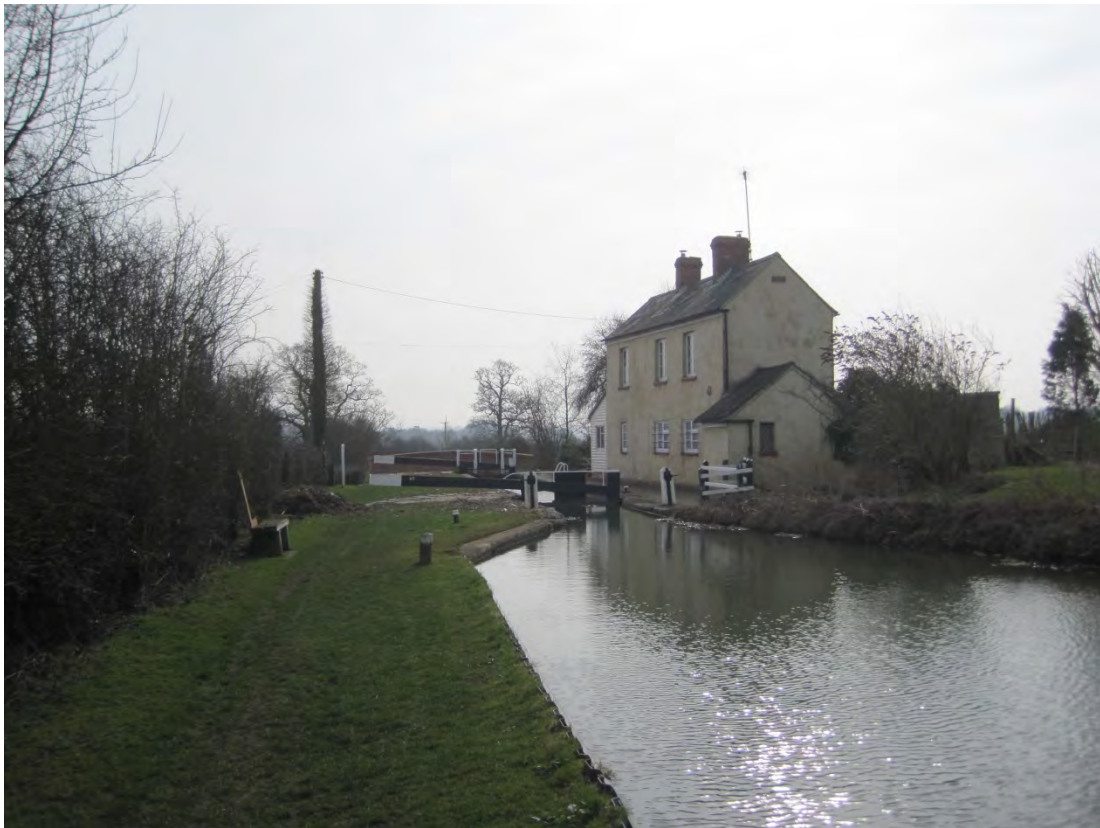
Plate 8: Lockkeeper's cottage and Grant's Lock
