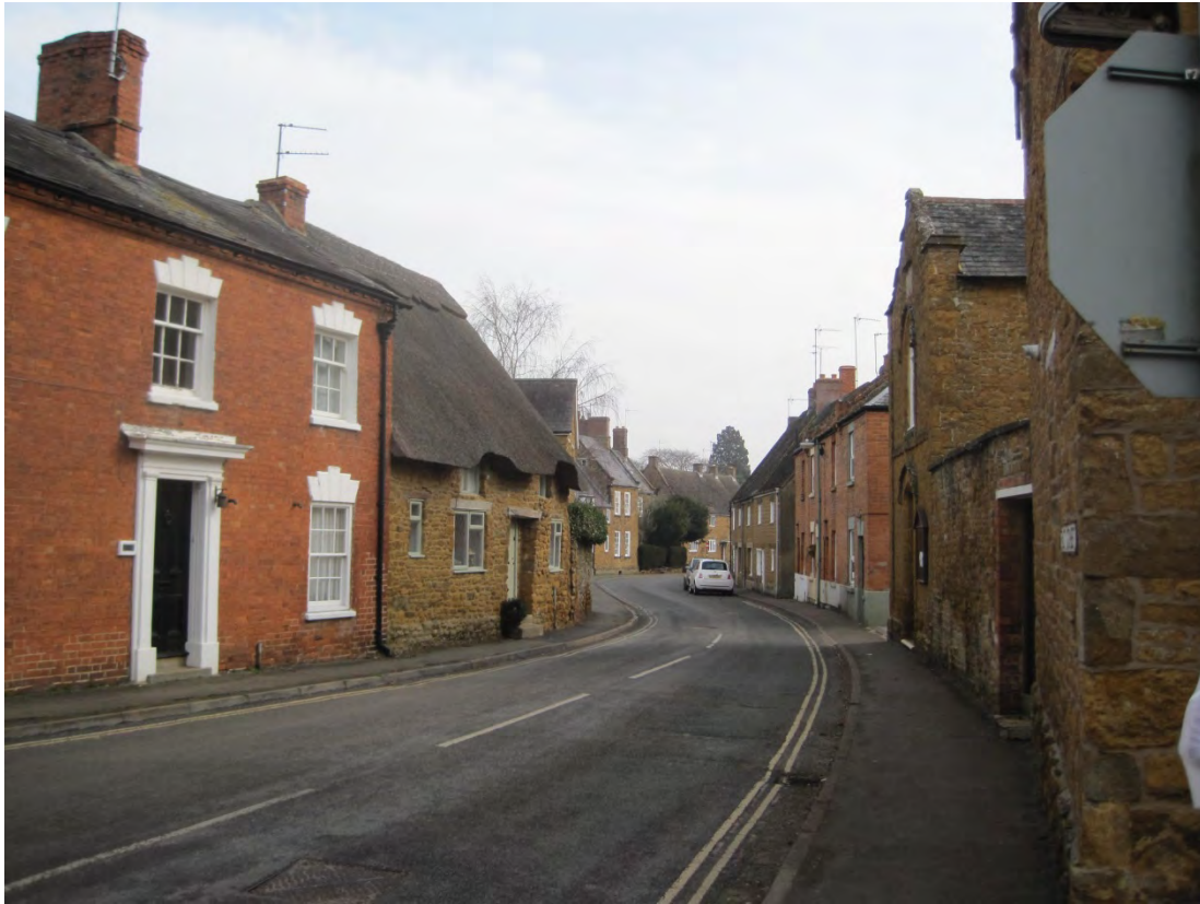
Plate 5: Street view within Bodicote Conservation Area
