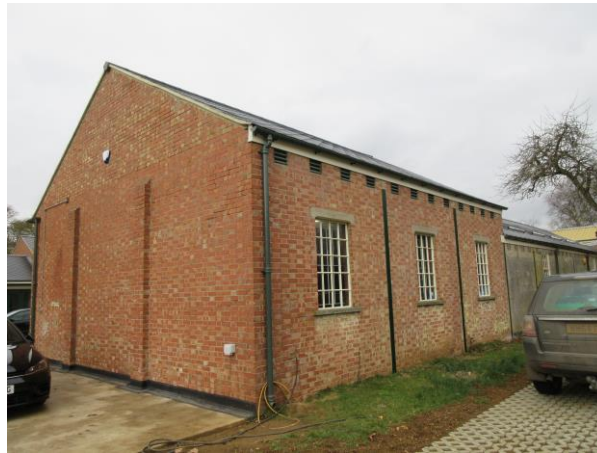
Proposed car port will be in front of the rendered building to the right
