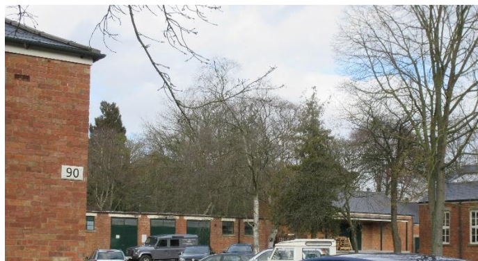
Building 97 seen from the south
