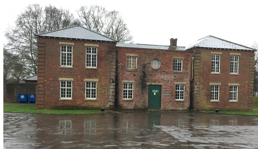
Building 147 as existing
