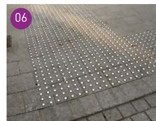
06 Blister Paving (Rivets into paving)
