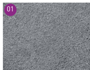
01 Macadam road surface
