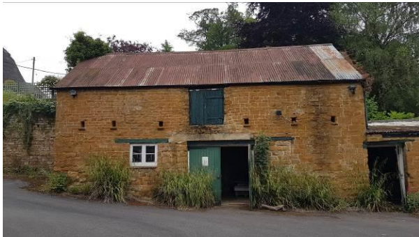
18. External view of barn
