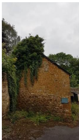
20. External view of barn
