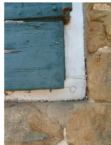
mortice and tenoned pegged joints
