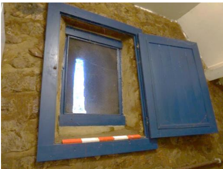
Gable end wall, lancet, fixed glazed window Scale 50cm
