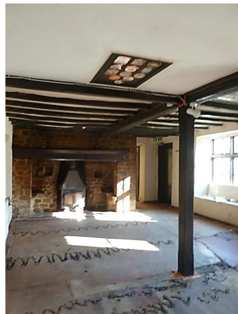
ROOM D View East
