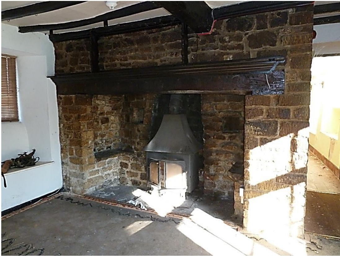
Large Inglenook with large chamfered bressumer beam
