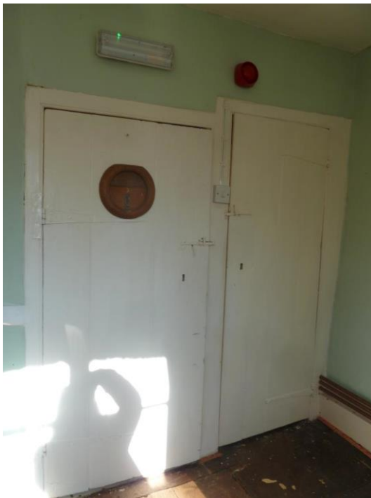
C17-C18 X2 Doors. Main Door and Cupboard
