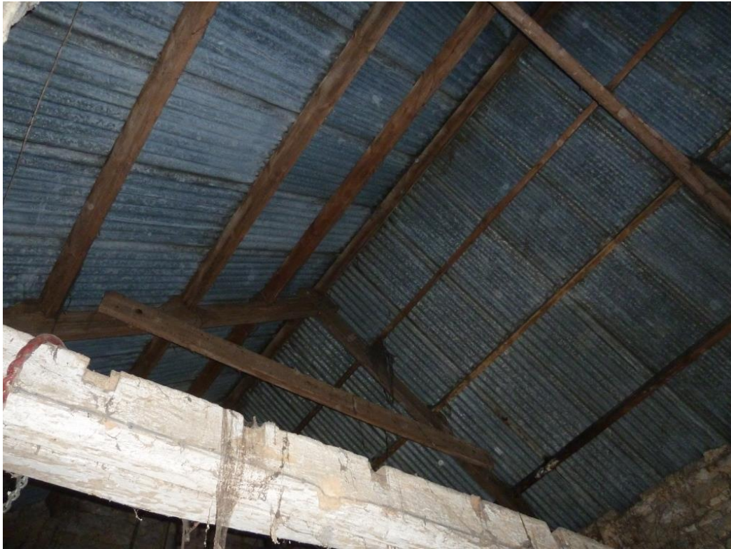
Evidence of former floor for second storey/ corrugated roof
