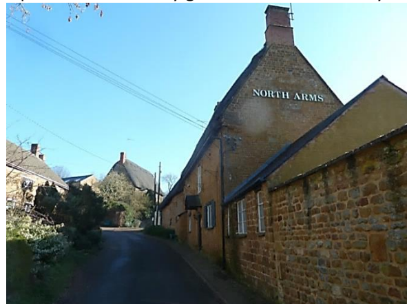
View up Mills Lane Gable end of North Arms
