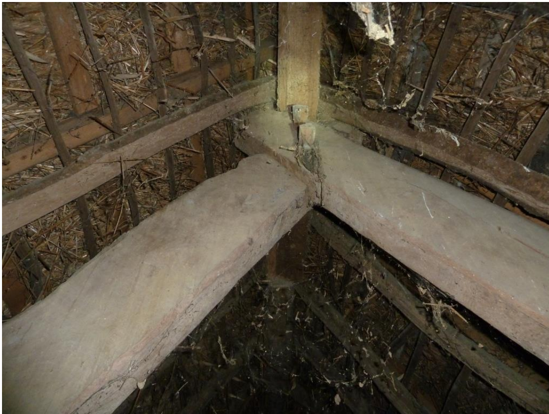
Cruck Blades seen from inspection hatch in Room M
