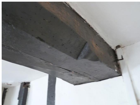
Central chamfered beam with ogee stop
