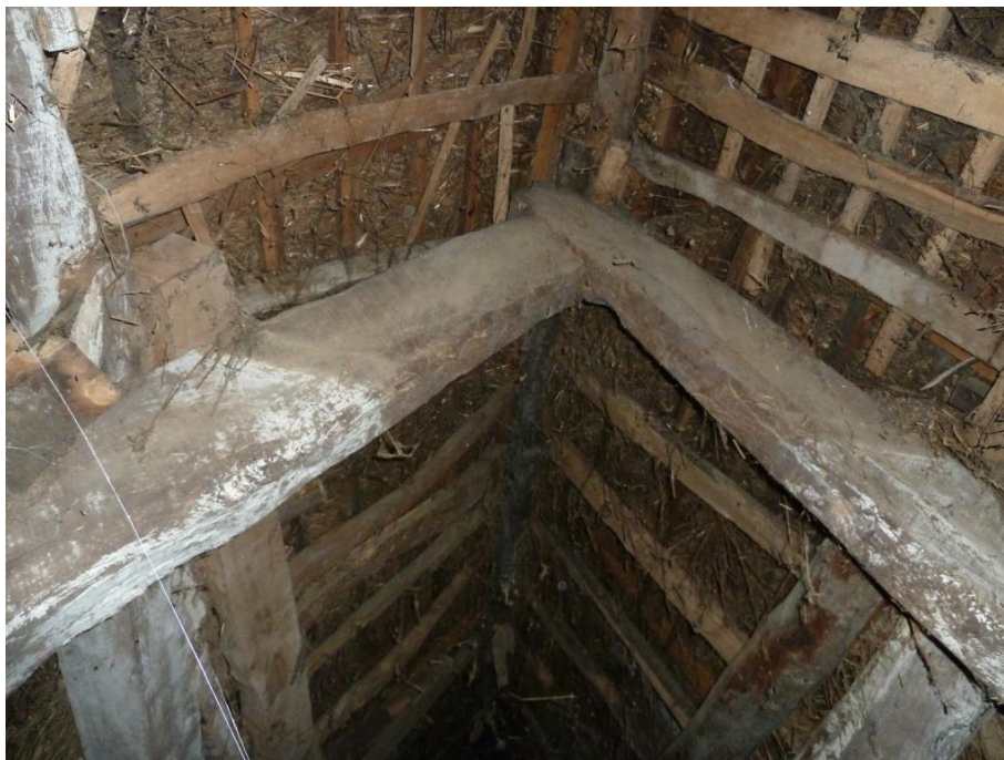
Cruck truss within the Roof area over H and G
