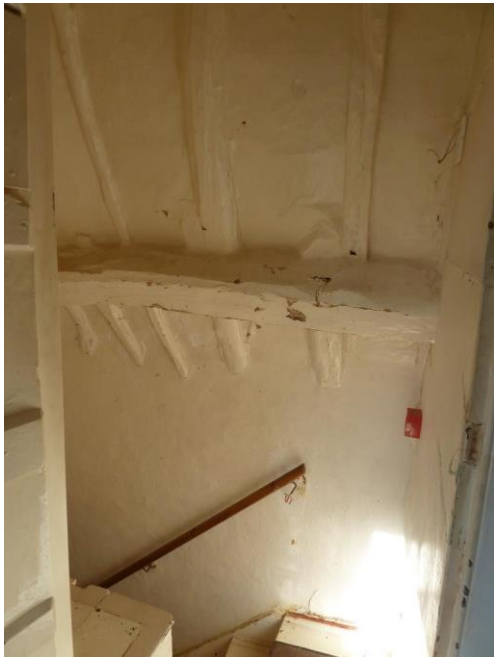
Roof timbers on stairs exposed and limewashed ceiling and wide timber boarding.
