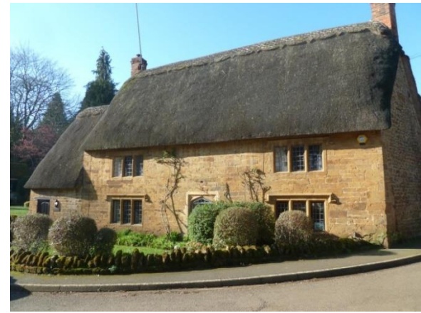
Mullions stone mullioned windows and coursed squared ironstone by gates to Wroxton Abbey
