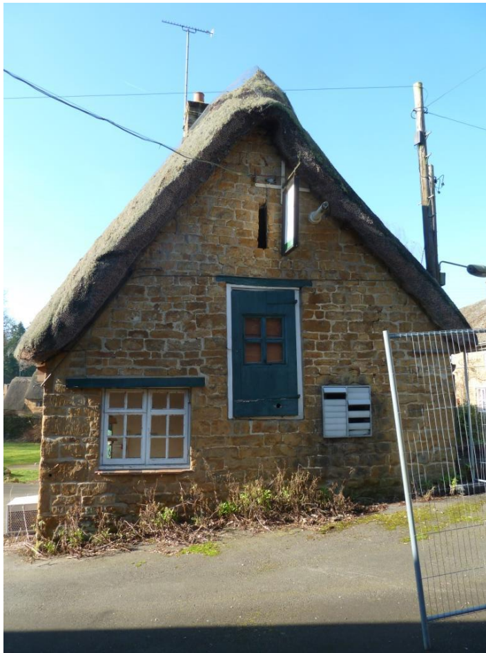
Gable end of Thatched stone building; x2 storey ; semi basement
