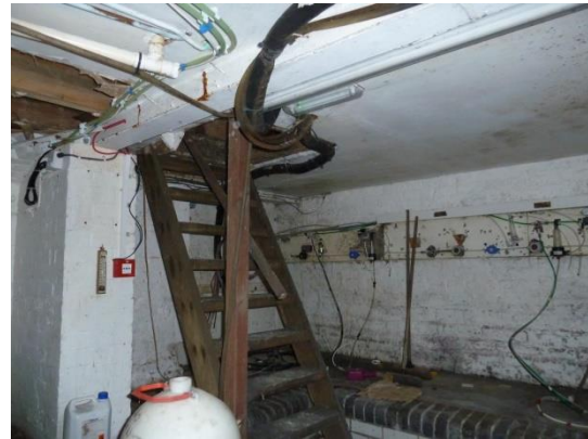
Cellar accessed via timber ladder steps from a floor hatch
