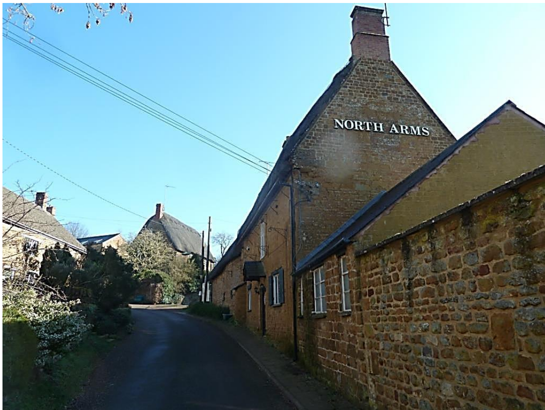
Photo West Elevations to Mills Lane
