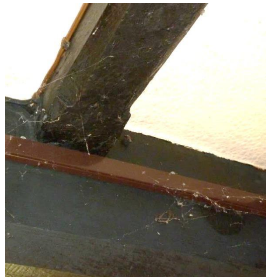
Chamfers to floor Joists
