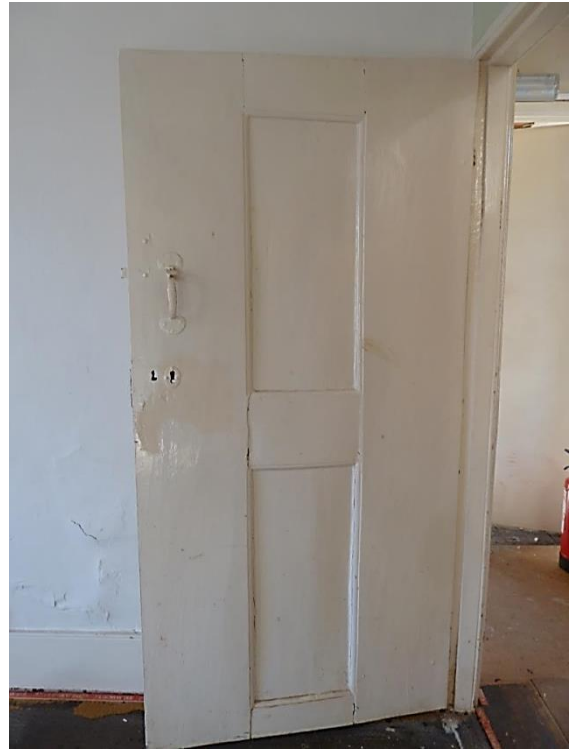
ROOM I C17 door with an applied panelling with moulded fillet
