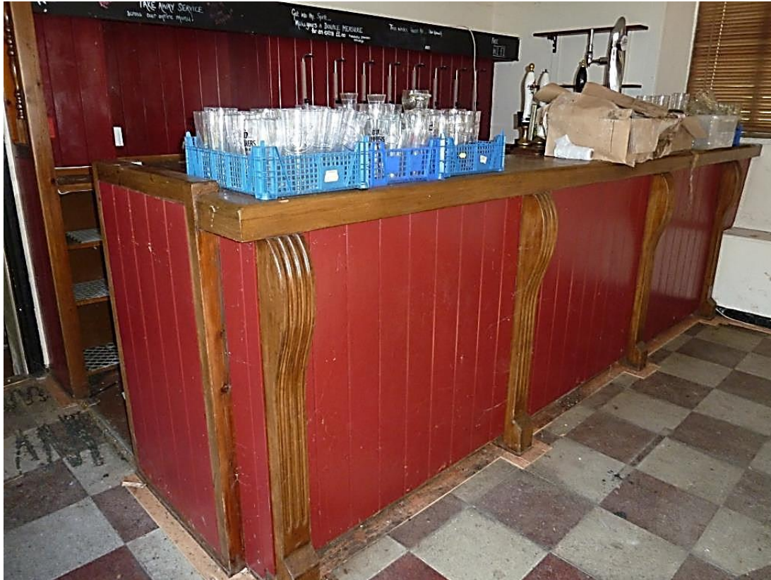
Former [painted] timber Bar with access in floor to Cellar below
