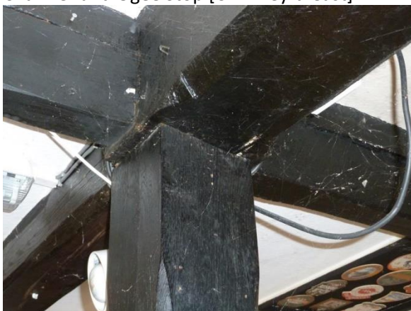
Chamfers and stops
