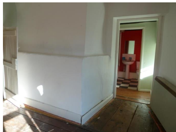
ROOM I Large chimney stack
