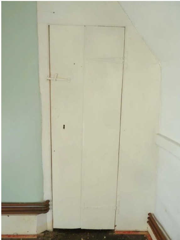
LH of Chimney Breast x2 C18 plank door with strap hinges and latch.
