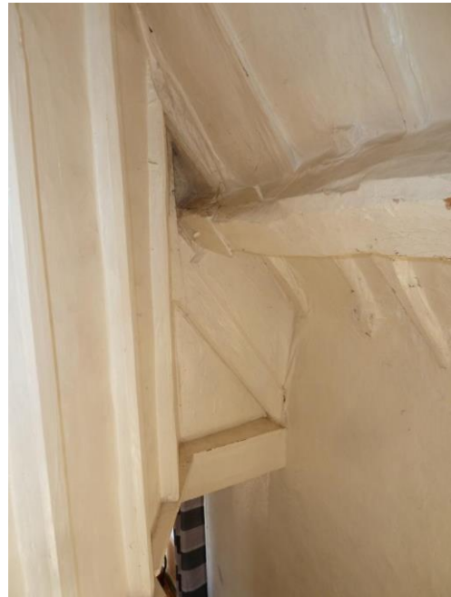
Roof timbers on stairs exposed and limewashed ceiling and wide timber boarding.
