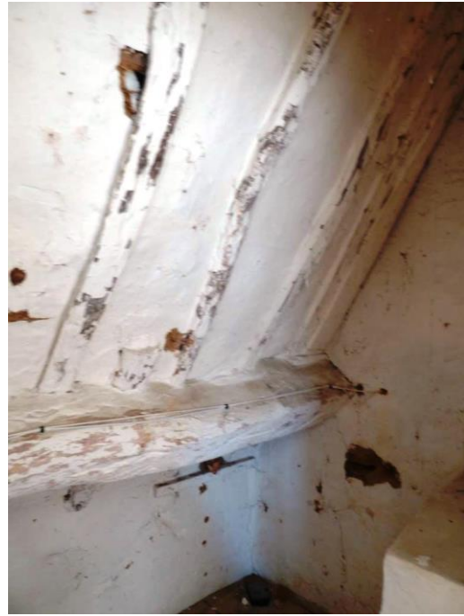
Cupboard to Eaves LH of Chimney
