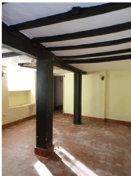
ROOM C View West
