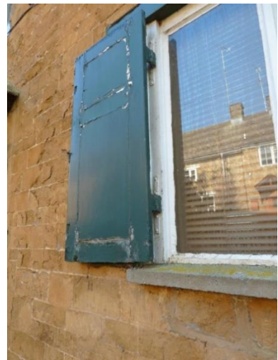
Shutters; possible early C19 Concrete sill/ C20 window pane.
