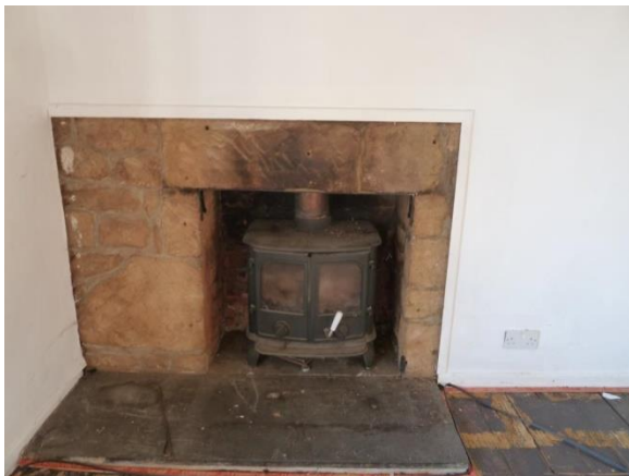
Fireplace opening inserted in stone wall
