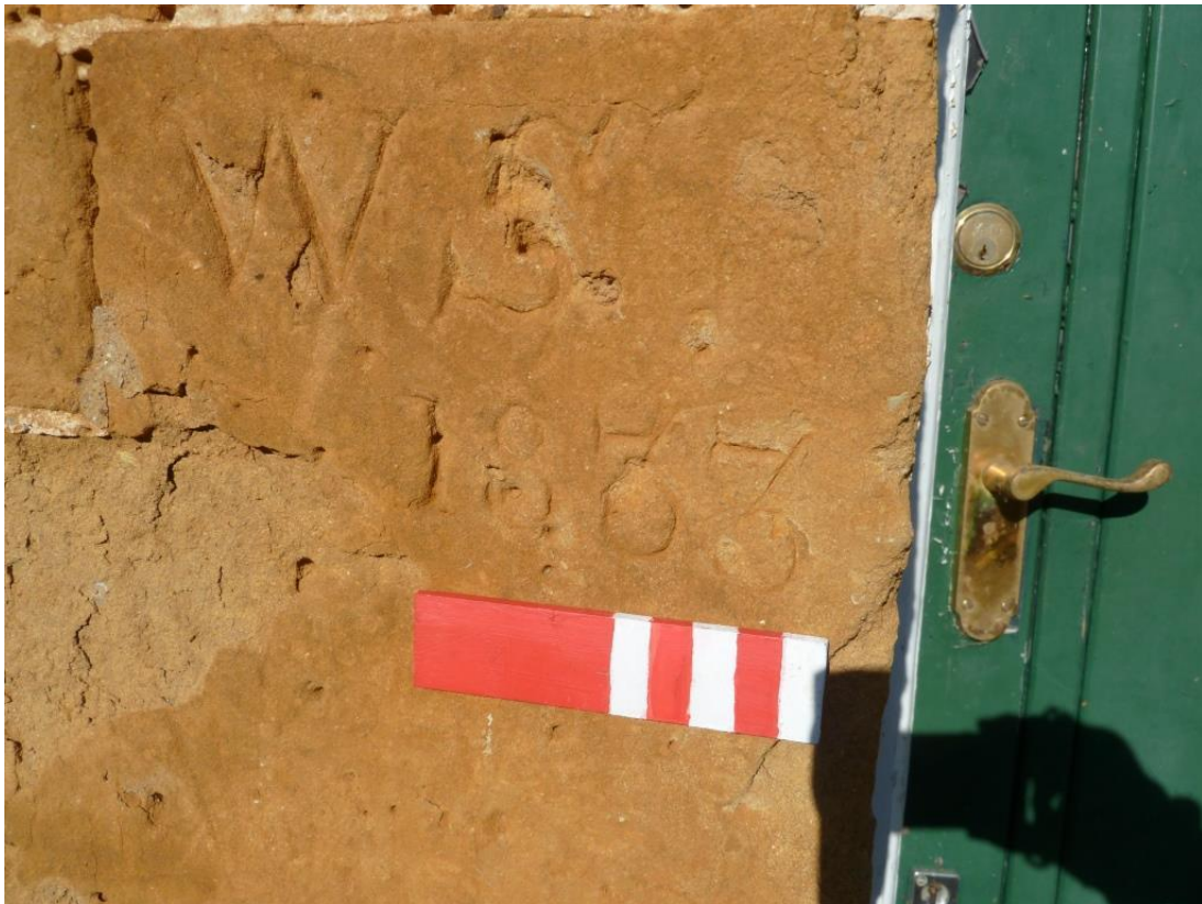
GF entrance door has stone lintel and graffiti inscribed on the left door jamb date 1833 and initials WS. The door is C20 plank. Photographic Scale 10cm
