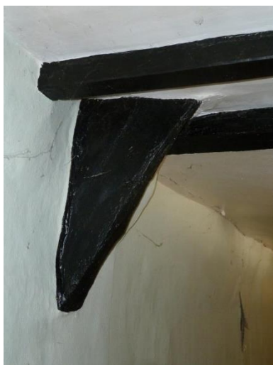
G possible raised cruck [Landing][See Roof Void]
