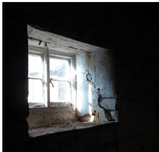
C19 Casement window internal view
