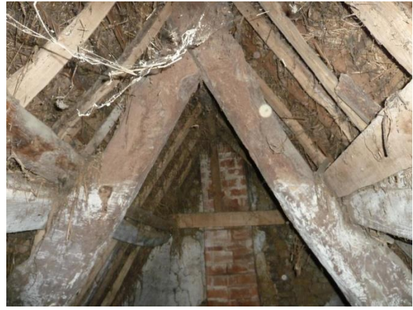
Evidence of limewash View to East and a brick Chimney stack
