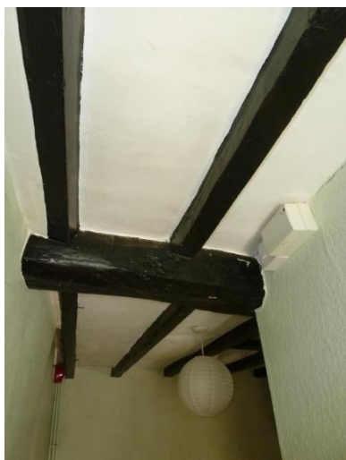
G central beam and joists.
