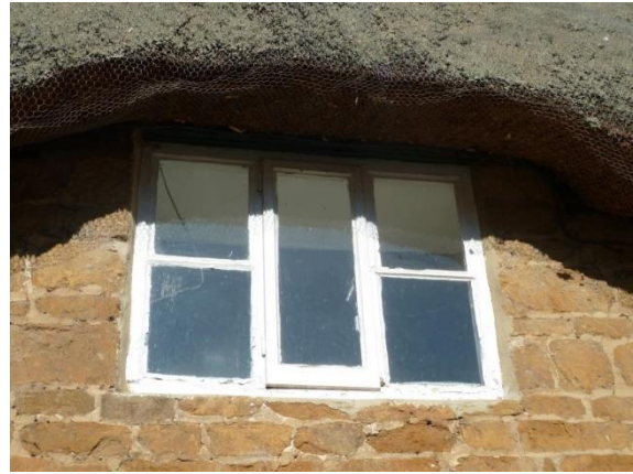
One window opening at eaves/attic that maybe of some C18/C19 origins.
