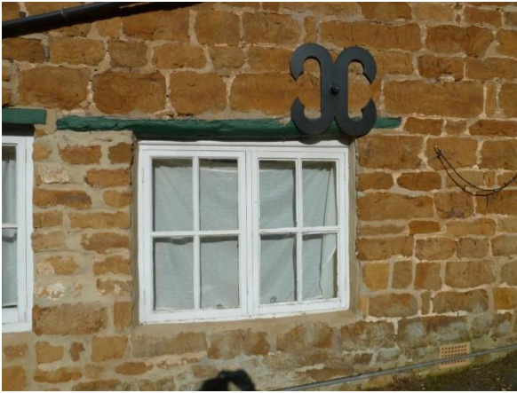
Example of Window openings with timber lintels
