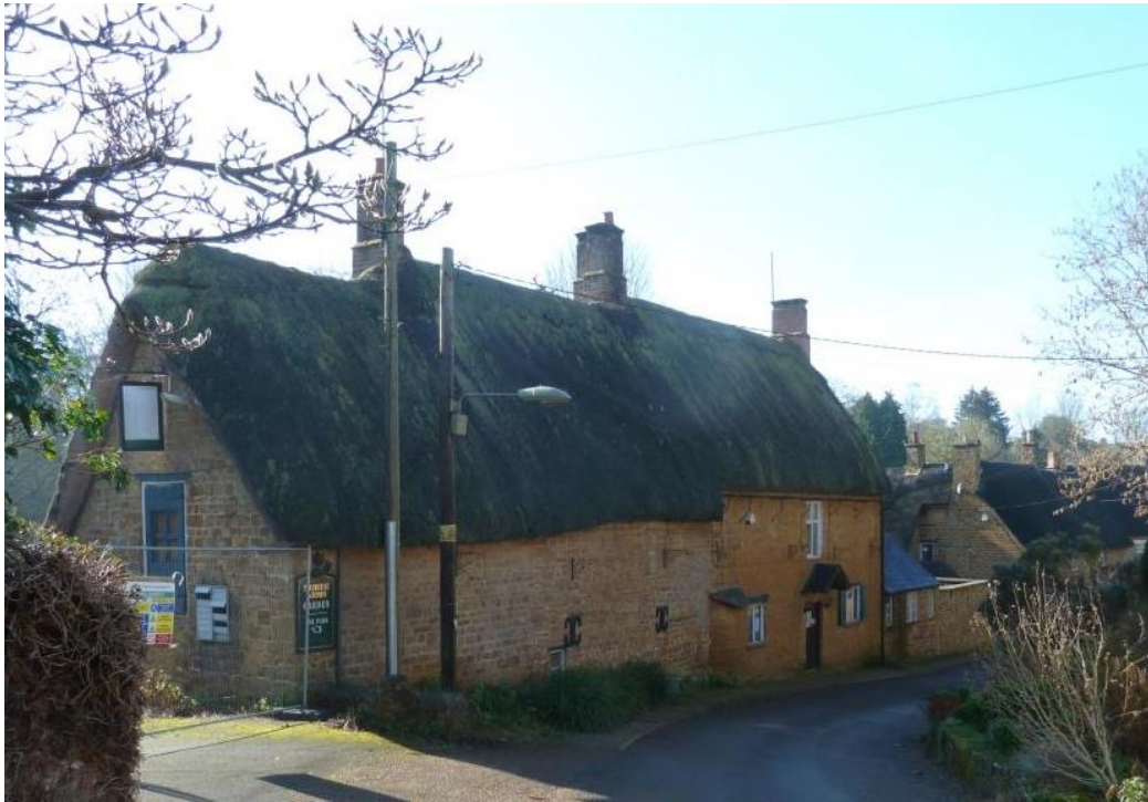
Photo North/East Elevations to Mills Lane
