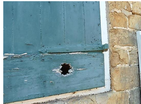
Iron spear headed brackets on pintles
