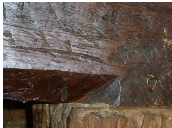
Fireplace Bressumer Beam chamfer and stop
