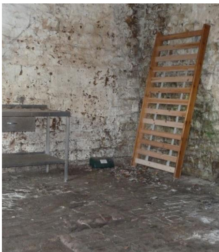
Some floor is historic laid to bricks
