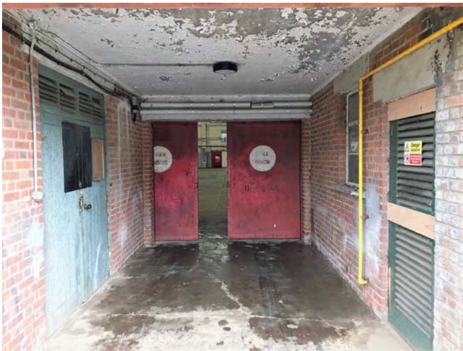
Exterior view of existing sliding steel doors to be retained.
