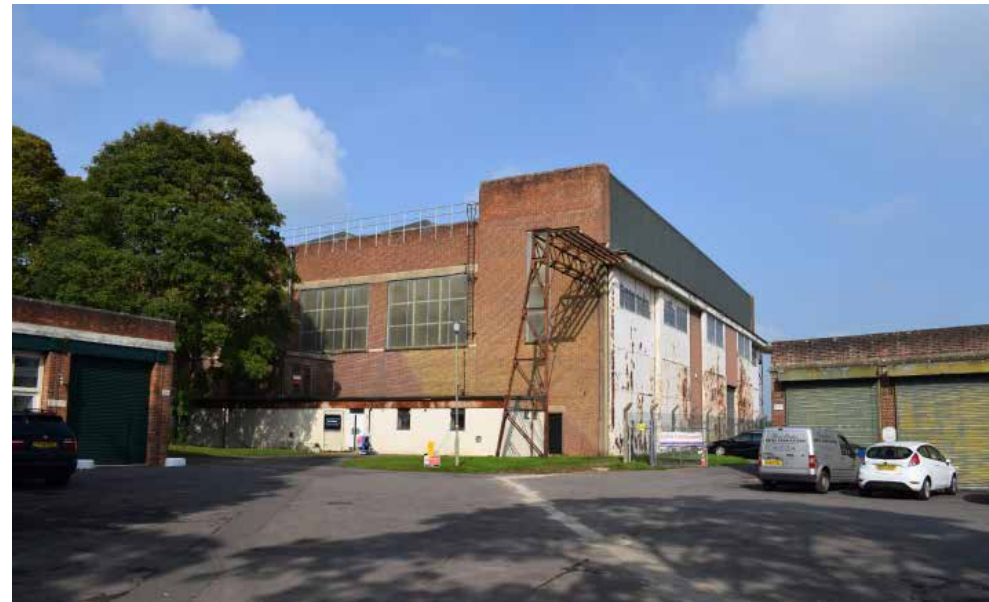
Fig 18: Northern most C Type Hangar
