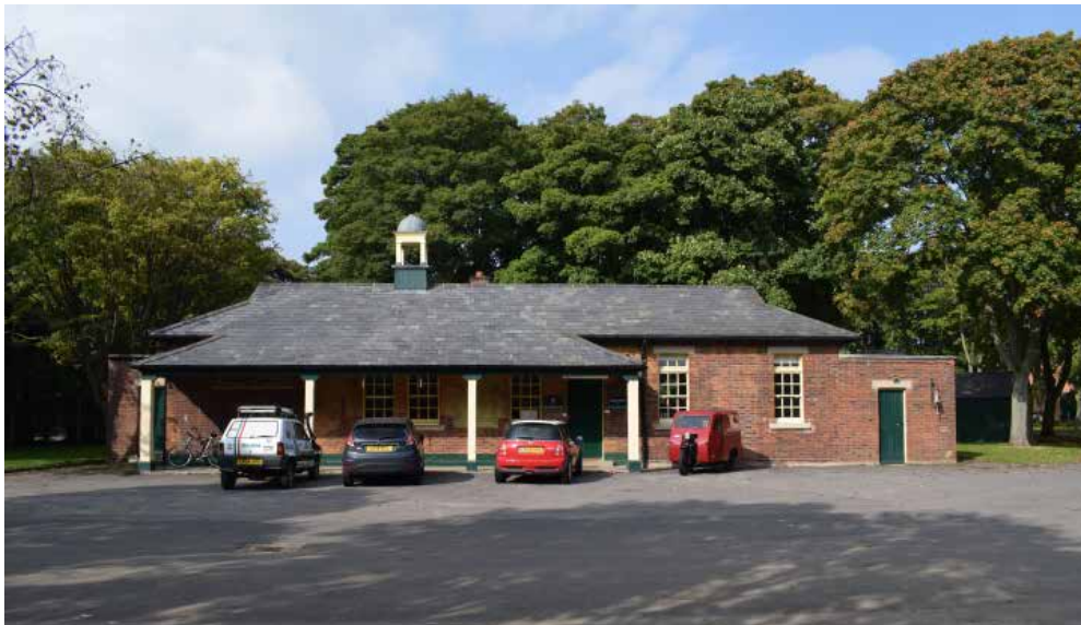
Fig 10: The Guard house, prominently sited at the entrance of the site and built in a neo-Georgian style thought commensurate with the activities carried out with it and with the status of its occupants.
