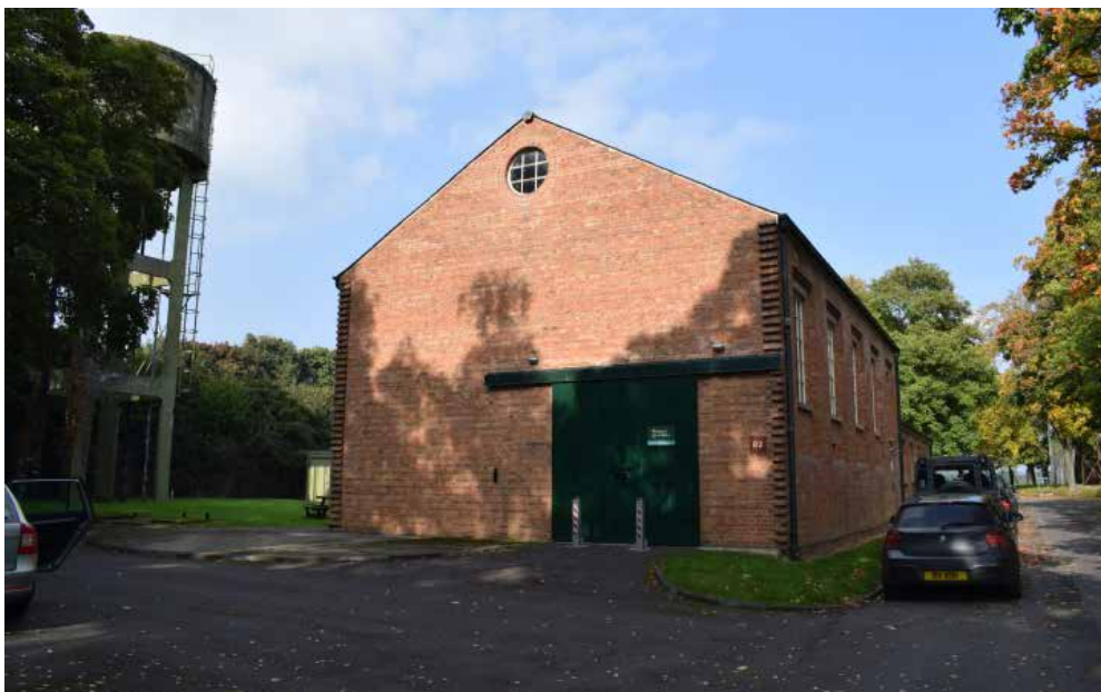
Fig 11: The Parachute Stores. The design of the building - featuring a high central area- is particularly informed by its function. The Stores at Bicester were a prototype, first seen here before being adopted in airfield sites elsewhere across the country.
