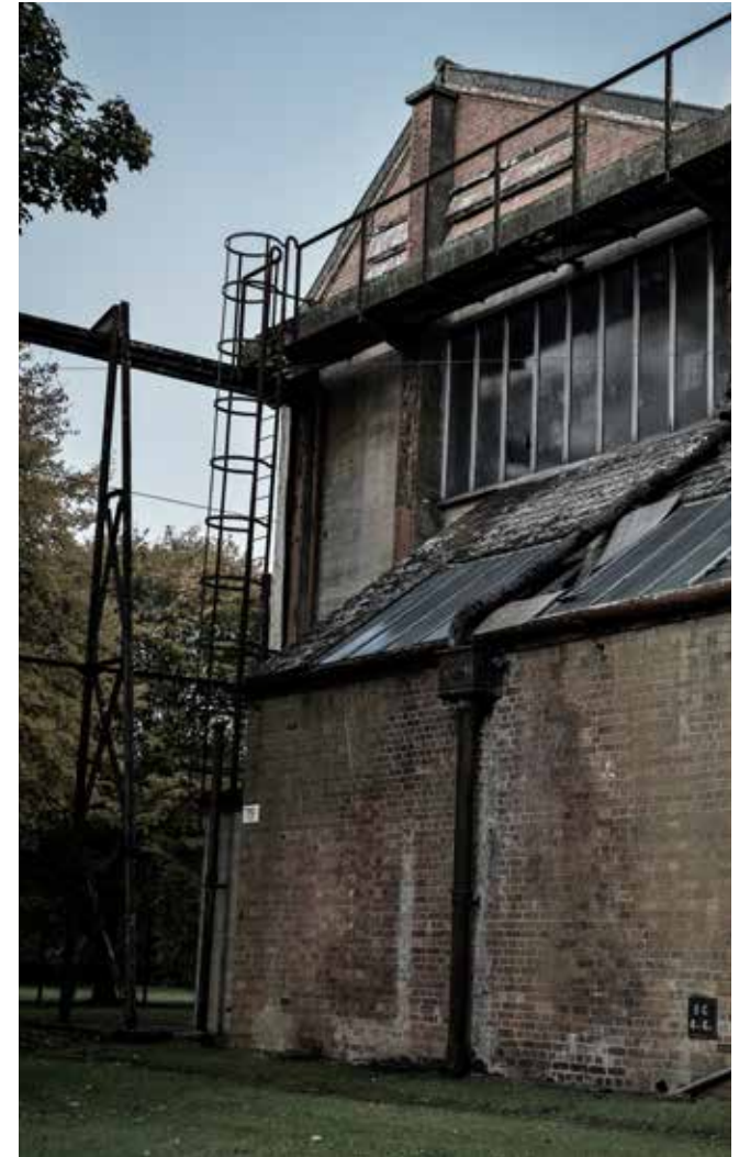
Fig 29: Type A Hangar
