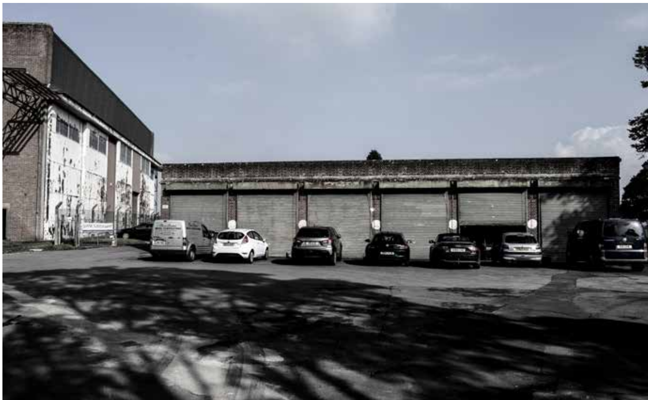
Fig 27: Ancillary buildings adjacent Type C hangar
