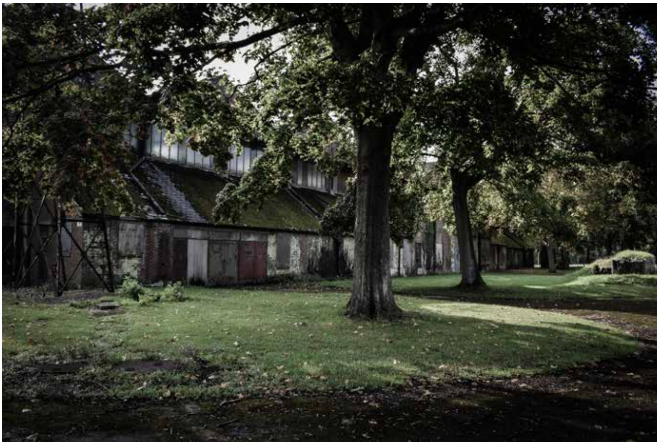
Fig 2: Type A Hangar
