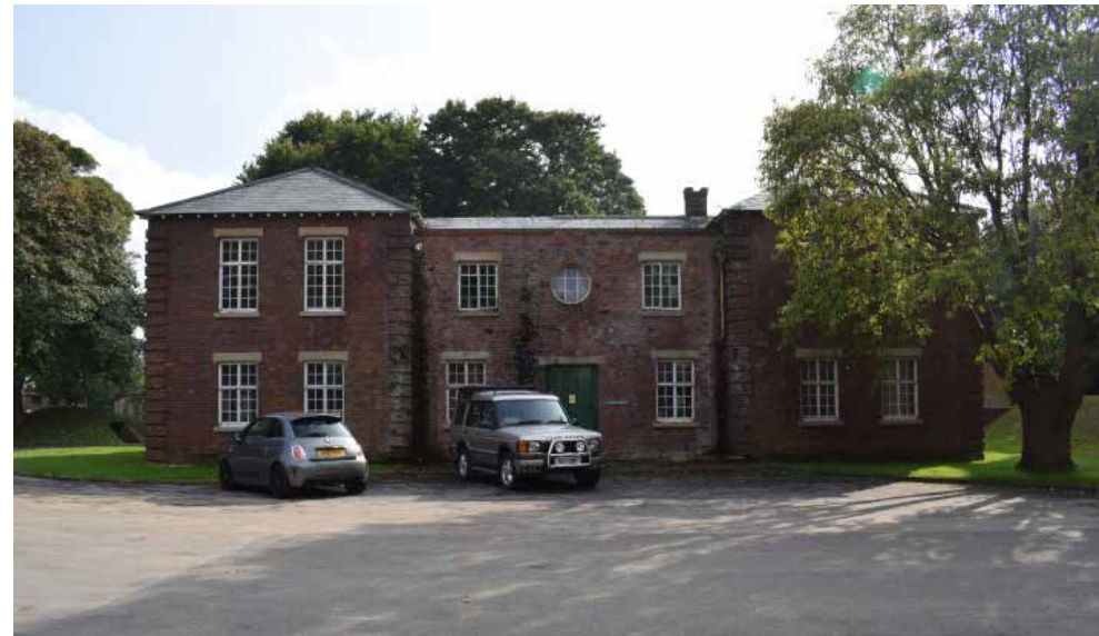
Fig 12: The Station Offices and Headquarters. Situated directly opposite the Guardhouse, the application of the neo-Georgian treatment to its design is also meant to symbolically emphasise the status of its occupants and serves as a strong visual marker of the relationship between the two buildings.
