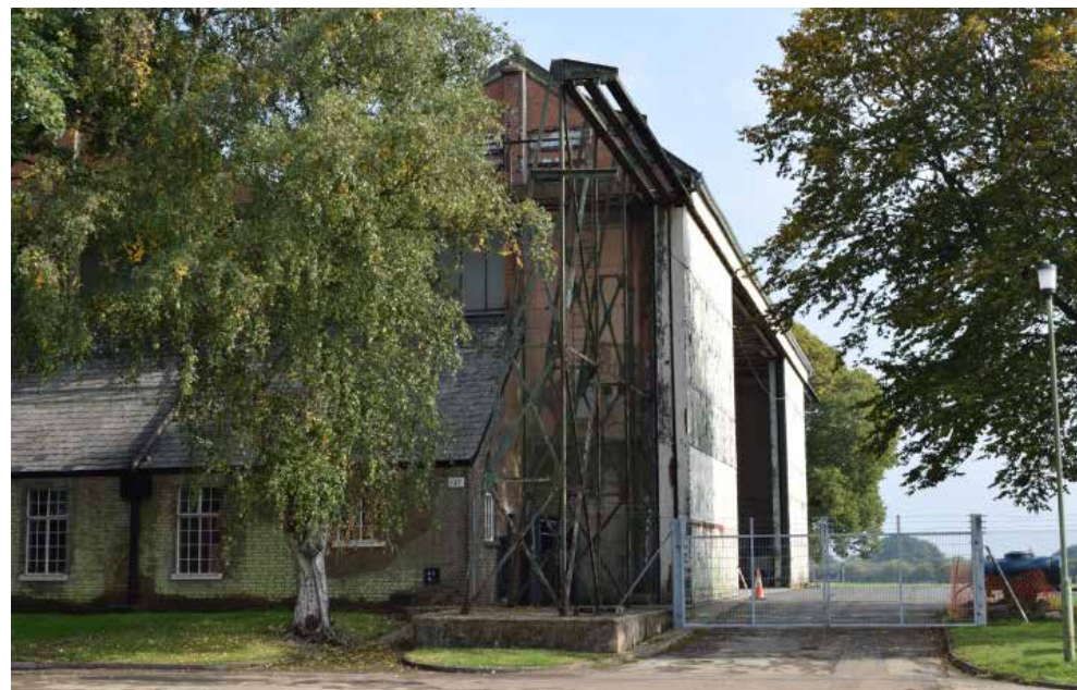
Fig 15: Southern most Type A Hangars
