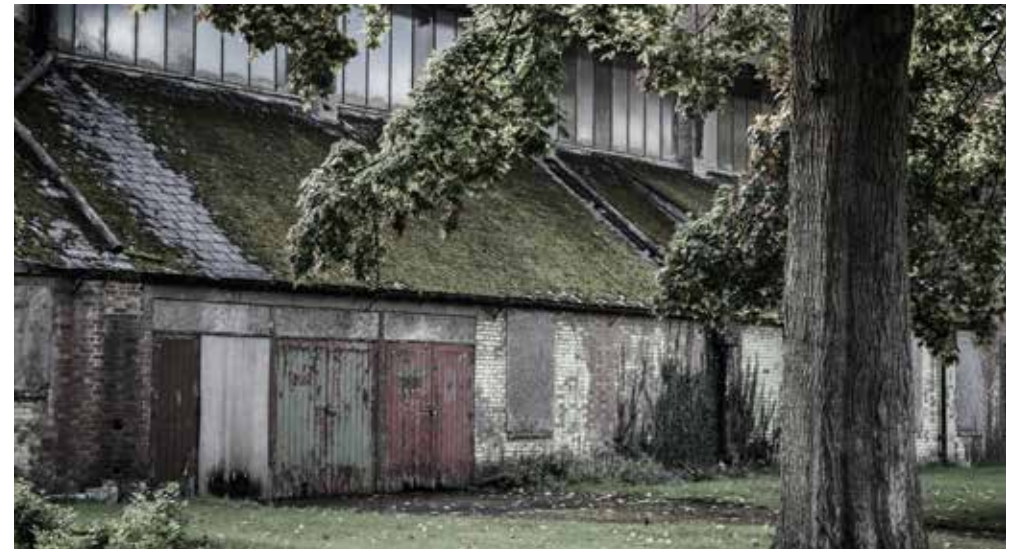
Fig 26: Type A Hangar
