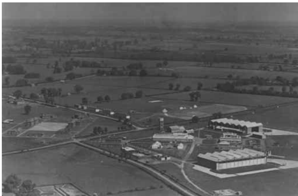
Fig 29: Photograph (probably 1930s) showing the early layout of the Technical site with Skimmingdish Lane forming the southern boundary. Note the young trees on the site lining the Avenue and along the lane.
