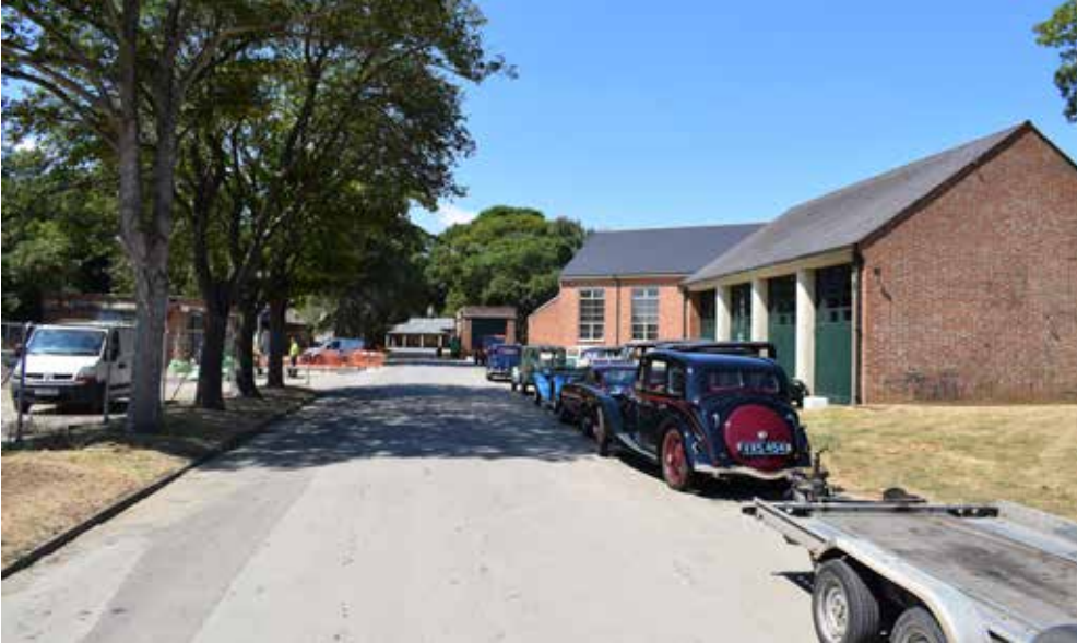
Fig 29: Looking down towards the Guards House. Note the use of brick off white painted window joinery and green painted door with the use of grey roofing materials.
