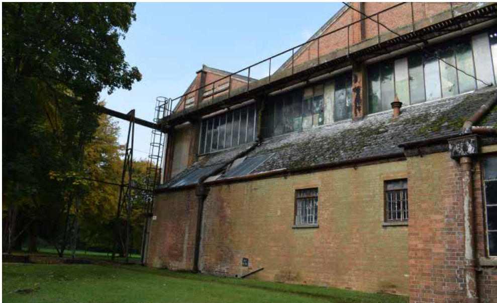
Fig 16: Western most Type A Hangar
