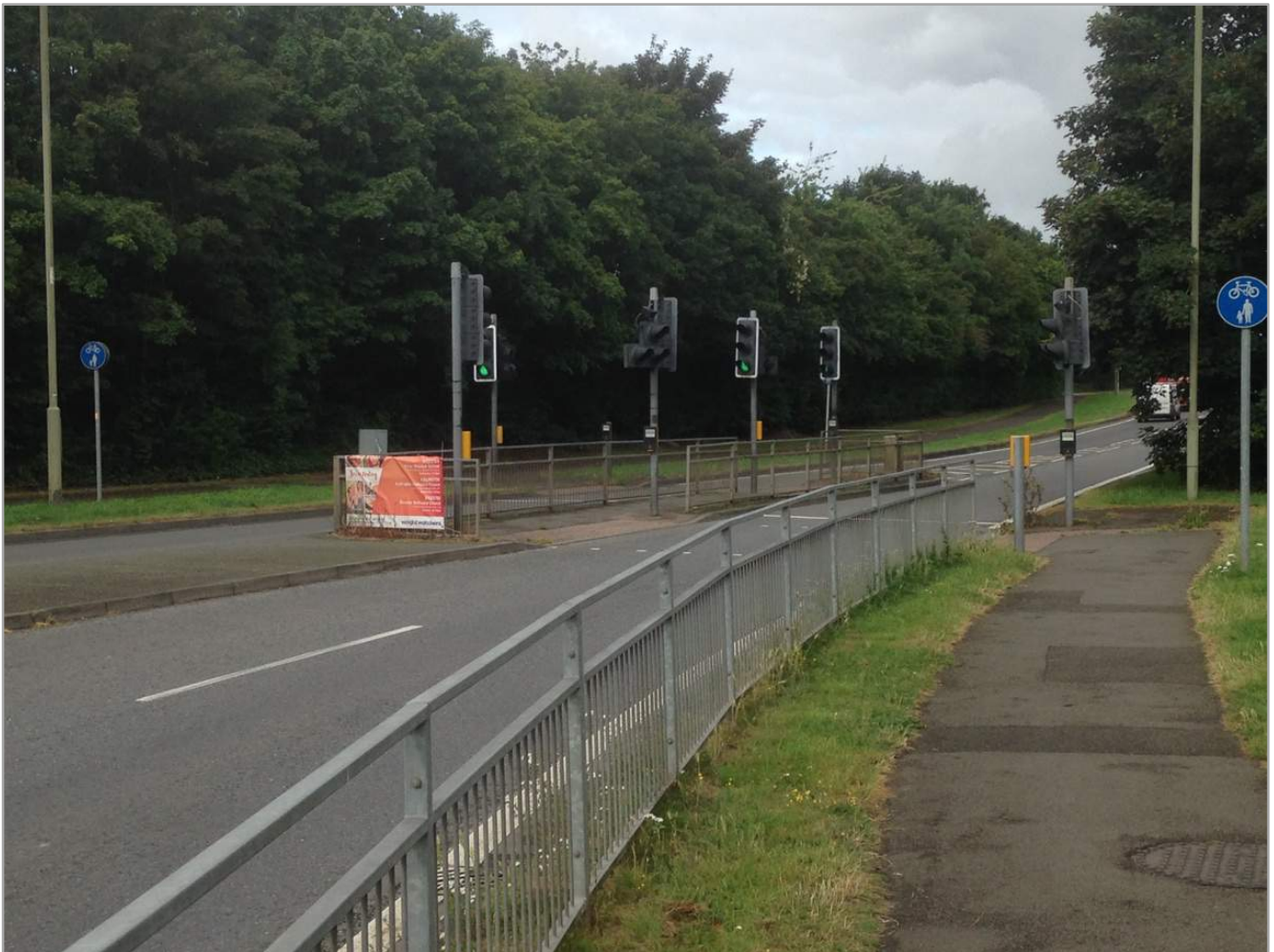
Figure 3.3: Existing Toucan Crossing
