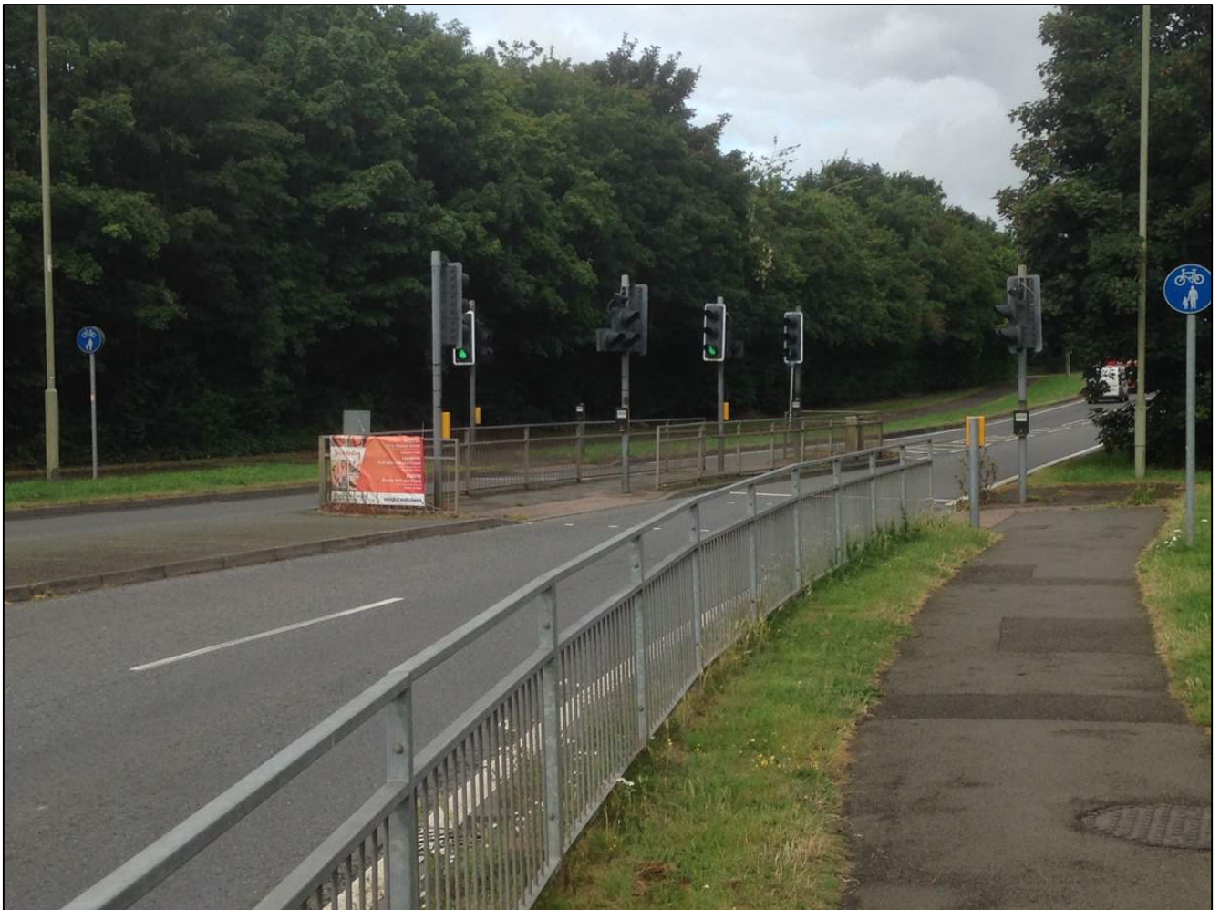
Figure 3.1: Existing Toucan Crossing
