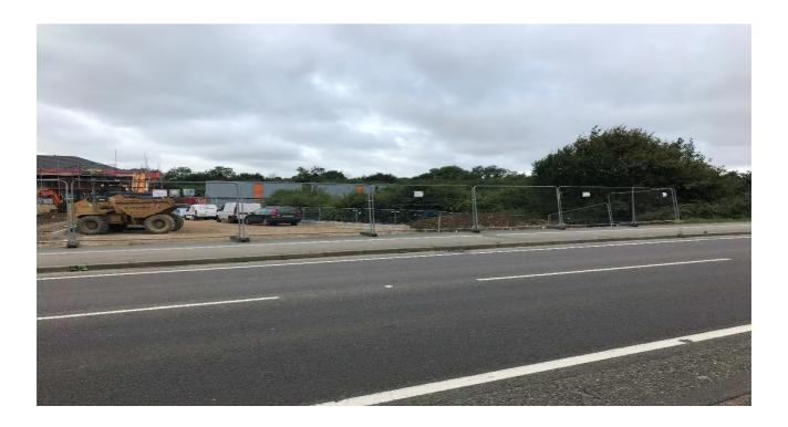
Video 05 is taken from the south elevation of the site and heading west to the existing bell mouth. It shows the existing verge and road. There is minor cracking to the tarmac road but generally it is in good condition. It also shows a lighting column that has been hit and the top two thirds removed.
