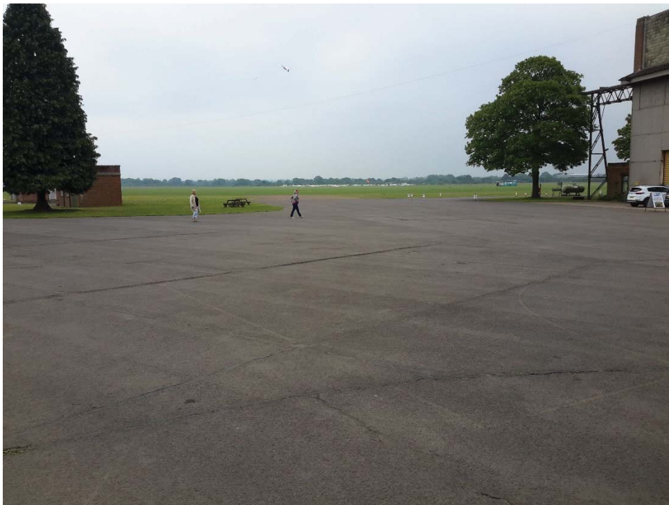
Plate 6 Concrete Hardstanding External to RAF Building (Looking Towards Airfield)
