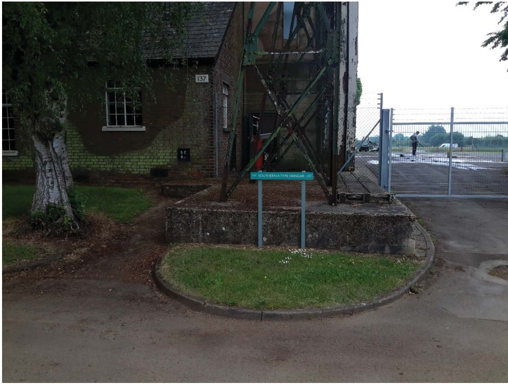
Plate 1 RAF Building No 137
