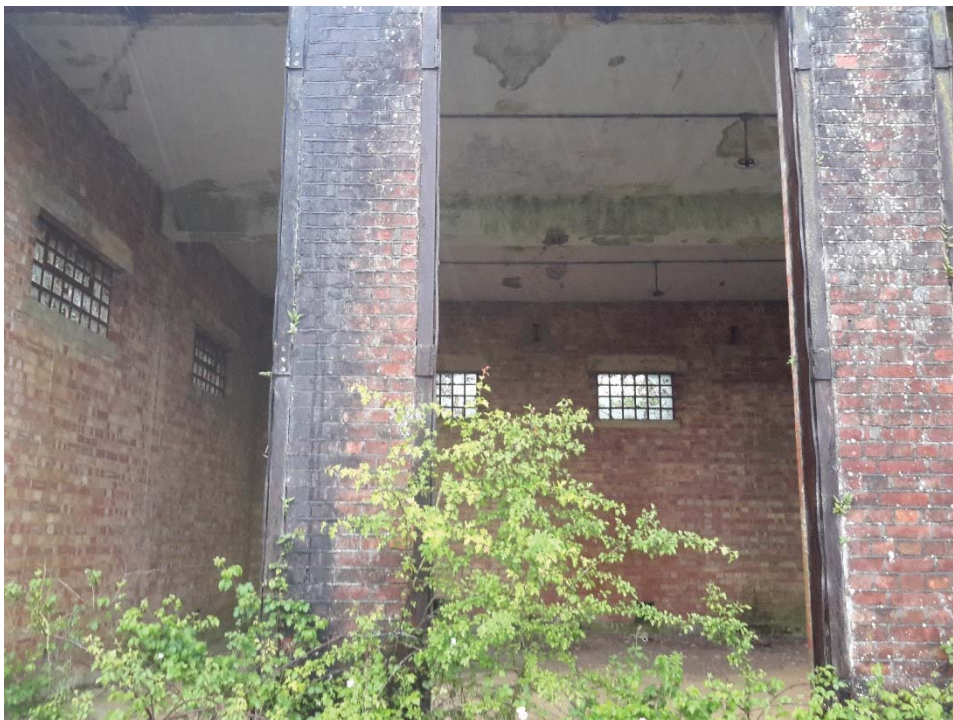
Plate 19 Building Within Former Ordnance Storage Area
