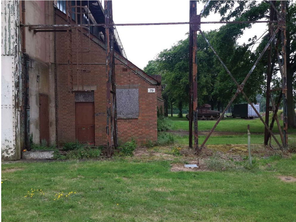
Plate 3 RAF Building No 79
