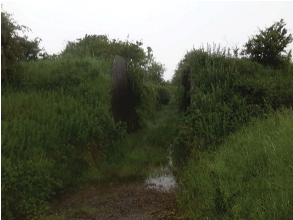
Plate 21 Blast Walls Within Former Ordnance Storage Area
