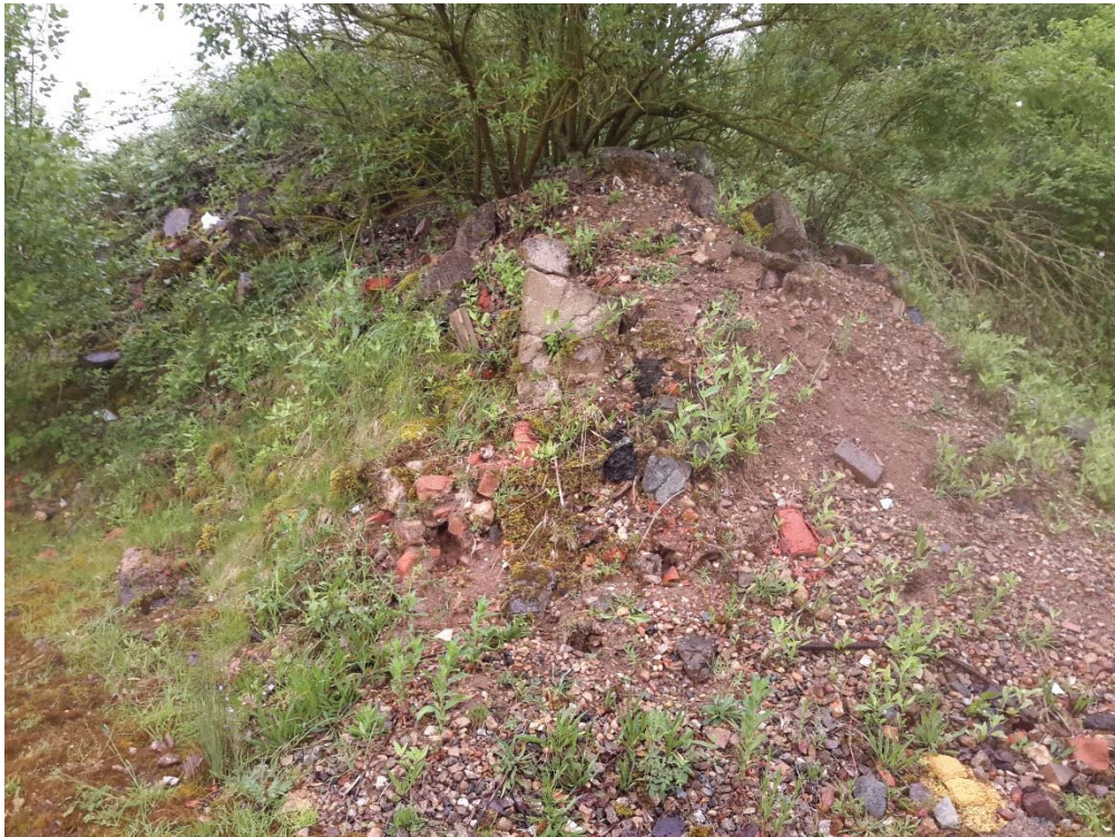
Plate 14 Waste Deposits in Former Quarry
