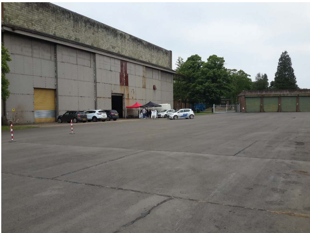
Plate 4 Concrete Hardstanding External to RAF Building
