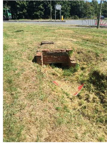
FIGURE 8: UPSTREAM CHANNEL AND CULVERT HEADWALL
