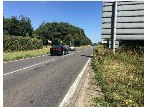
FIGURE 2: WESTERN BOUNDARY OF THE SITE
