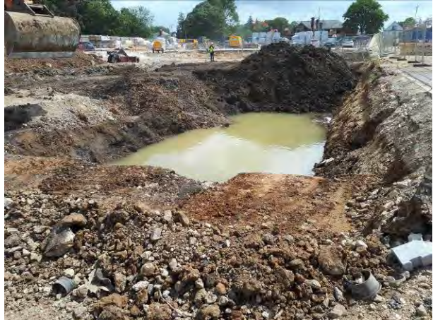
14.06.18 – Pooled water within excavation following inflow from western wall.
