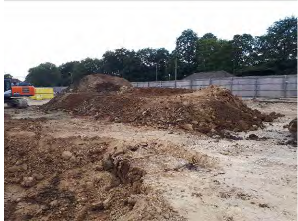
12.06.18 – Stockpile of recovered soils retained for replacement after contamination removal.
