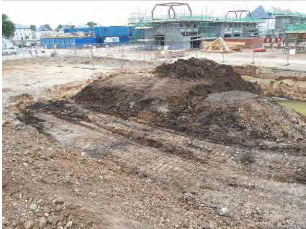
14.06.18 – Temporary stockpiling of hydrocarbon impacted materials within excavation.
