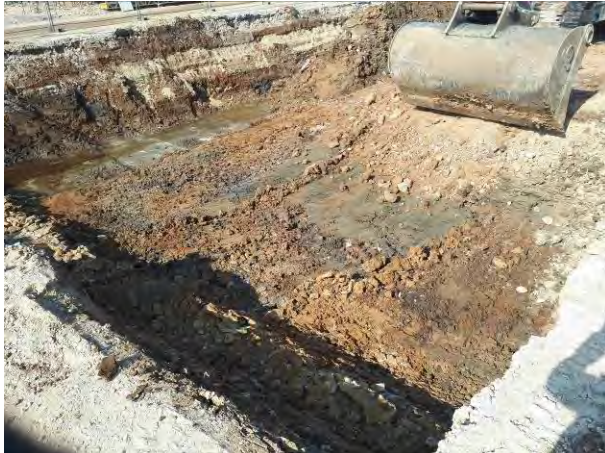
13.06.18 – Continuation of soil strip of materials not demonstrating contamination indicators.
