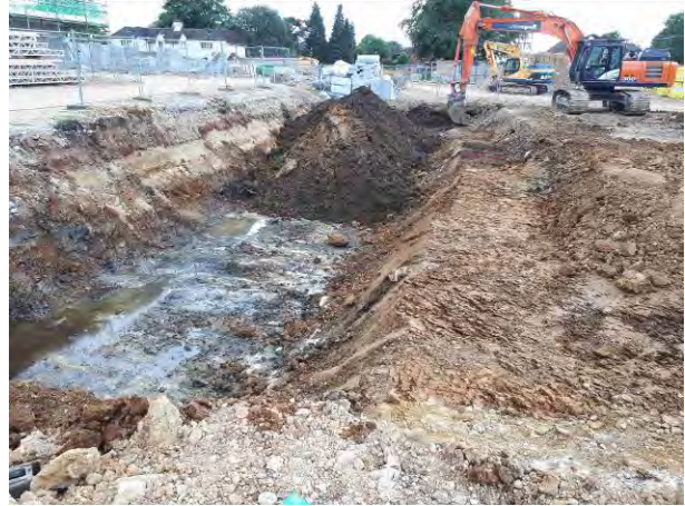
12.06.18 – Hydrocarbon contaminated soils temporarily stockpiled within excavation pending removal offsite; residual staining present on lower reaches of southern sidewall.
