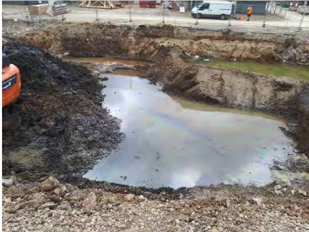
20.06.18 – Iridescent sheen observed on pooled water within excavation.
