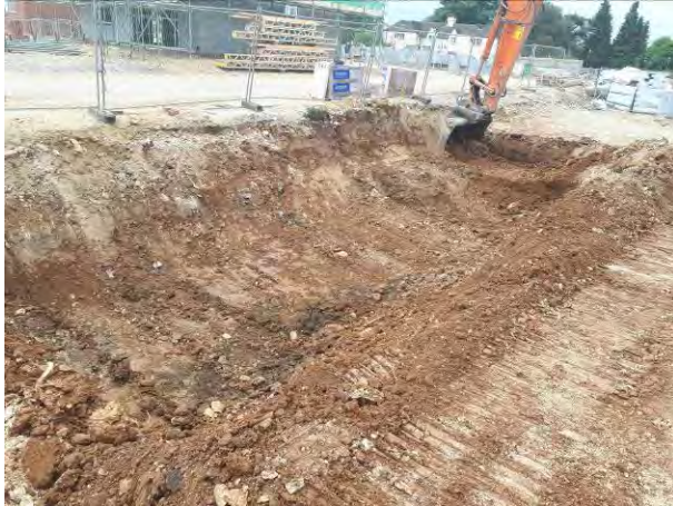
12.06.18 – Initial strip of surface soils not demonstrating contamination indicators along southern extent of excavation.
