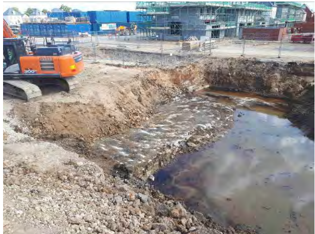
20.06.18 – View of eastern extent of excavation following removal of hydrocarbon contaminated soils.
