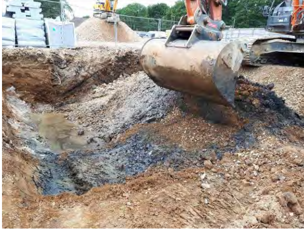
12.06.18 – Excavation of hydrocarbon contaminated soils along southern extent down to weathered bedrock.
