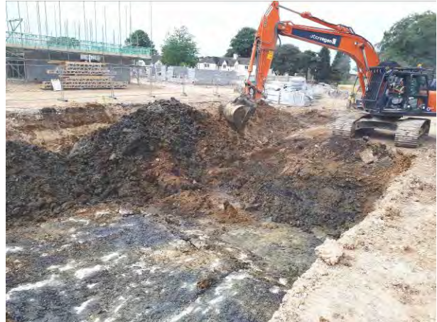
13.06.18 – Continued excavation of hydrocarbon contaminated soils down to weathered bedrock.
