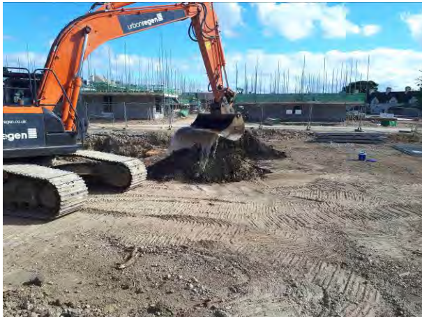
20.06.18 – Soils excavated from area above ACM sheeting dampened down using pooled water.
