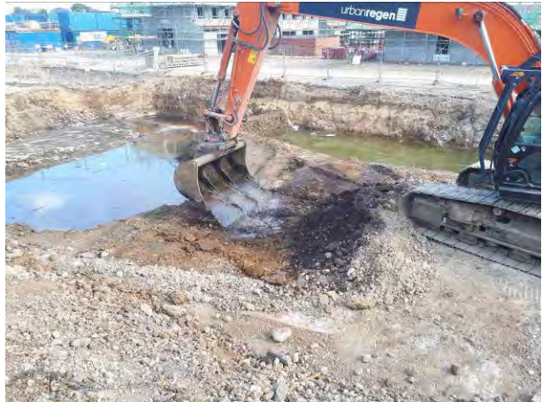
20.06.18 – Pooled water used to dampen down discovered ACM cement sheeting to reduce potential for fibre dispersal.
