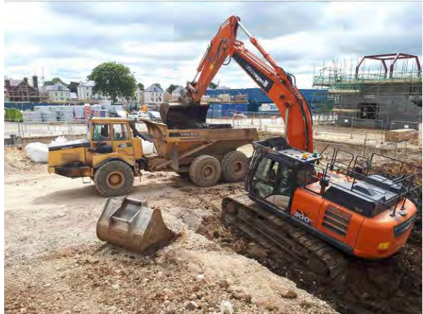
20.06.18 – Removal of hydrocarbon impacted soils to quarantine area within wider NSA area.
