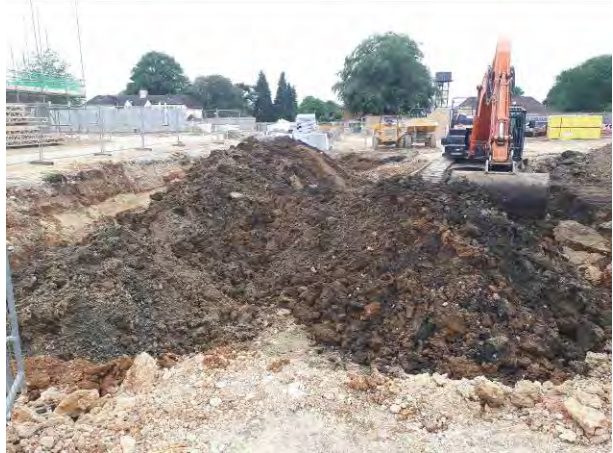
13.06.18 – Temporary stockpiling of hydrocarbon impacted materials within excavation.
