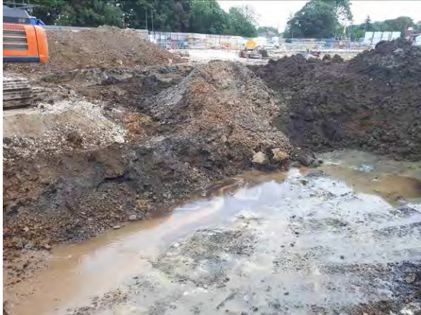
14.06.18 – Inflow of water into excavation from western wall; black product observed floating on surface.
