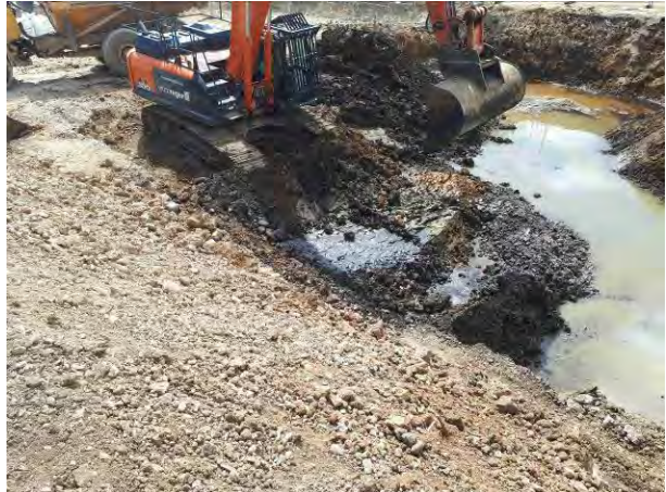
20.06.18 - Continued excavation of hydrocarbon contaminated soils down to weathered bedrock.
