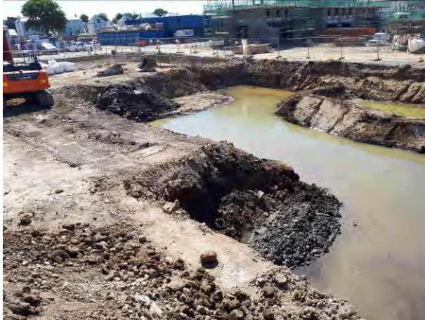
25.06.18 - View southeast across excavation area.
