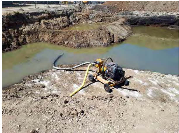
26.06.18 – Water pumped from excavation into adjacent USTs to east.
