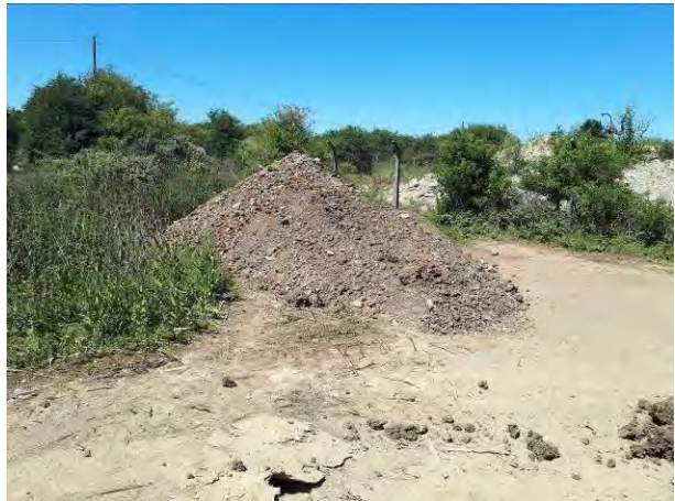
02.07.18 - Stockpile of hydrocarbon / asbestos contaminated soils in quarantine area; material excavated from area of the hotspot surrounding the deposits of ACM cement sheeting.
