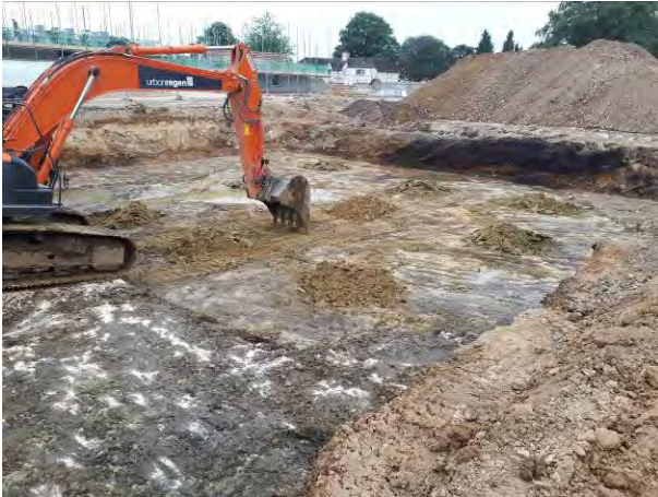
27.06.18 – Weathered bedrock at base of excavation disturbed for sample collection.
