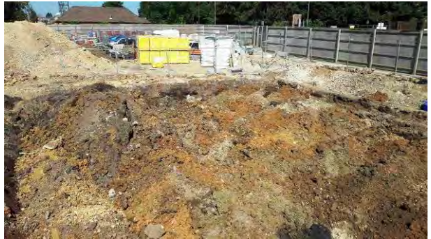
29.06.18 - Retained soils in northwest of excavation.
