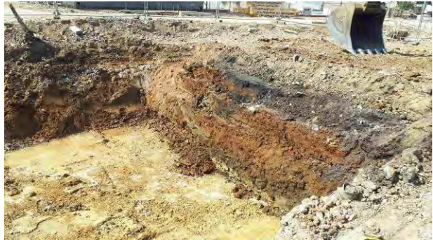
28.06.18 – View of southern end of western sidewall; no significant contamination indicators observed.
