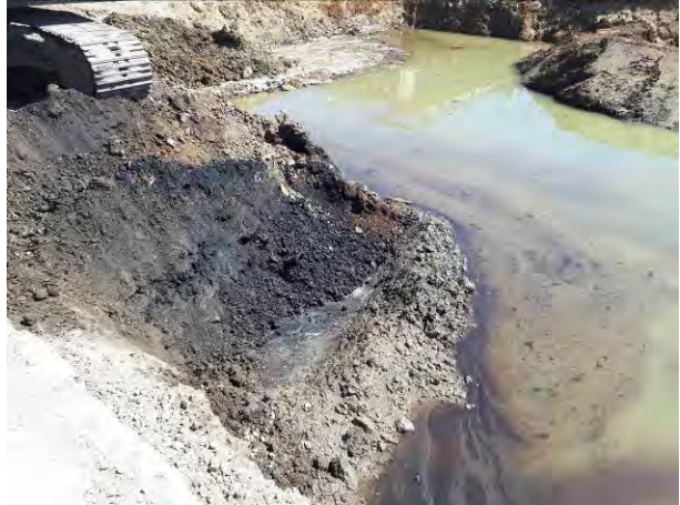
25.06.18 - Continued excavation of hydrocarbon contaminated soils down to weathered bedrock.
