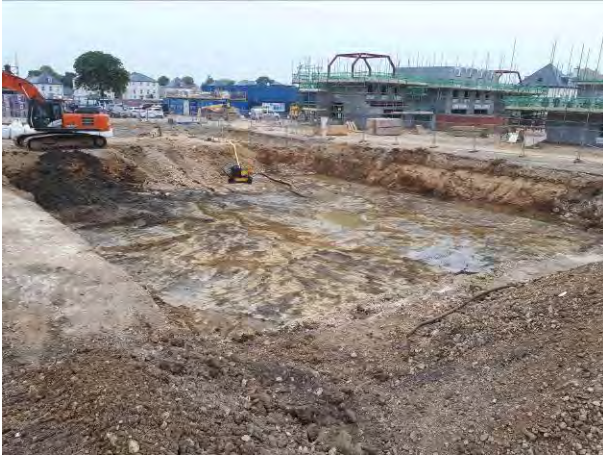
27.06.18 – Pooled water pumped from excavation area exposing weathered bedrock.
