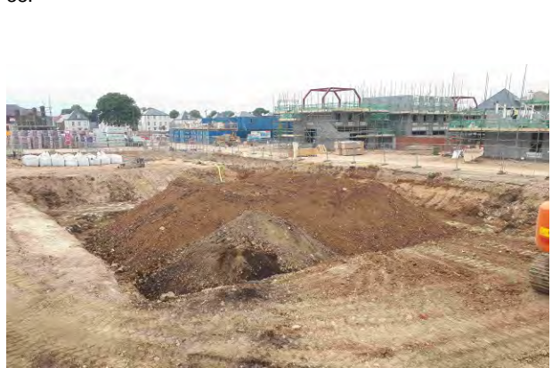
28.06.18 – Retained soils stockpiled within excavation.
