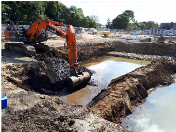
22.06.18 - Continued excavation of hydrocarbon contaminated soils down to weathered bedrock.
