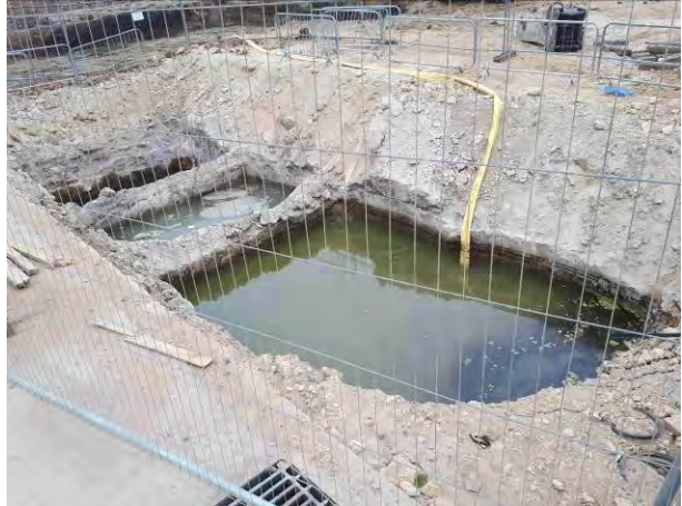
27.06.18 – Water pumped from excavation contained within adjacent USTs to east.
