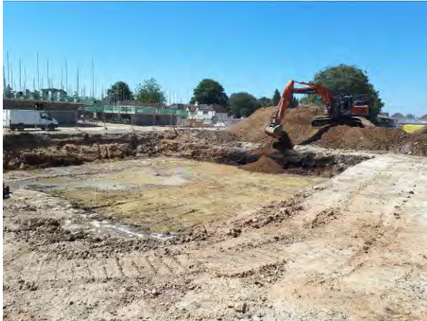
27.06.18 – Replacement of retained soils into excavation.
