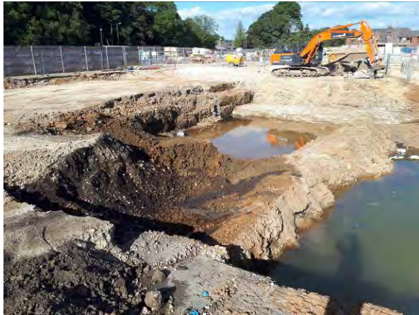
21.06.18 – View east across excavation area.
