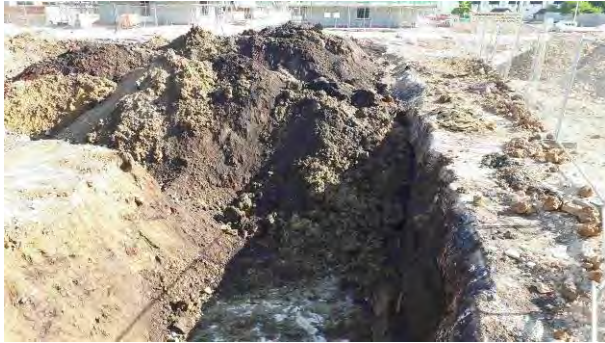
28.06.18 – View along southern extent of excavation.
