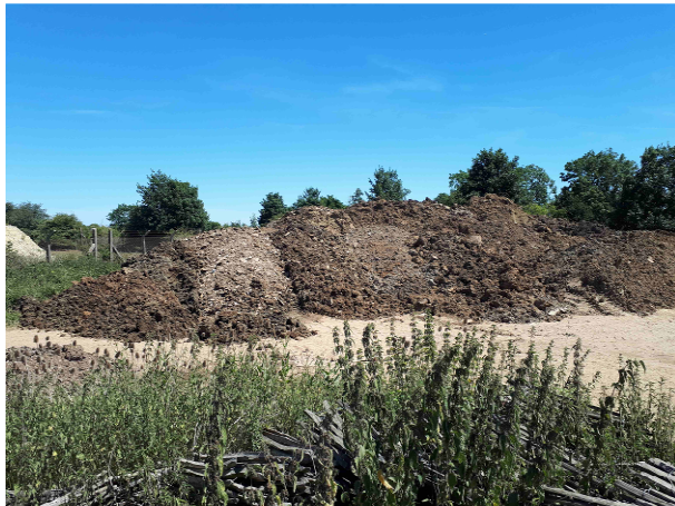
02.07.18 – Stockpile of hydrocarbon contaminated soils in quarantine area.
