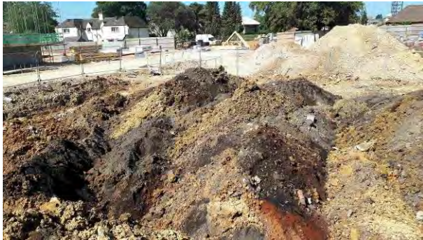
29.06.18 – Retained soils in southwest of excavation.
