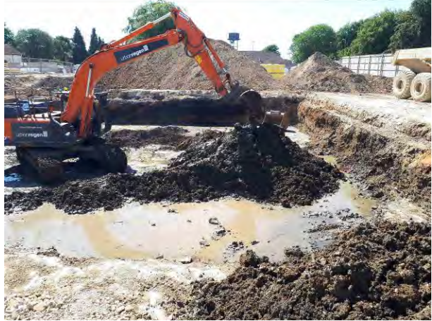
26.06.18 - Continued excavation of hydrocarbon contaminated soils down to weathered bedrock.
