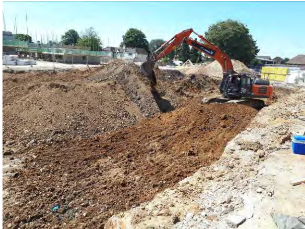
02.07.18 – Replacement and recompaction of retained soils within excavation.
