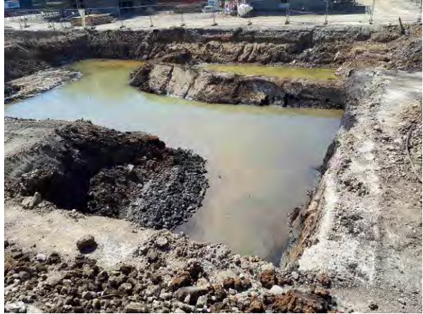
25.06.18 - View south across excavation area.
