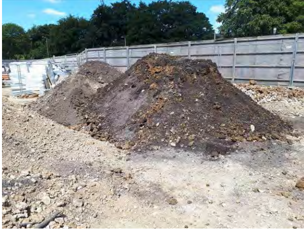
22.06.18 – Additional stockpile of recovered soils retained for replacement after contamination removal.
