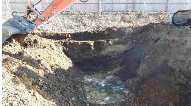
29.06.18– Continuation of excavation down to natural bedrock along western end of northern extent; no significant contamination indicators observed - soils sampled and retained.
