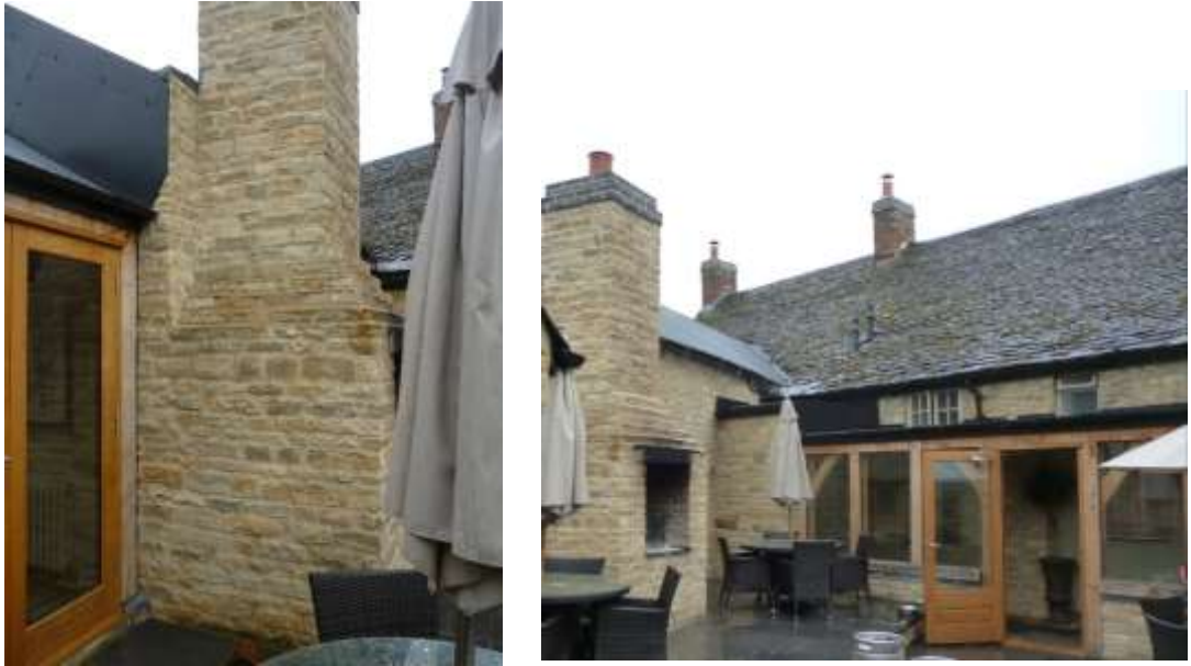
Side view of chimney & chimney in context.
