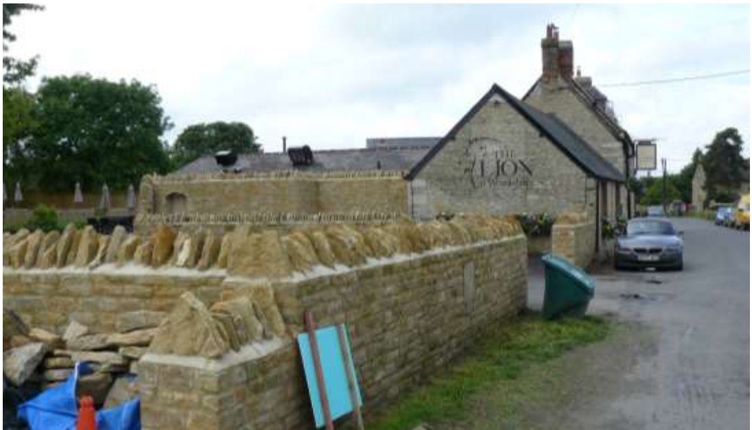
View looking South along Wendlebury Road. Chimney barely noticeable.
