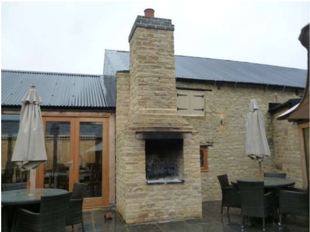
Above: Front view of external fire & chimney.
