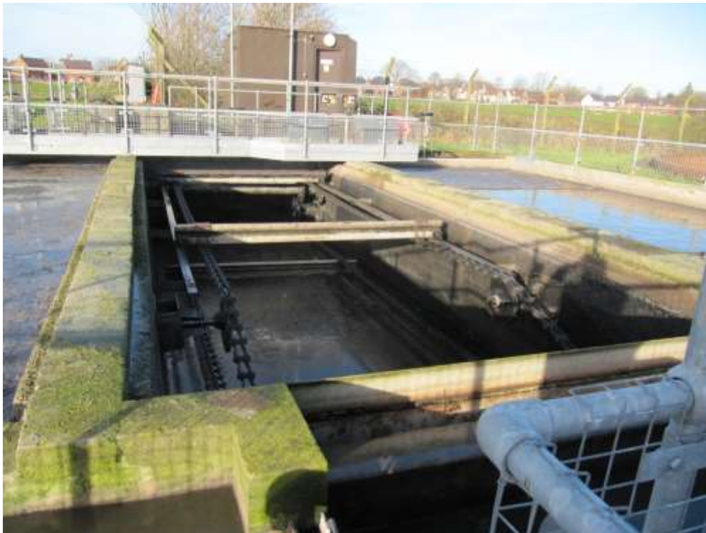
Fig. 2. Primary sedimentation tanks during emptying
