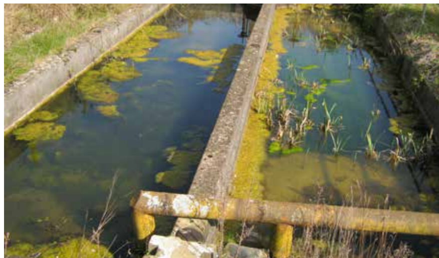
Typical on site waterbody - manmade storage tanks
