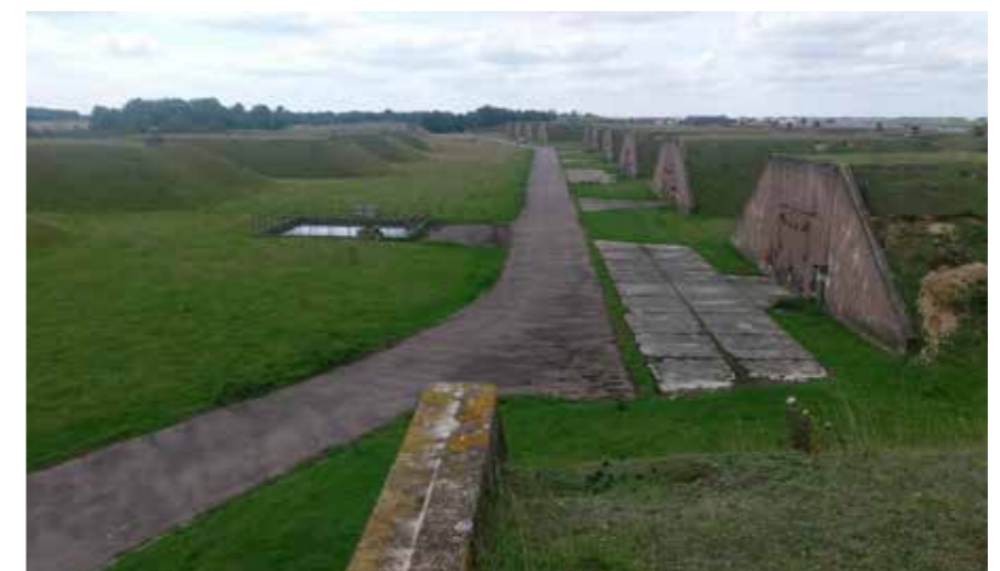
Unimproved and semi-improved calcareous grassland in the Southern Bomb Stores (the light brown areas are unimproved calcareous)
