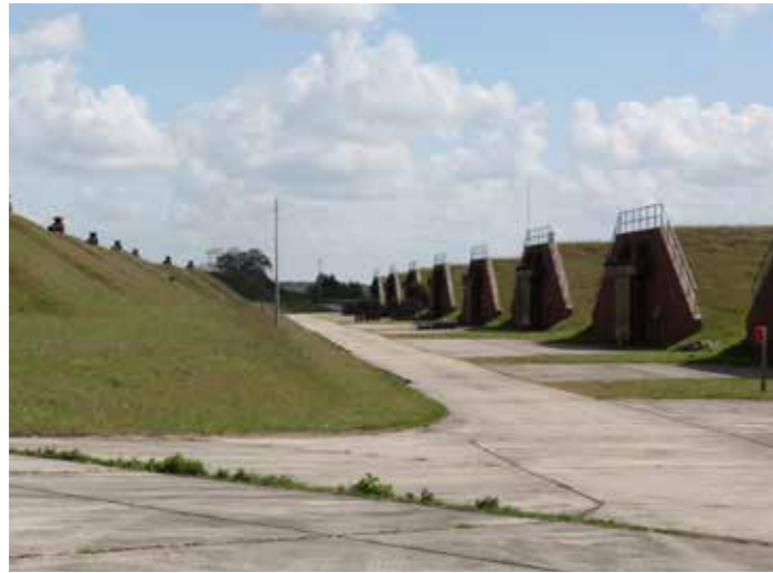
Photograph 3 - Southern Bomb Stores
