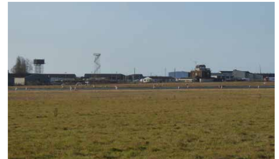
View across the runway towards the Control Tower and Water Tower
