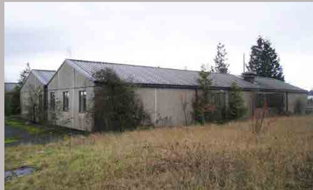
EXISTING BUILDING 370 TO BE RETAINED AND CONVERTED INTO OFFICES
