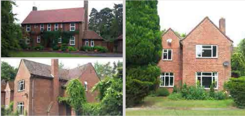
EXISTING FORMER OFFICERS HOUSING LOCATED OPPOSITE THIS ZONE
