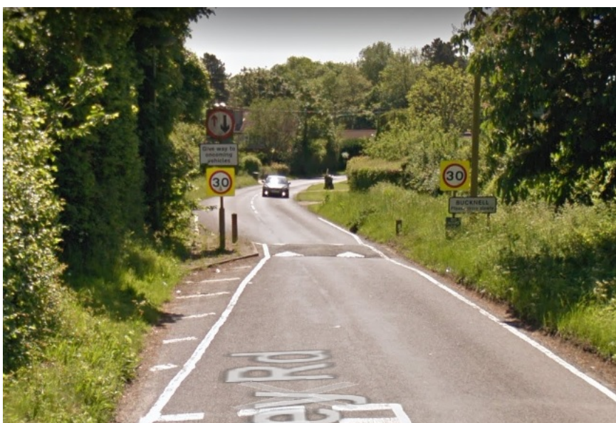
Image 1. Example of Village entrance speed restriction at Bucknell.
