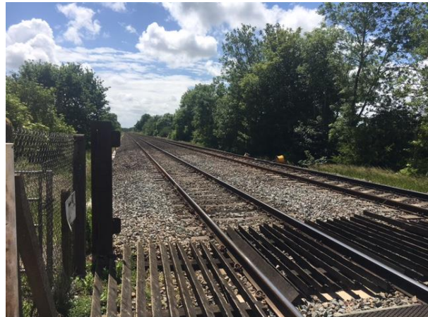
Up side towards down train approach
