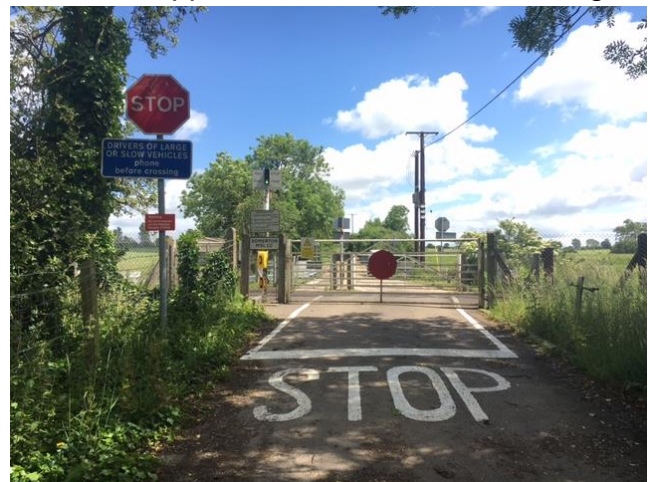
Down side approach of Somerton Crossing
