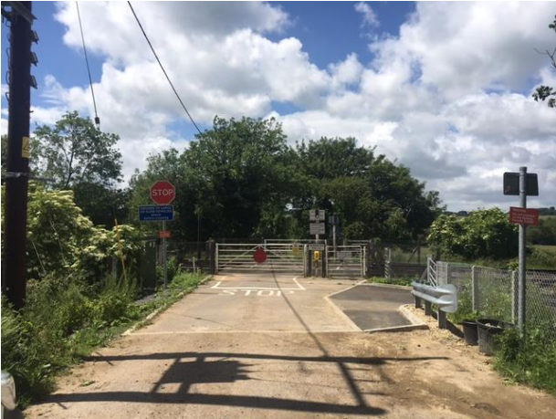
Up side Crossing approach
