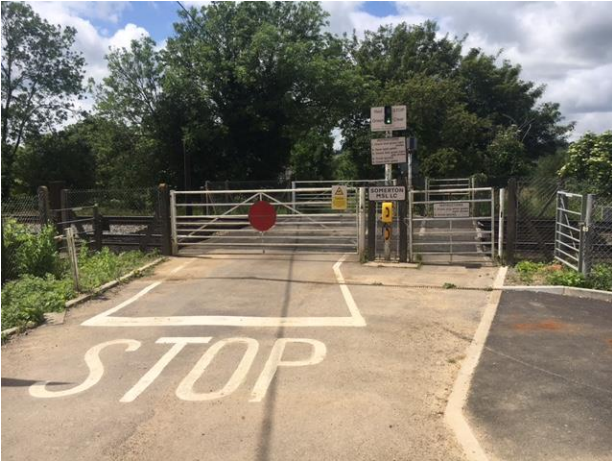
Up side crossing approach
