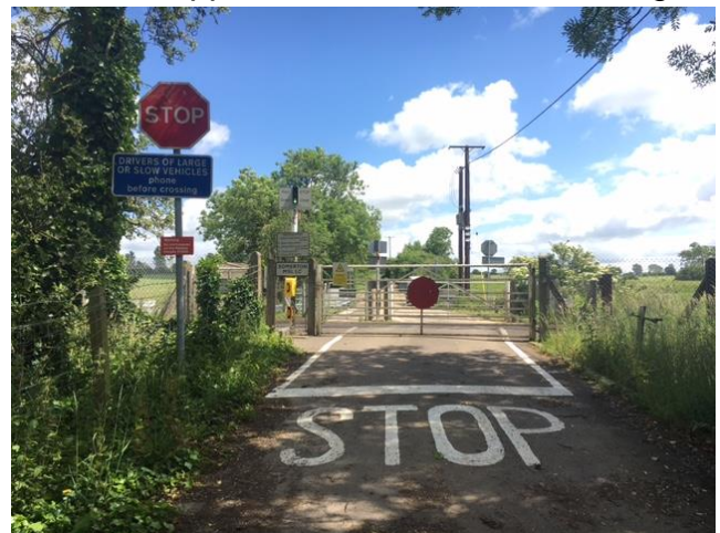
Down side approach of Somerton Crossing
