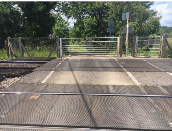
Up side across crossing
