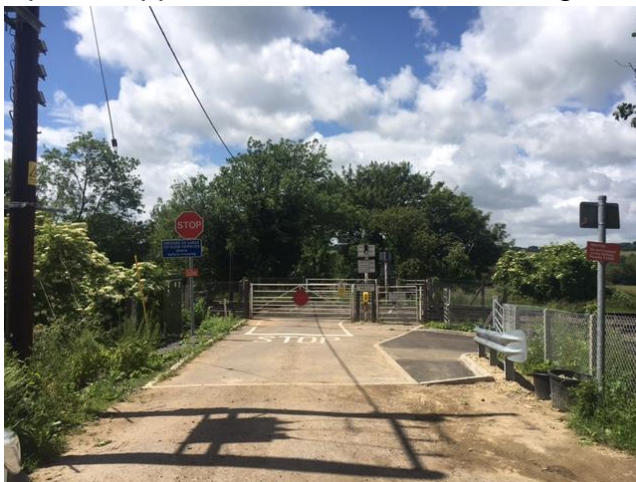
Up side approach of Somerton Crossing
