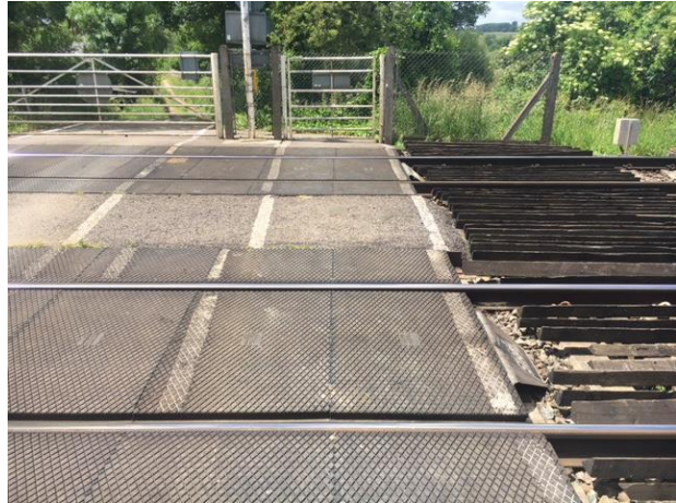
Up side across crossing
