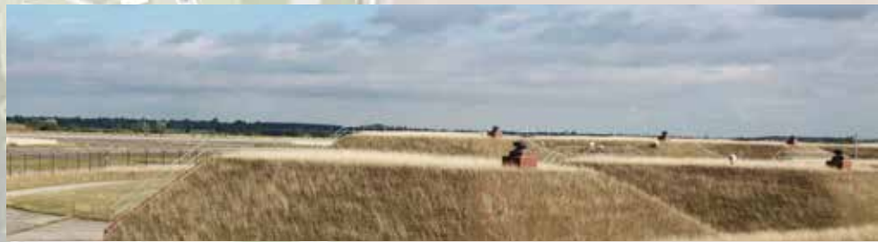
EXISTING SOUTHERN BOMB STORE LOCATED ADJACENT TO ZONE
