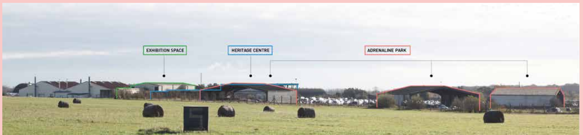
LOOKING SOUTH TOWARDS THE PROPOSED VISITOR DESTINATION AREA FROM THE FLYING FIELD
