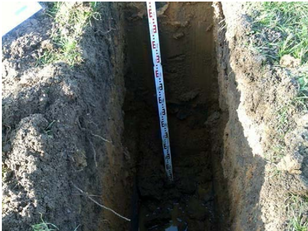
Trial pit 09 south face
