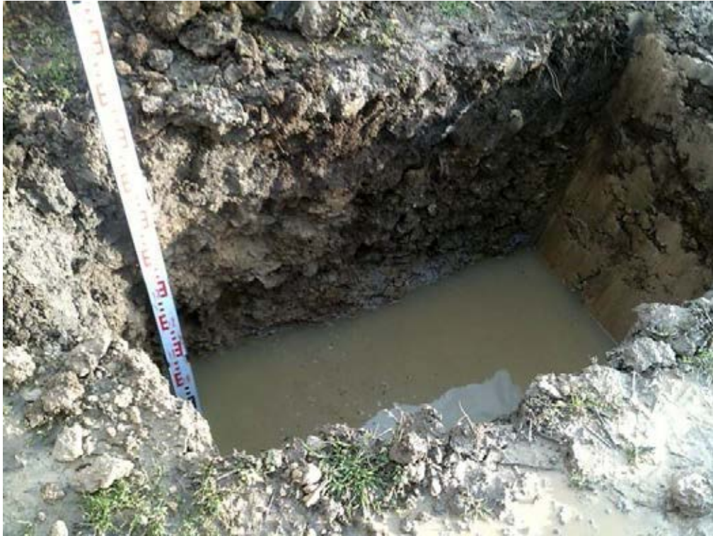
Trial pit 06 north face
