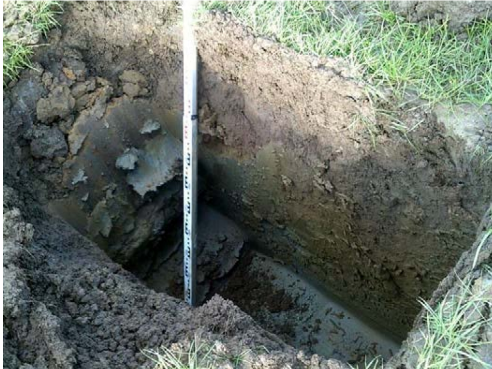
Trial pit 08 north face
