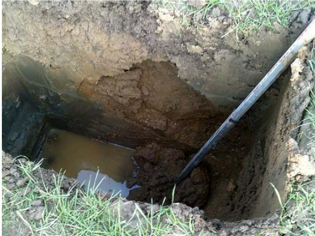
Trial pit 07 north face
