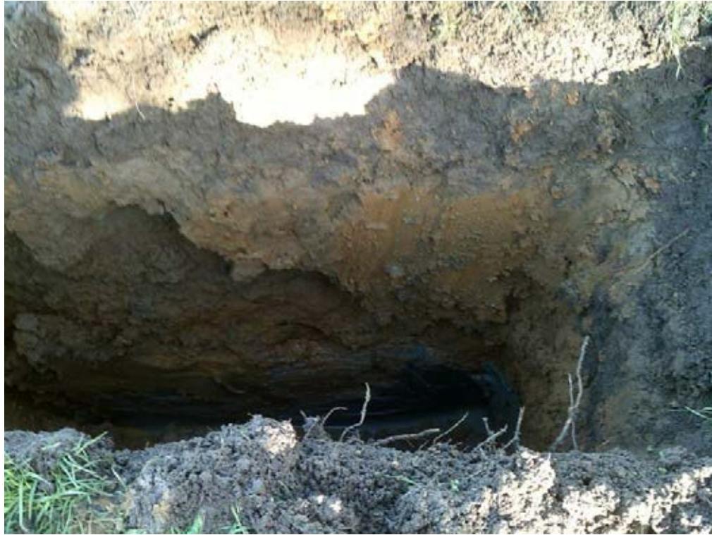
Trial pit 09 west face
