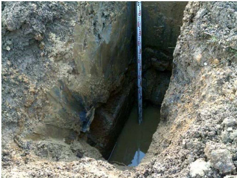
Trial pit 11 south face
