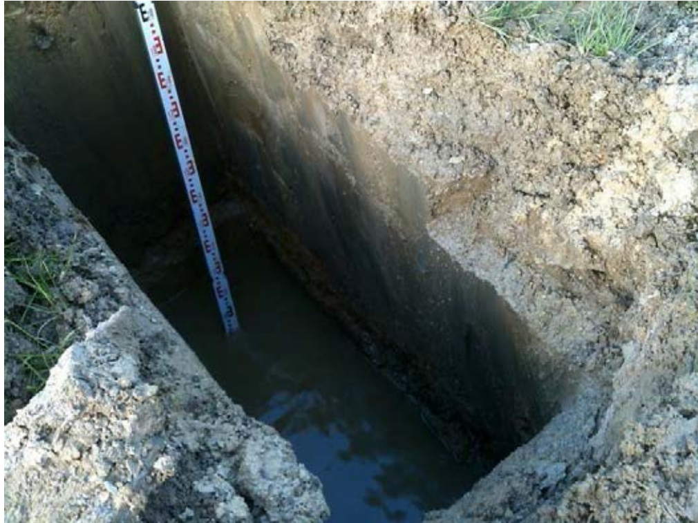
Trial pit 10 east face
