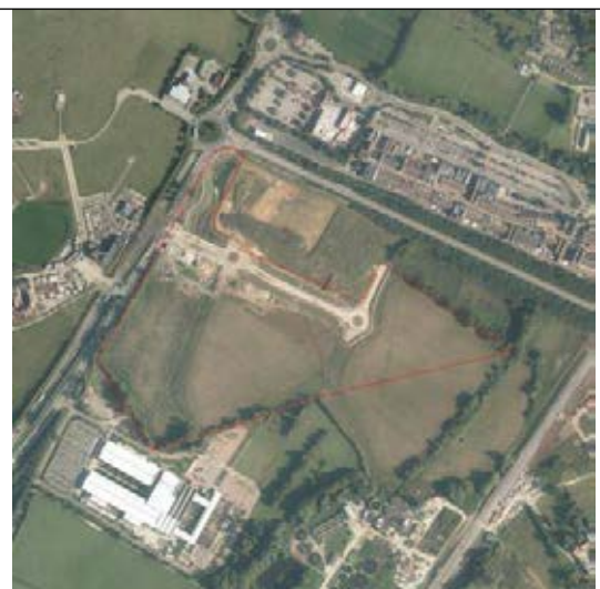
Figure 1-2 Aerial photograph of the site showing study area red line (September 2015)
