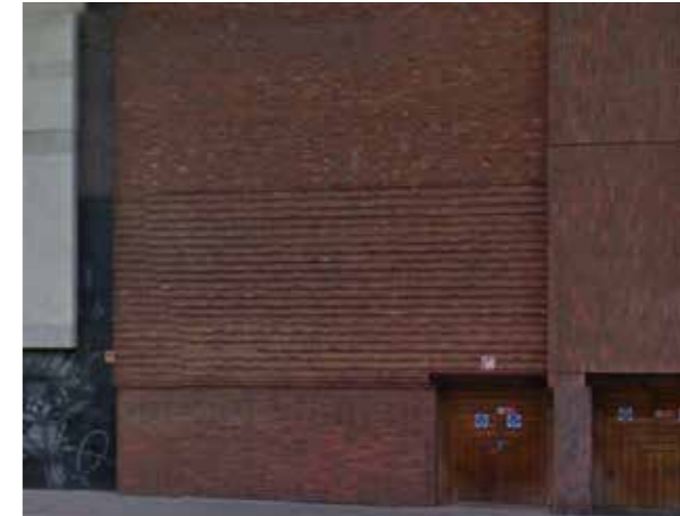
A6 BRICK BANDING COURSES ADDS A RICHNESS OF DETAIL TO THE MAIN FACADES.
