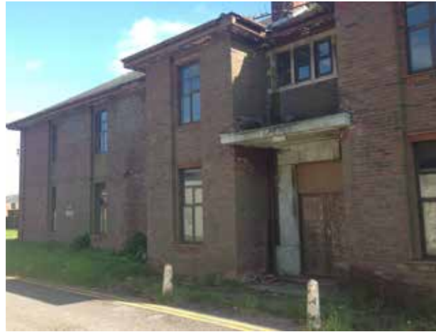
A3 CONTEMPORARY FLAT DOOR CANOPIES ARE INSPIRED BY TRADITIONAL ENTRANCE FEATURES FOUND THROUGHOUT HEYFORD PARK.
