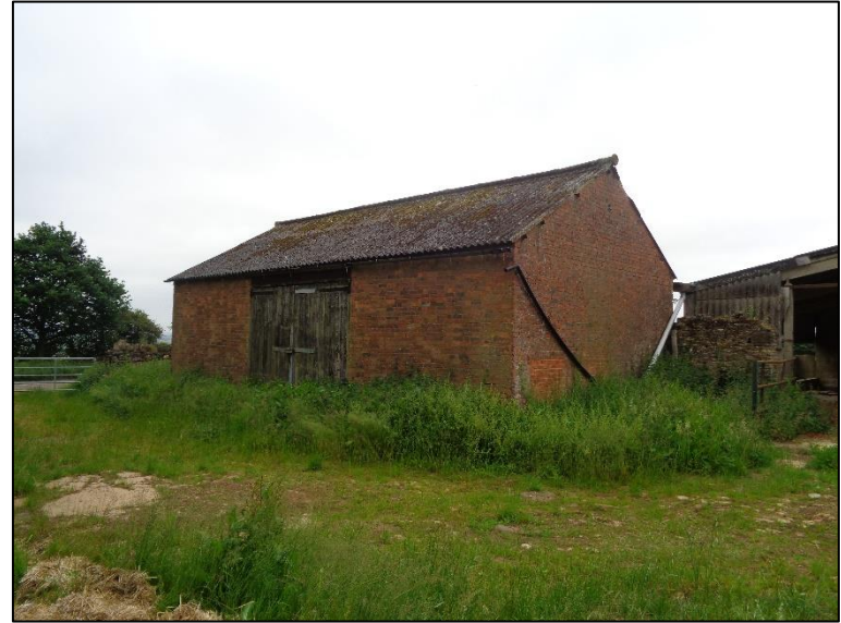
Building 2 as viewed from yard
