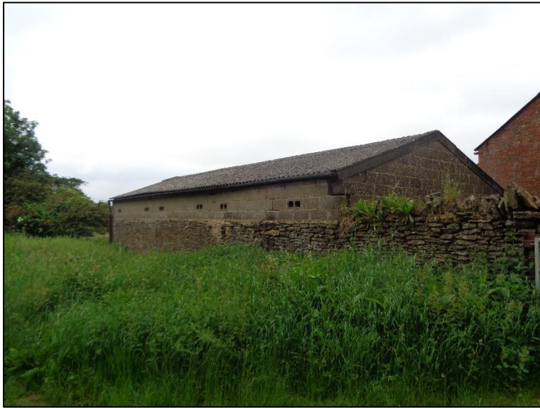
Building 1 as viewed from B4035
