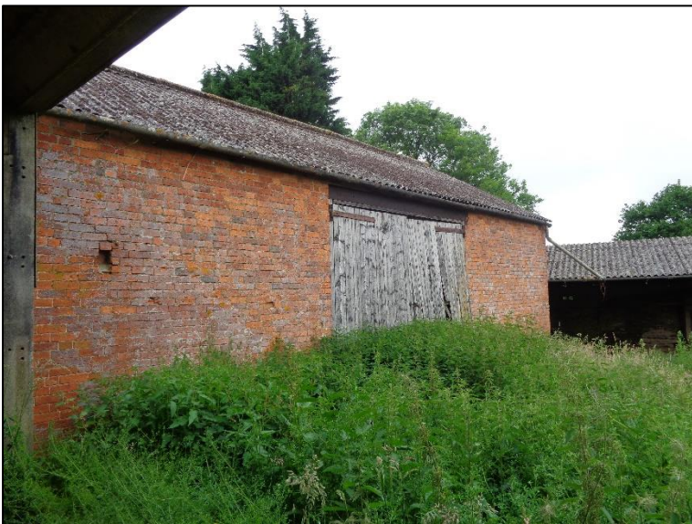
Building 2 as viewed from Building 3
