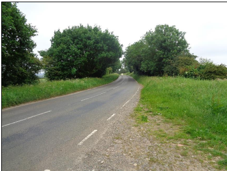
View from site entrance looking South-East along B4035
