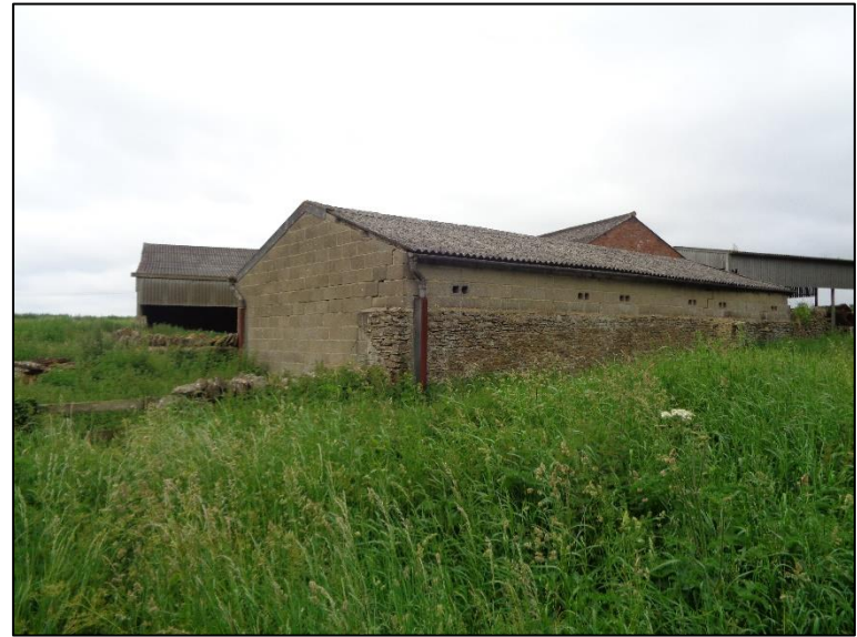
Building 1 as viewed from B4035
