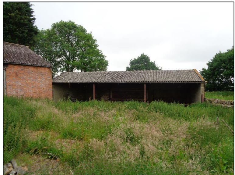
Building 1 as viewed from Building 3
