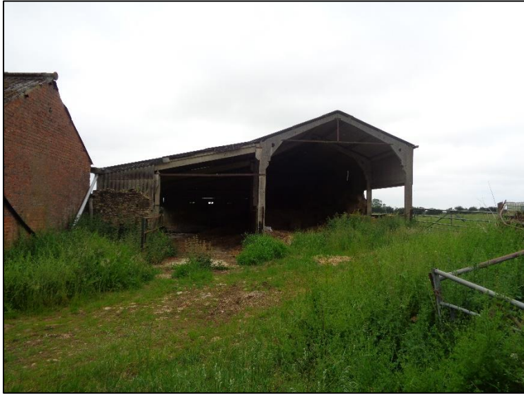
Building 3 as viewed from yard
