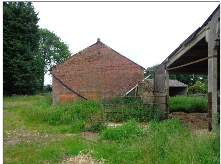
Building 2 as viewed from land adjacent to Building 3
