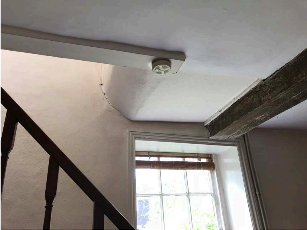
Make good to ceiling where staircase removed
