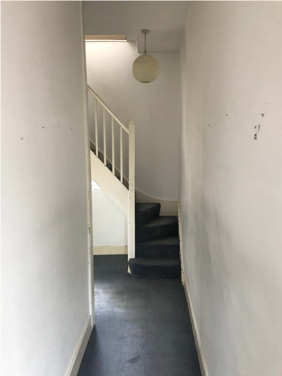
Staircase and partition beyond to be removed
