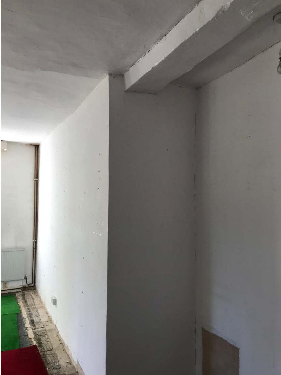
Block wall to be removed and create double fronted study
