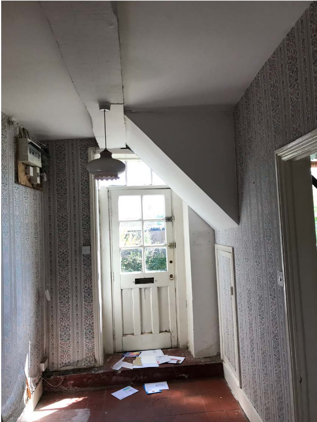
Remove stair soffit and under stairs cupboard
