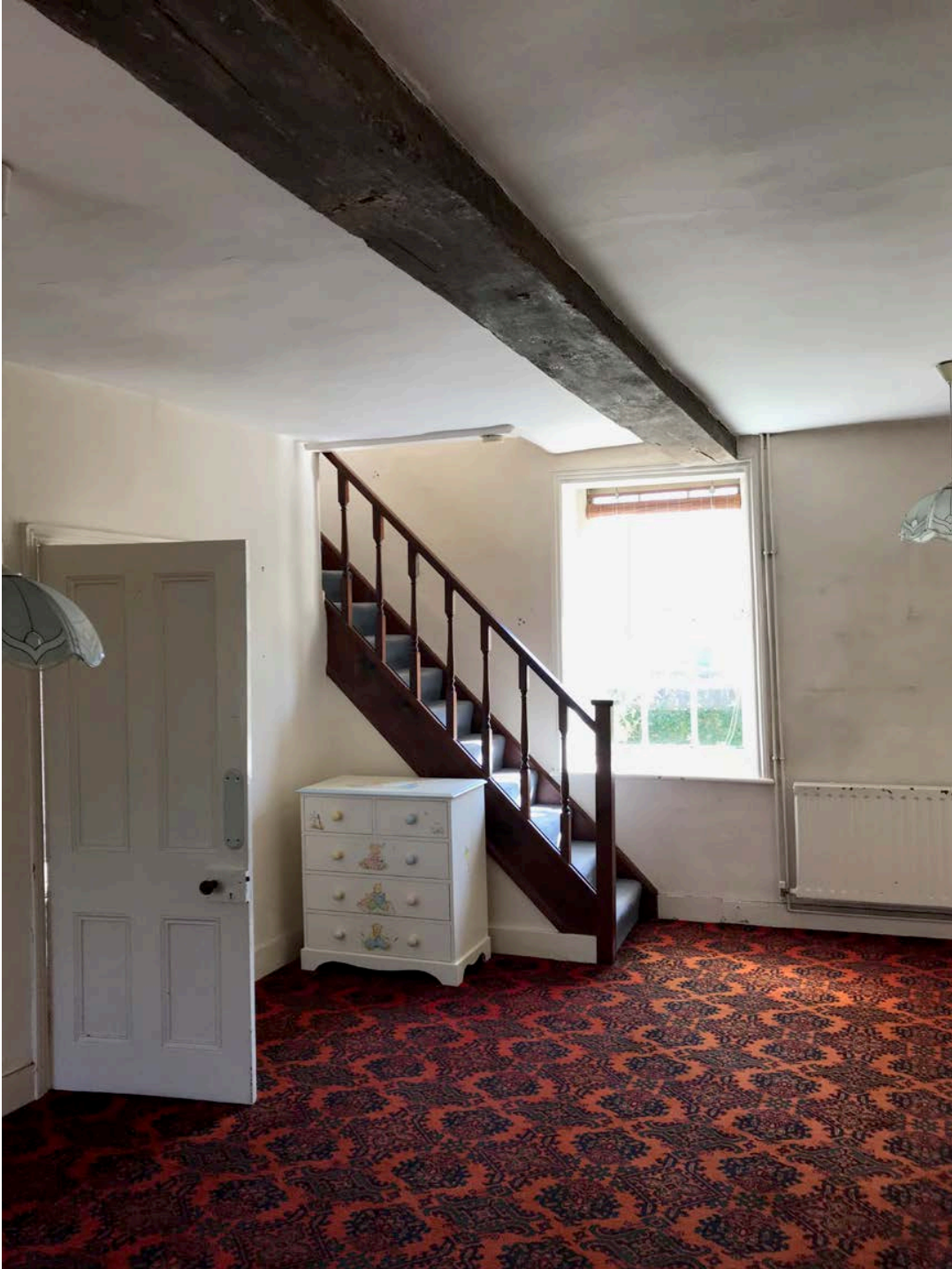
Staircase removed. Existing door relocated to new position.
