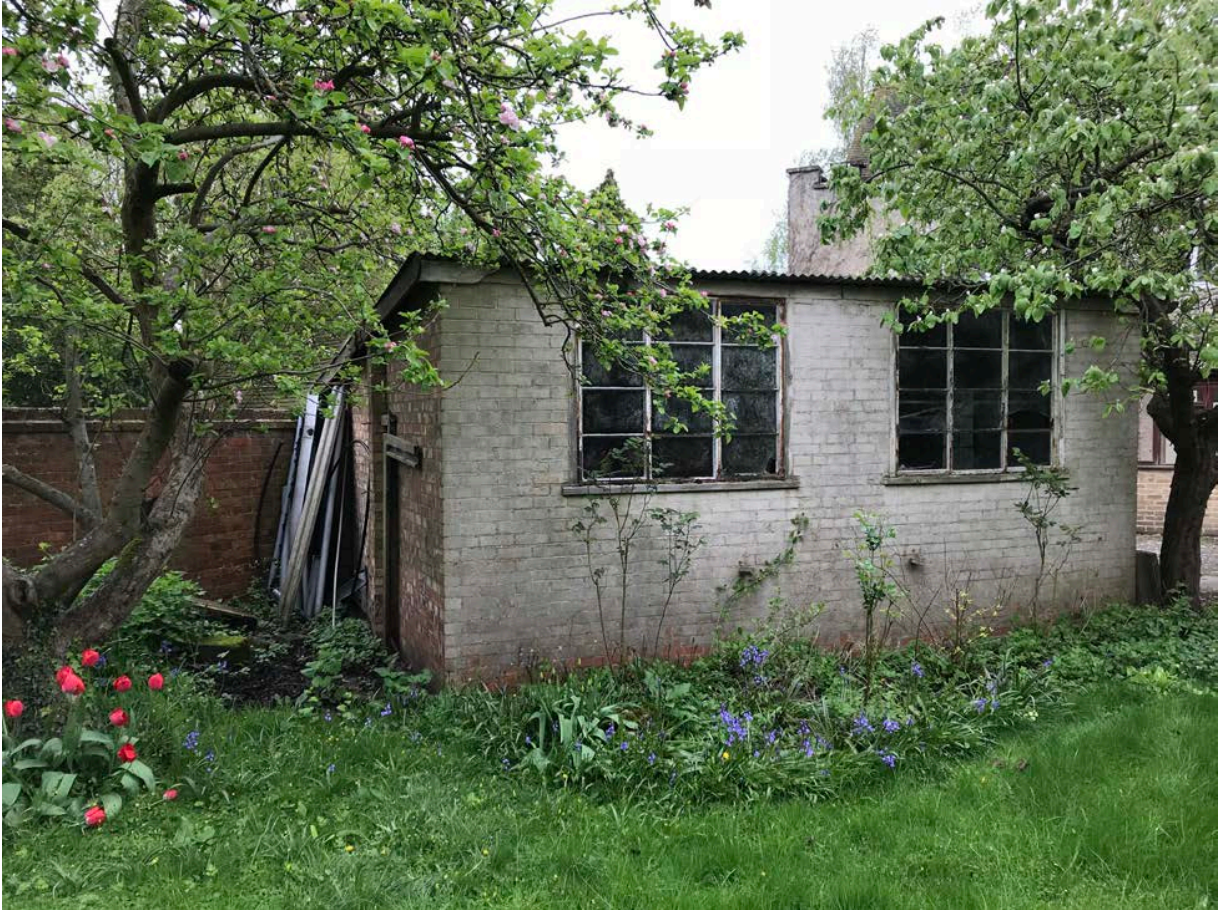
Brick garage to be removed
