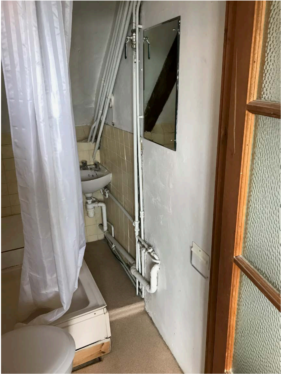
Shower room to be removed
