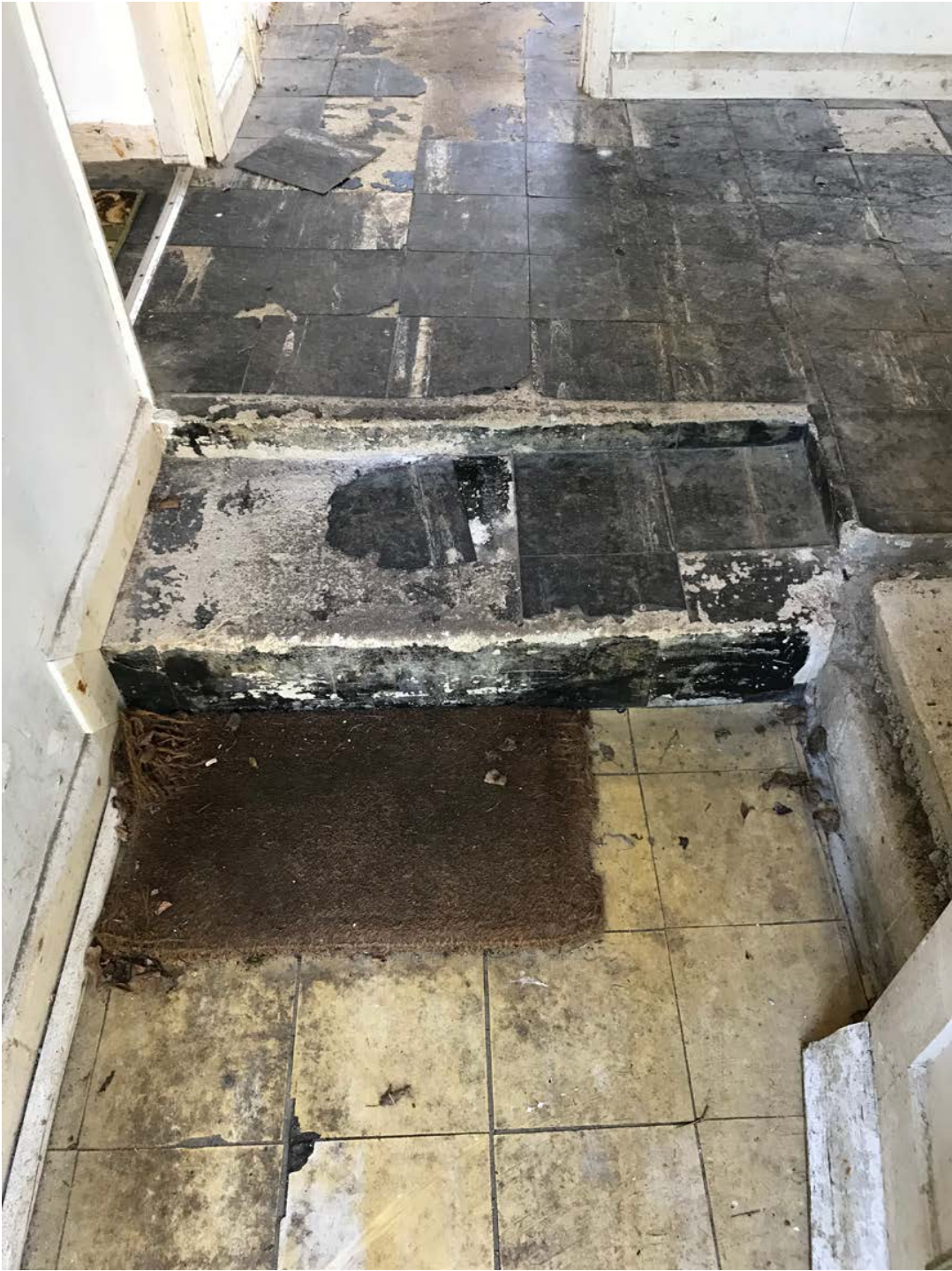
Remove existing floor finishes
