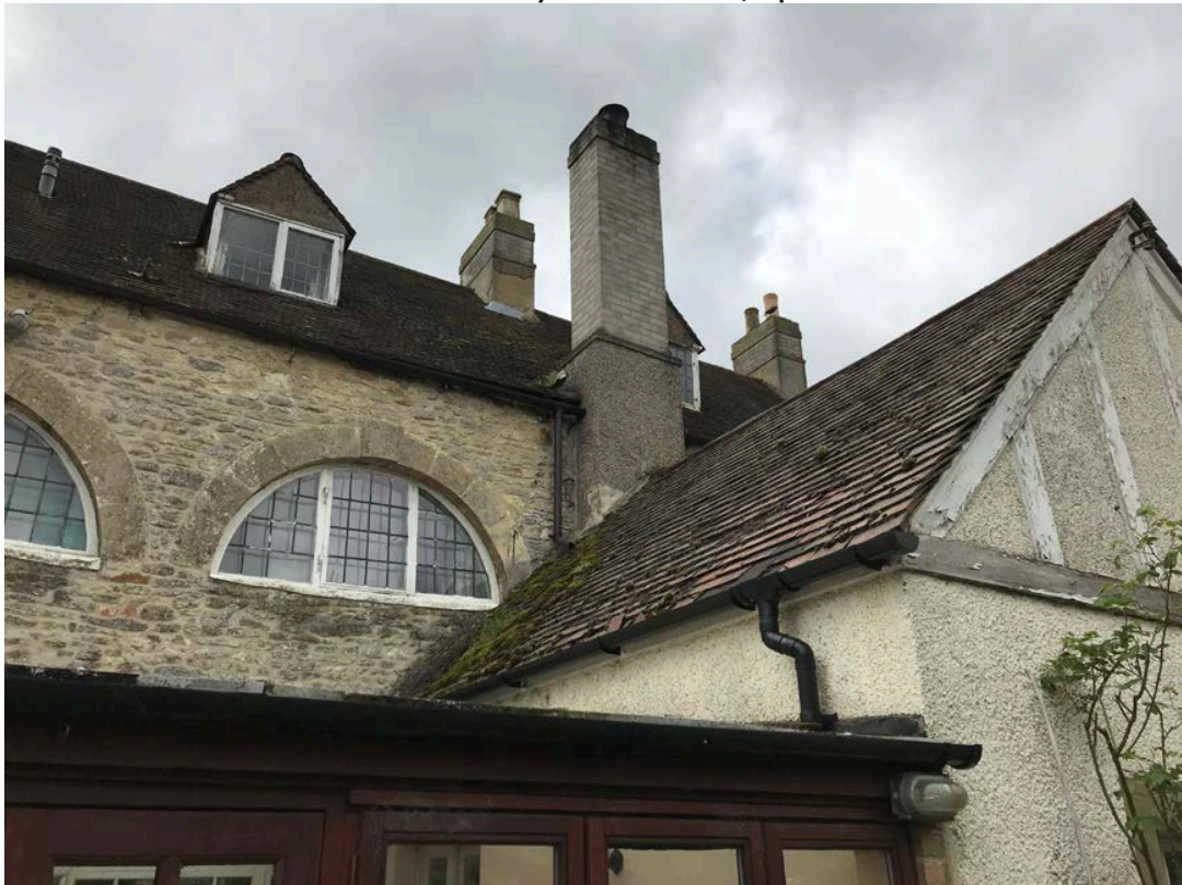
Later chimney stack to be removed
