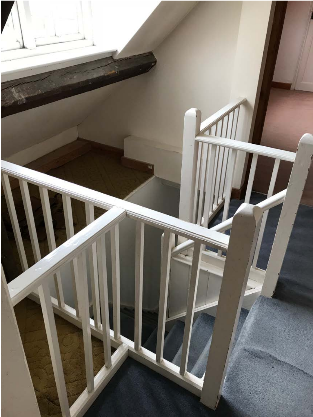
Staircase removed/replaced from first to second floor
