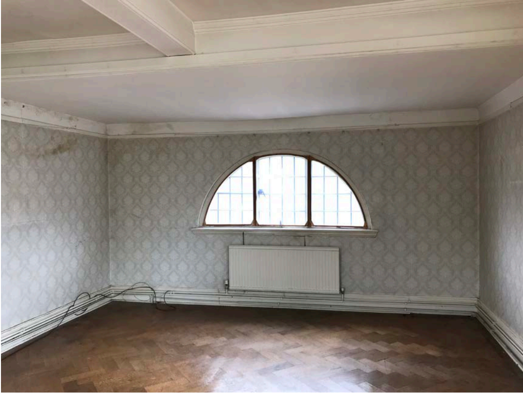
Area to be partitioned by new panelled wall to create wardrobe and ensuite facilities off master bedroom
