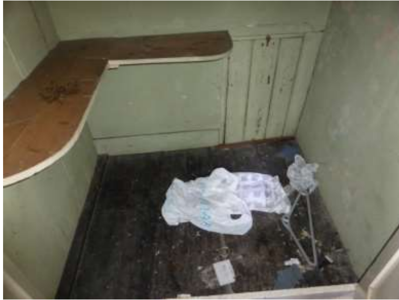
Figure 59: Narrow floorboards in A5
