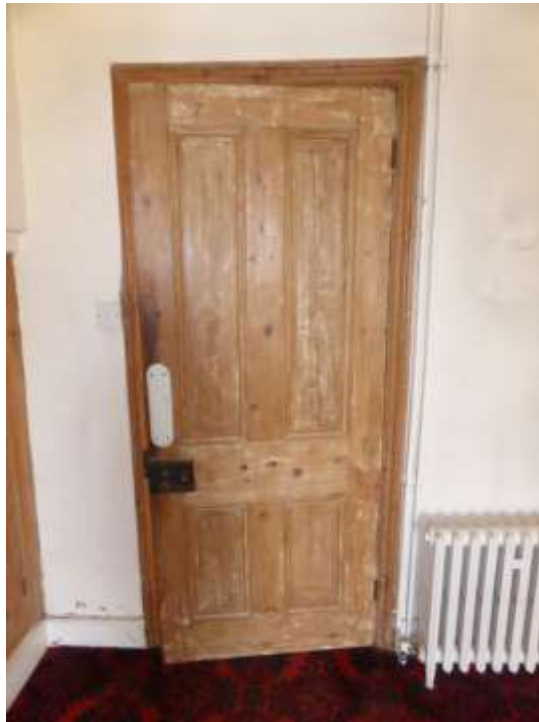
Figure 22: An early 20 th century door leading to the Kitchen (G10)
