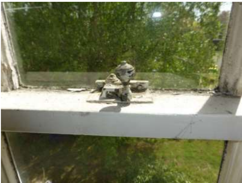
Figure 51: Later 19 th century type sash fasteners in F5
