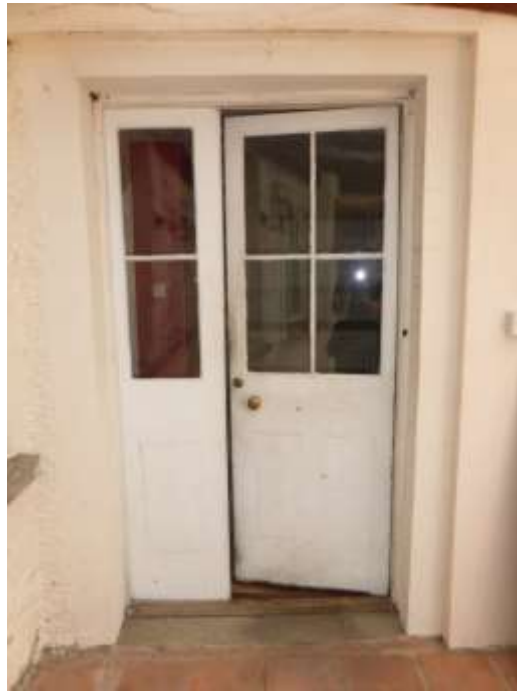
Figure 34: Door to the Kitchen (G10) from the Conservatory (G9)
