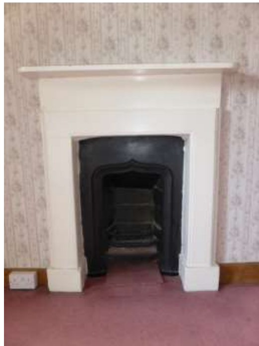
Figure 39: Later 19 th century coal grate in F1
