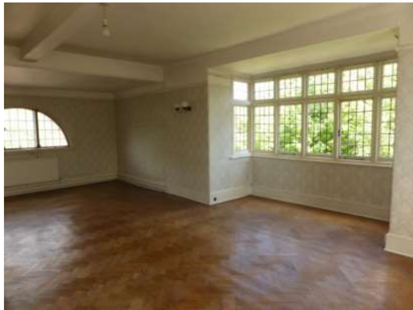
Figure 49: Re-set thermal window to the left and early 20 th century oriel to the right
