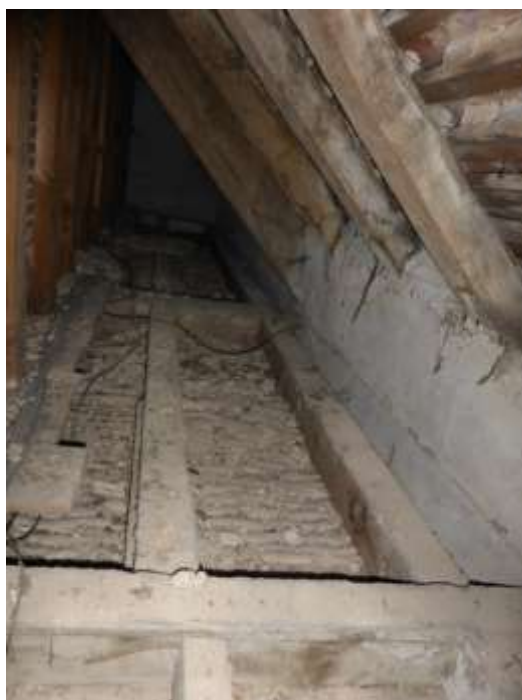
Figure 58: Structure of the ceiling over F5 and machine sawn timbers of an ashlar wall in A5
