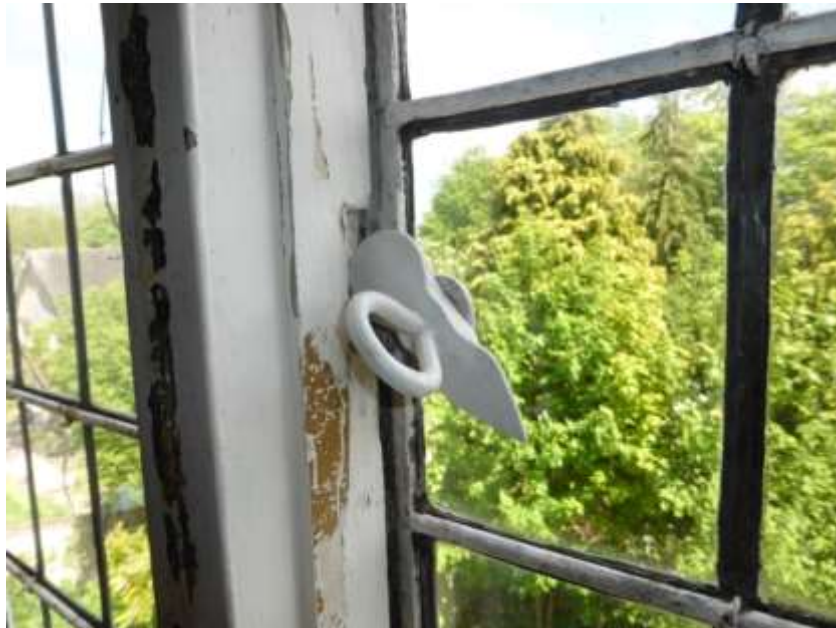
Figure 60: Early 20 th century window catch on the window in the eastern gable end
