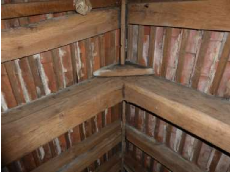
Figure 55: Apex of principal rafters at A1
