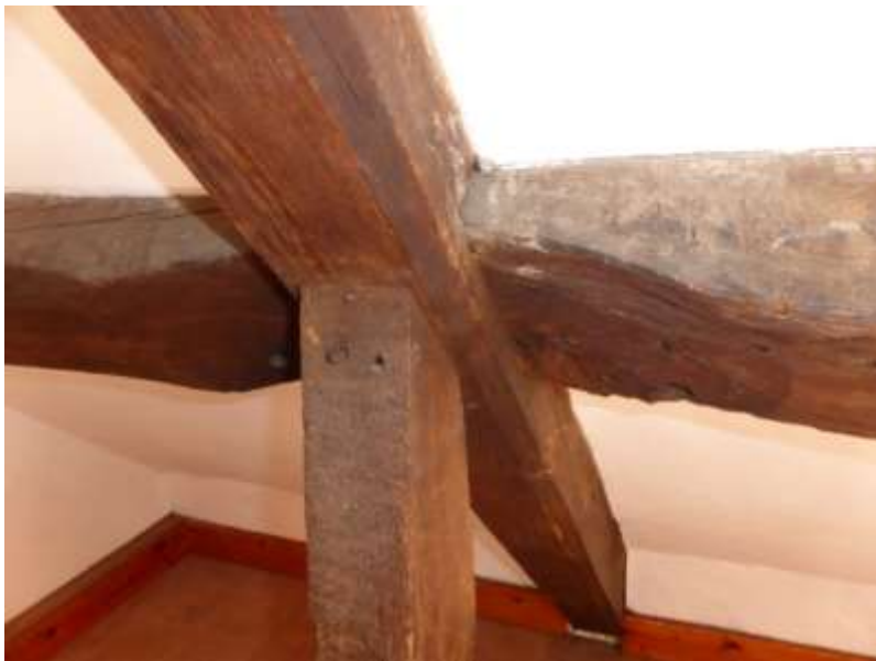
Figure 56: Tenoned purlin in A1
