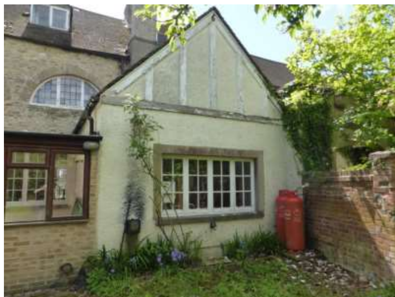
Figure 18: Early 20 th century single storey extension on the right hand side of the rear elevation
