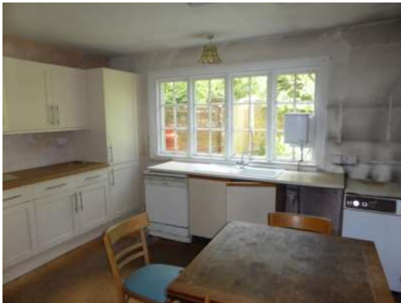
Figure 35: The Kitchen (G10) looking north
