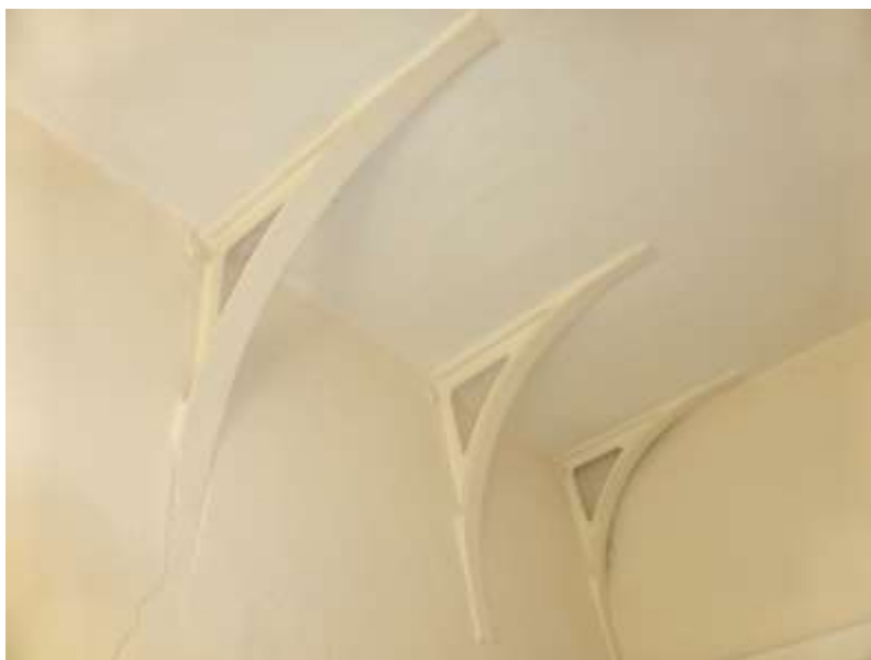
Figure 28: Brackets supporting a first floor hearth
