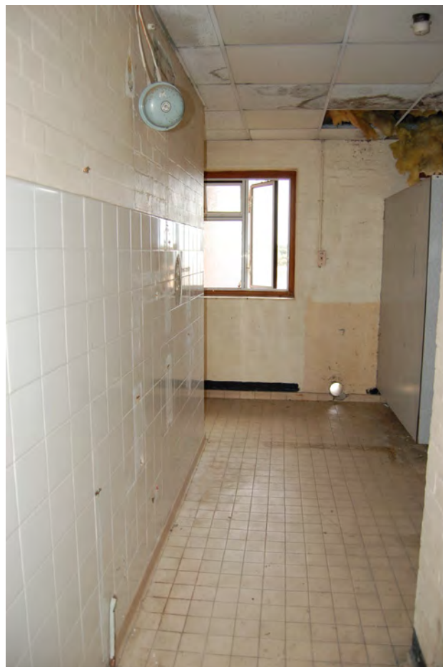
Plate 485.10 The range of finishes in the ablutions block
