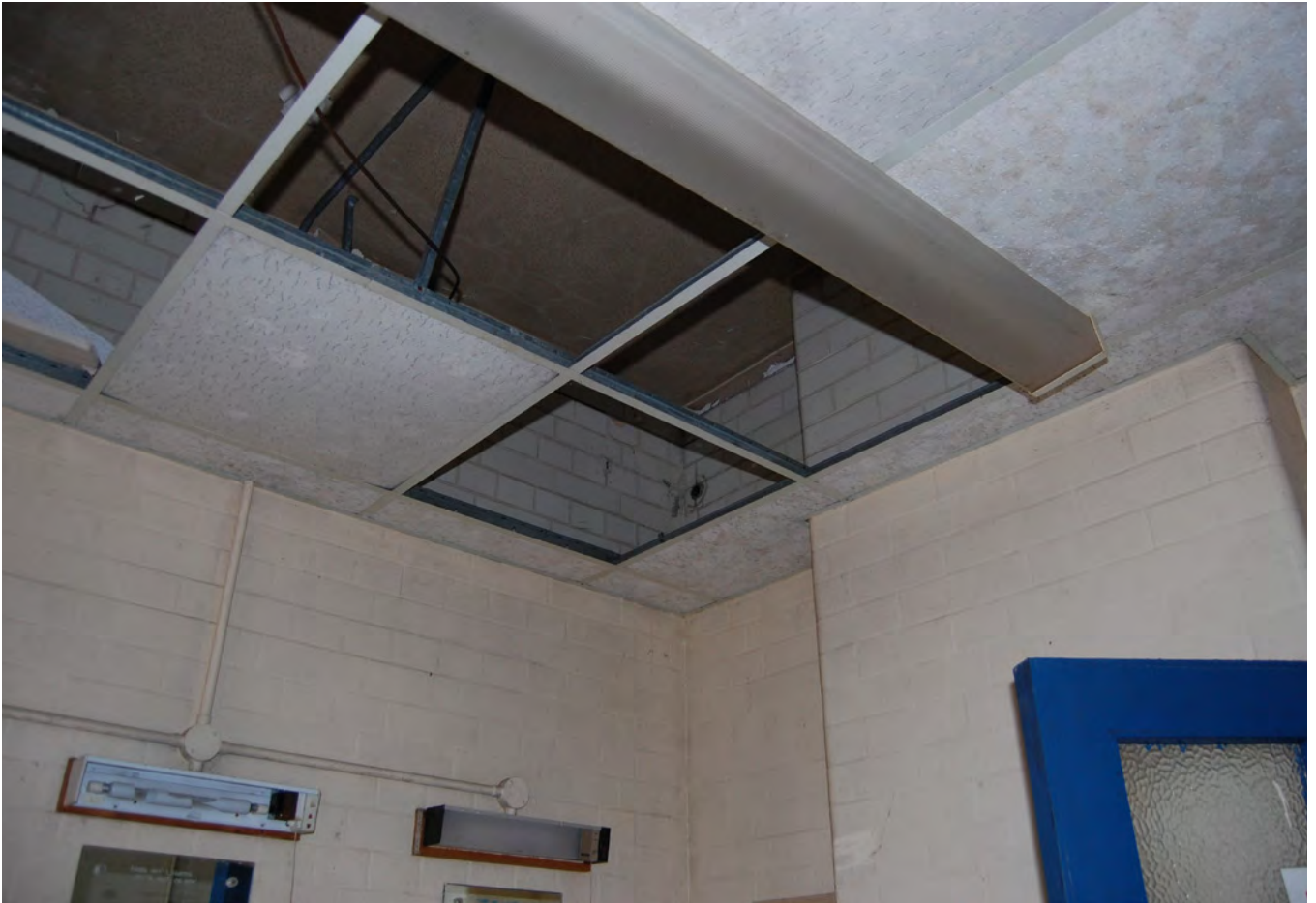
Plate 485.9 The glazed brickwork in the ablutions, visible above suspended ceiling
