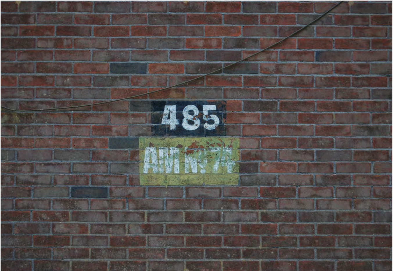
Plate 485.5 New and old building numbers
