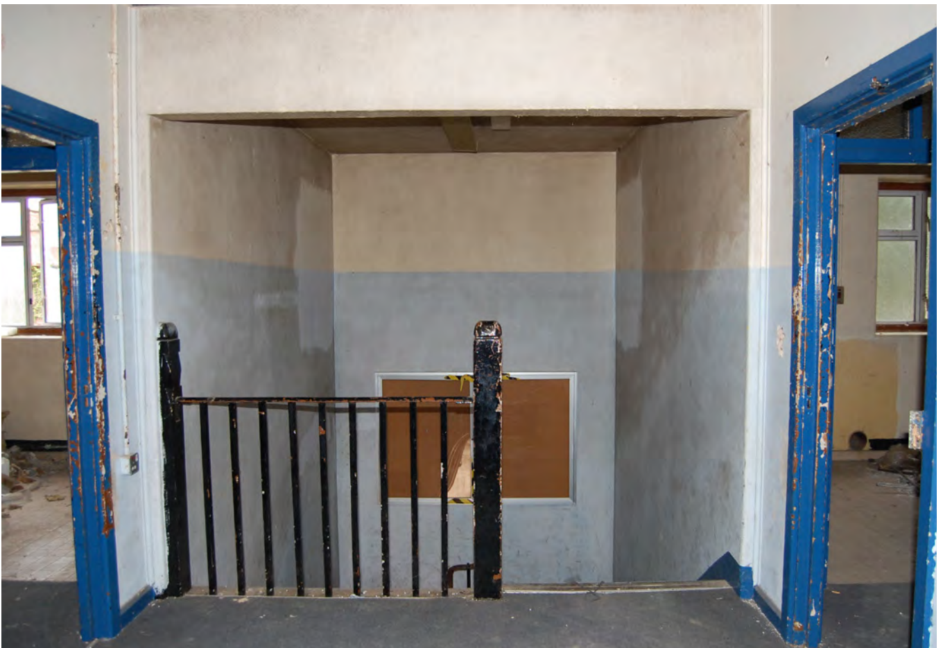
Plate 485.8 The stairwell, also showing the location of blocked lights to ablutions
