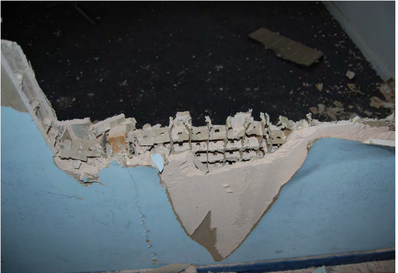
Plate 485.11 The partition panel construction
