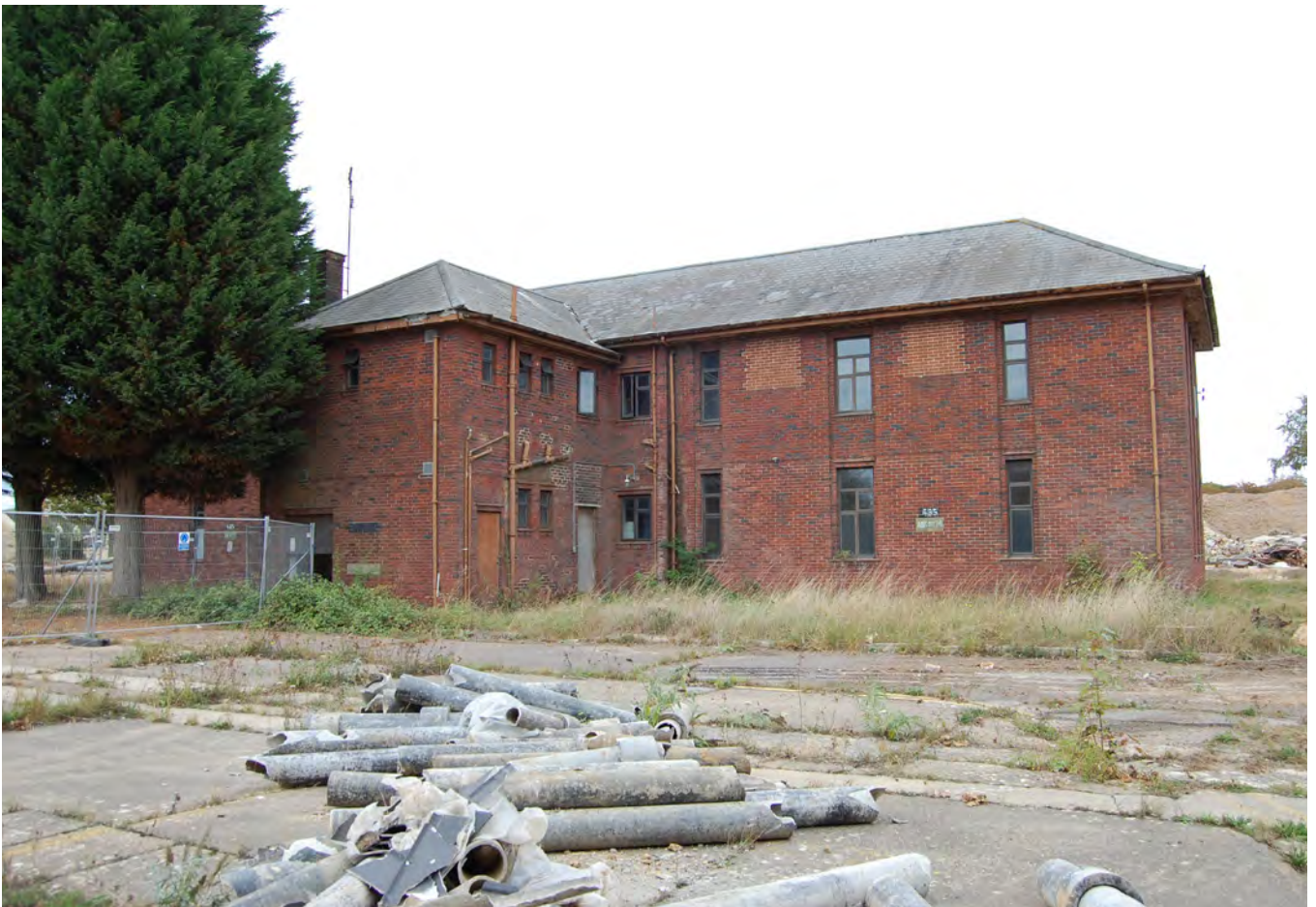
Plate 485.3 Rear, south, elevation: east end and ablutions block
