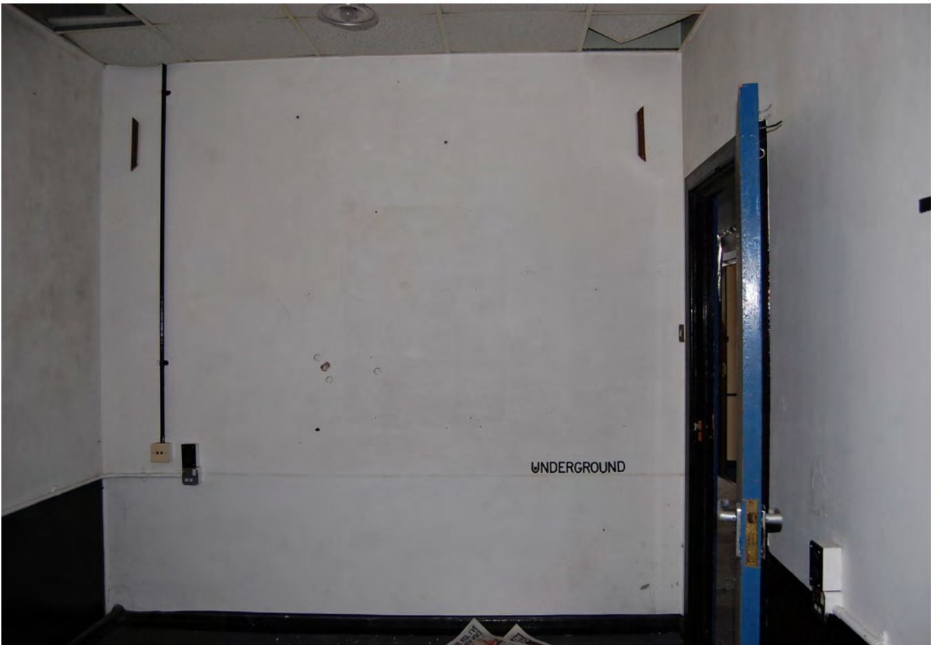
Plate 485.19 'Underground' stencil in a ground floor room
