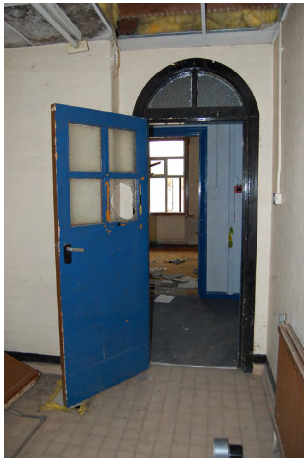
Plate 485.6 Example of a doorway between the ablutions and the corridor
