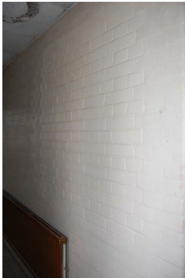
Plate 485.12 The blocked lights visible in the ablutions brickwork
