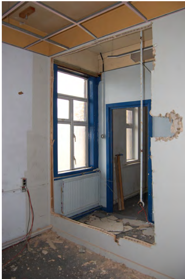
Plate 485.22 Western end of first floor landing following artwork removal
