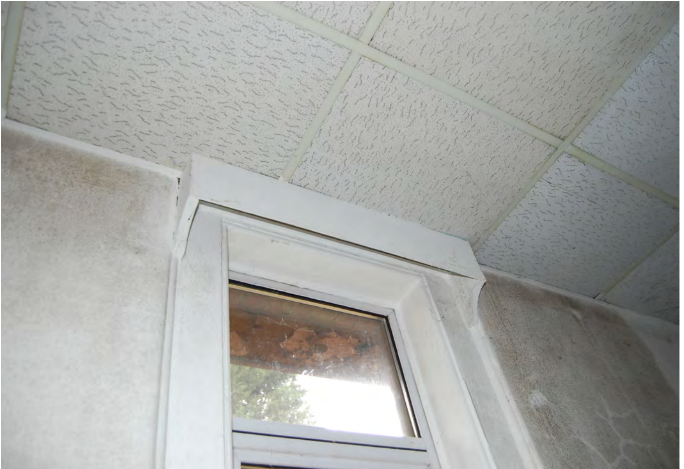
Plate 485.15 The suspended ceiling abutting a first floor window pelmet
