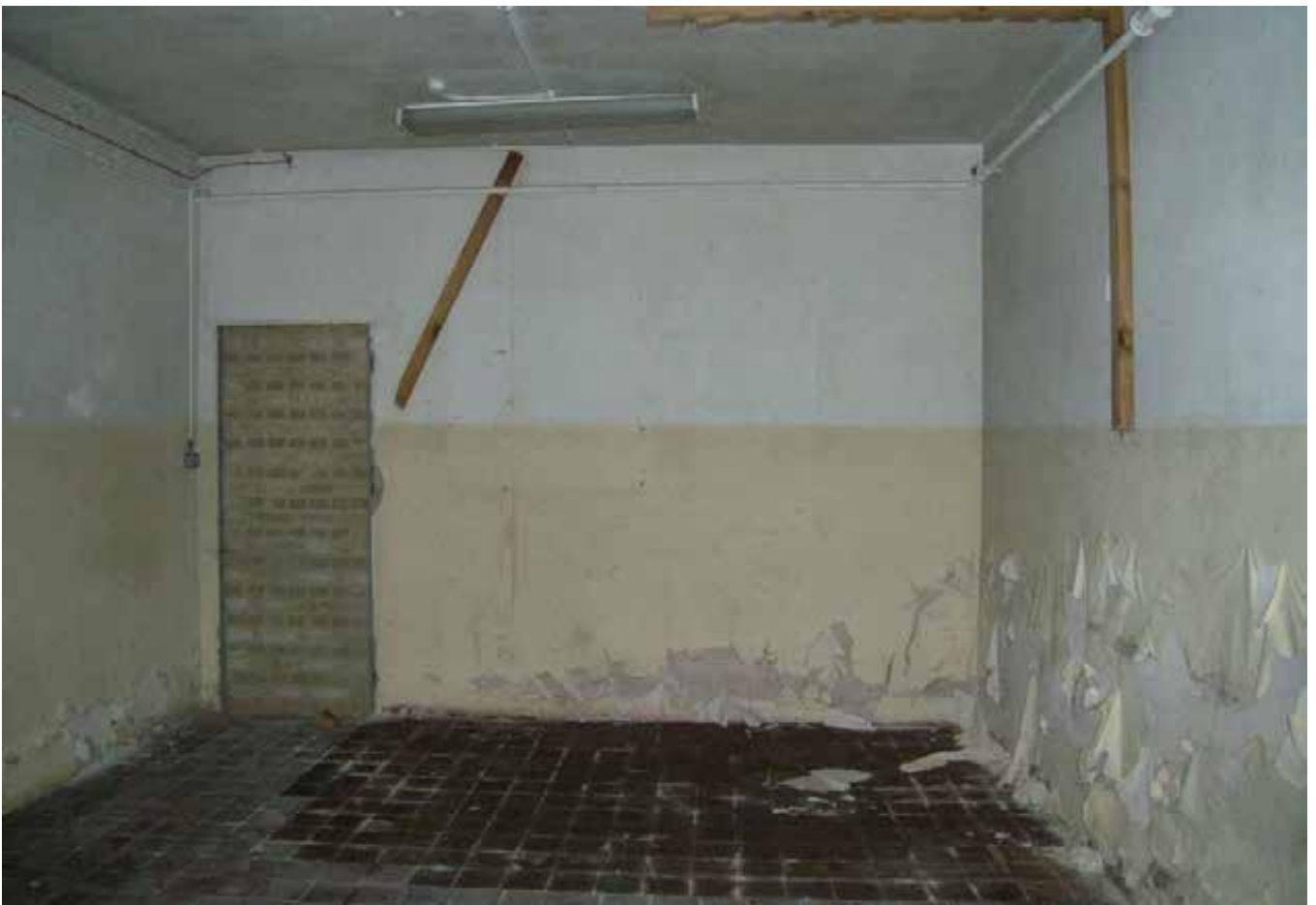
Plate 488.34 The former kitchen equipment store
