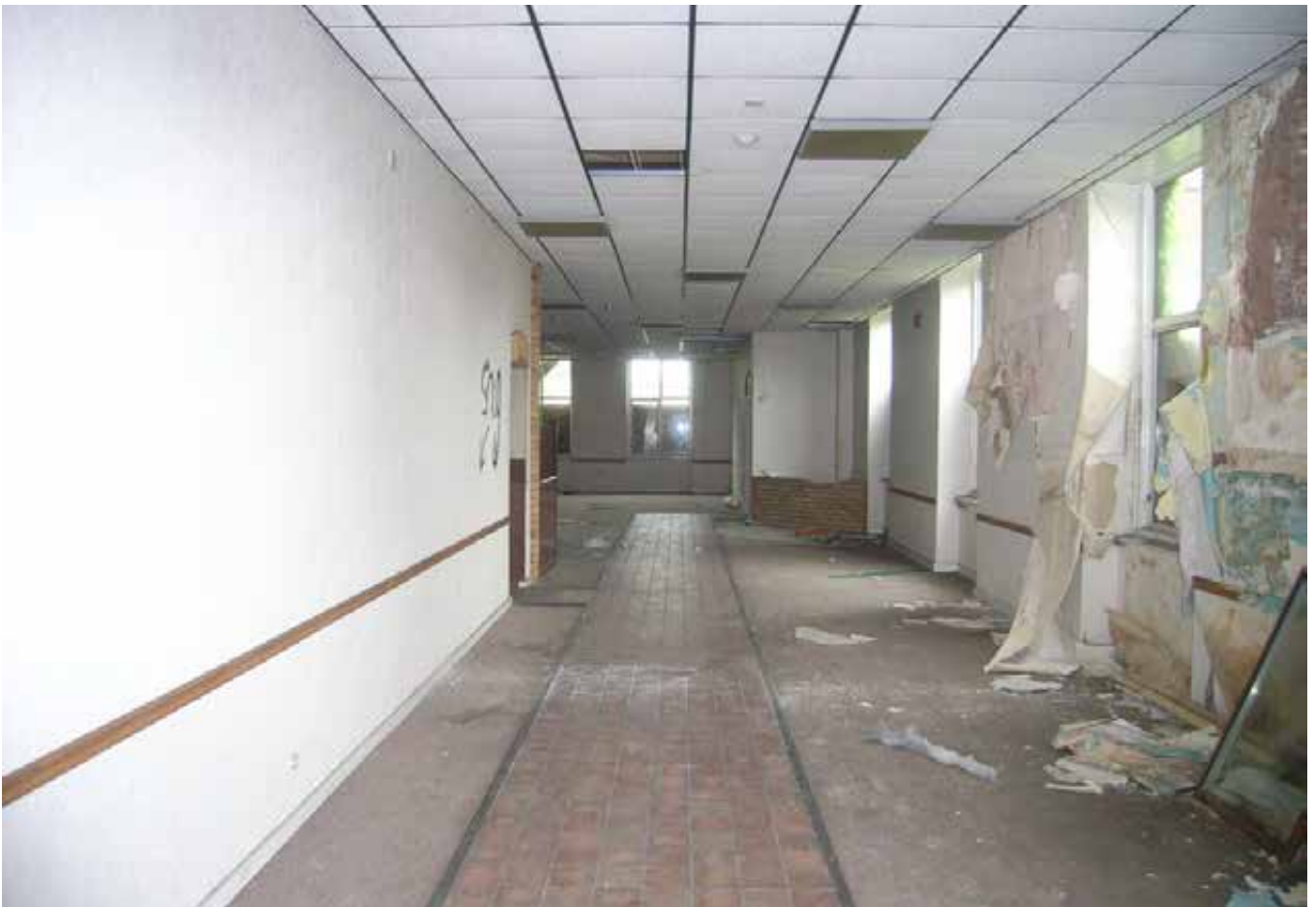
Plate 488.15 The corridor alongside the servery, looking towards the dining room
