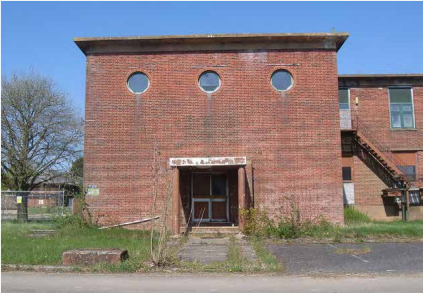
Plate 488.7 The west wing south elevation
