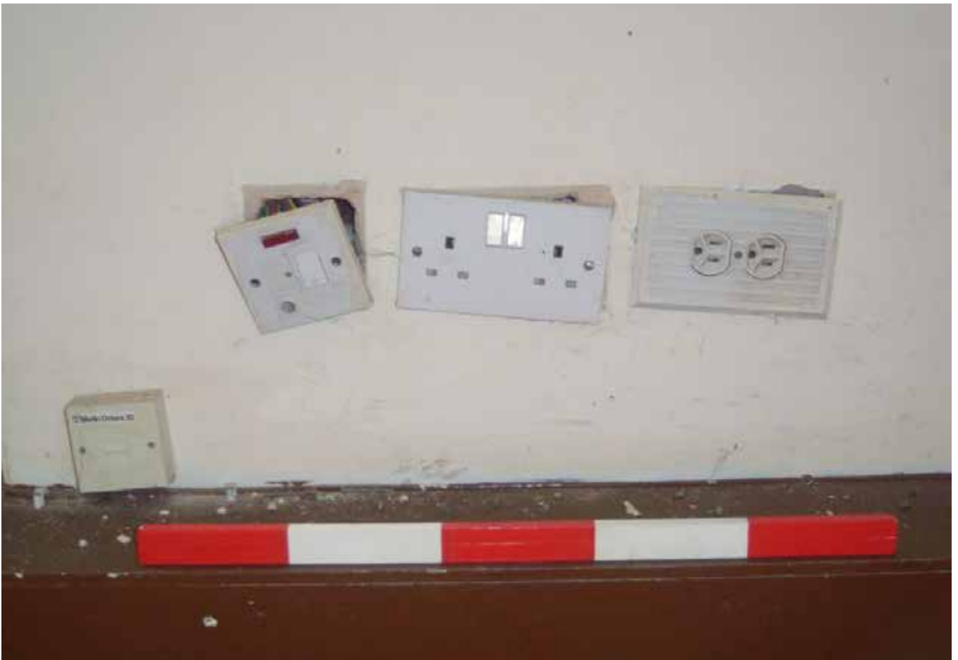
Plate 488.13 An example of the American and British power sockets
