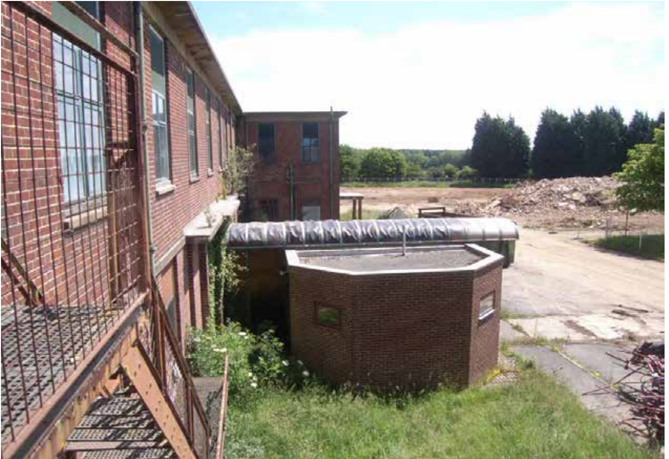
Plate 488.5 The entrance block extension
