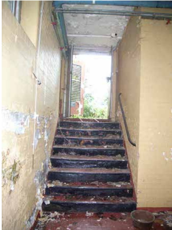
Plate 488.33 The steps from the boiler room to the yard
