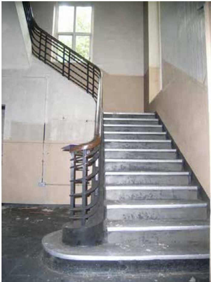
Plate 488.40 The staircase in the west wing
