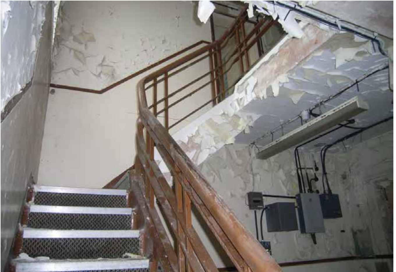
Plate 488.37 The staircase to the NAAFI dormitories
