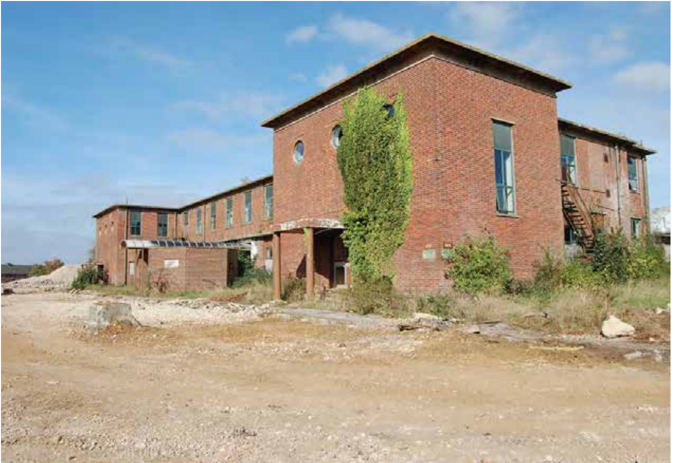
Plate 488.1 South (front) and east elevations
