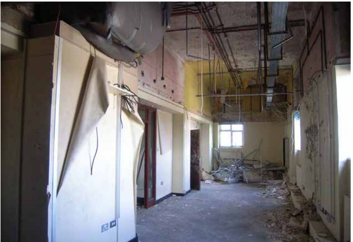
Plate 488.48 The former service rooms on the first floor
