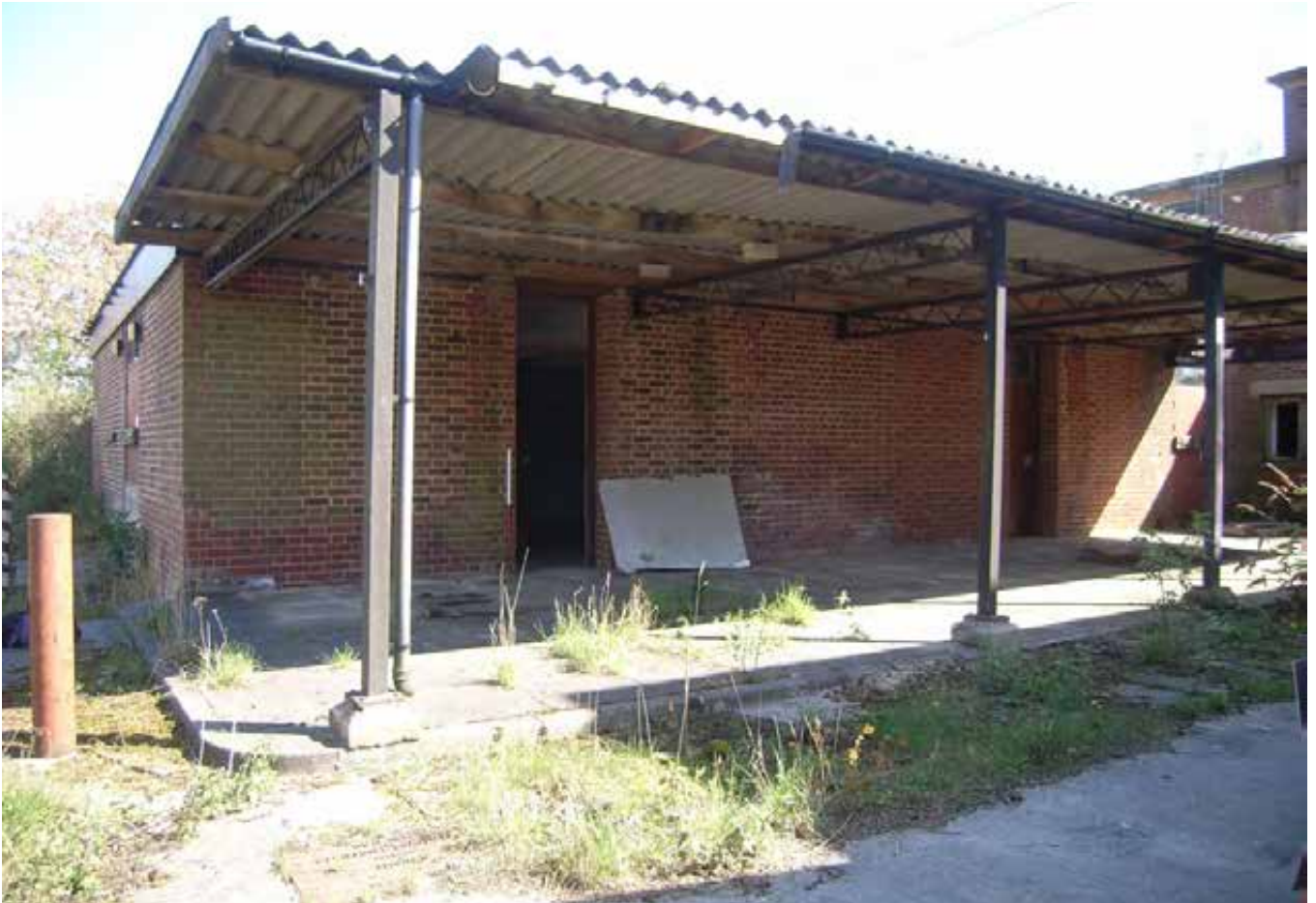
Plate 488.11 The covered area of the service yard
