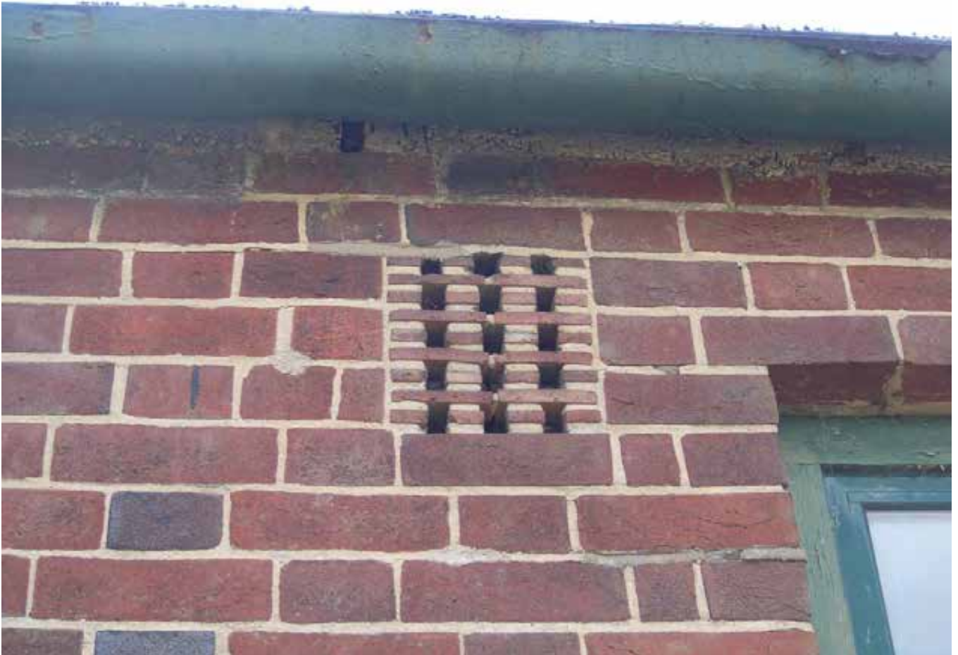
Plate 488.3 Example of a vent
