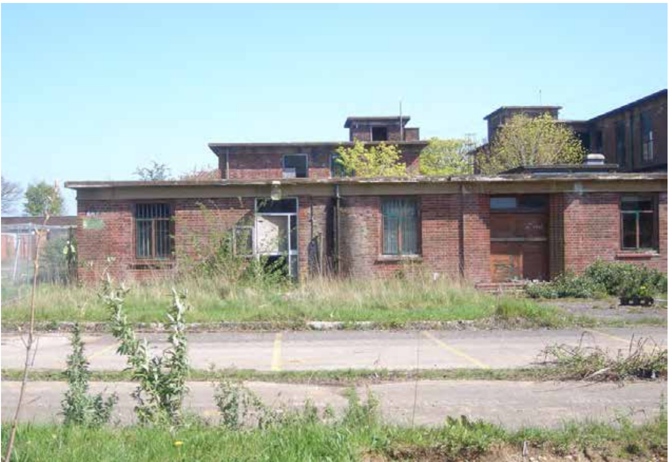
Plate 488.6 The two second storey tank rooms visible in the roofline
