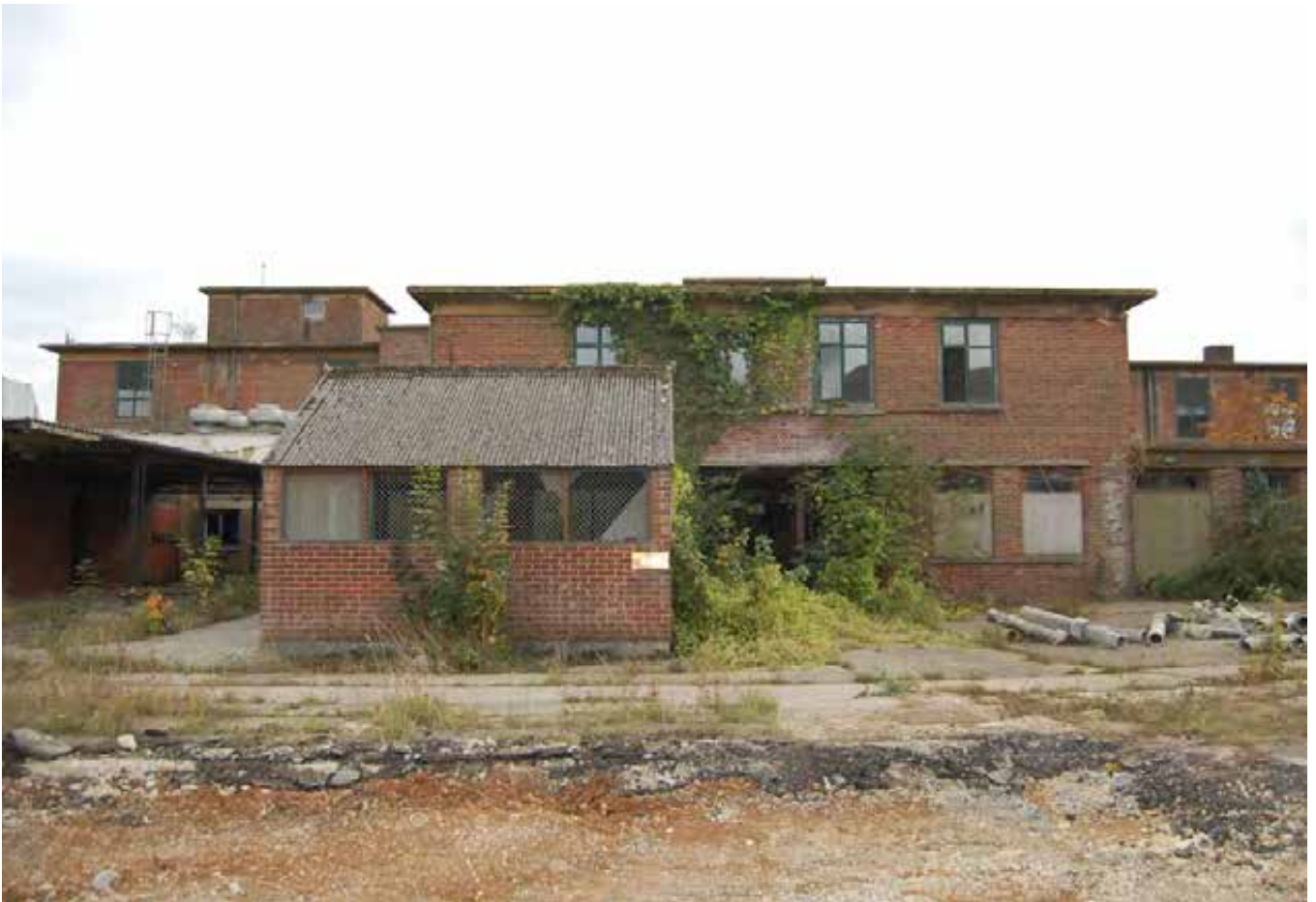
Plate 488.2 North (rear) elevation
