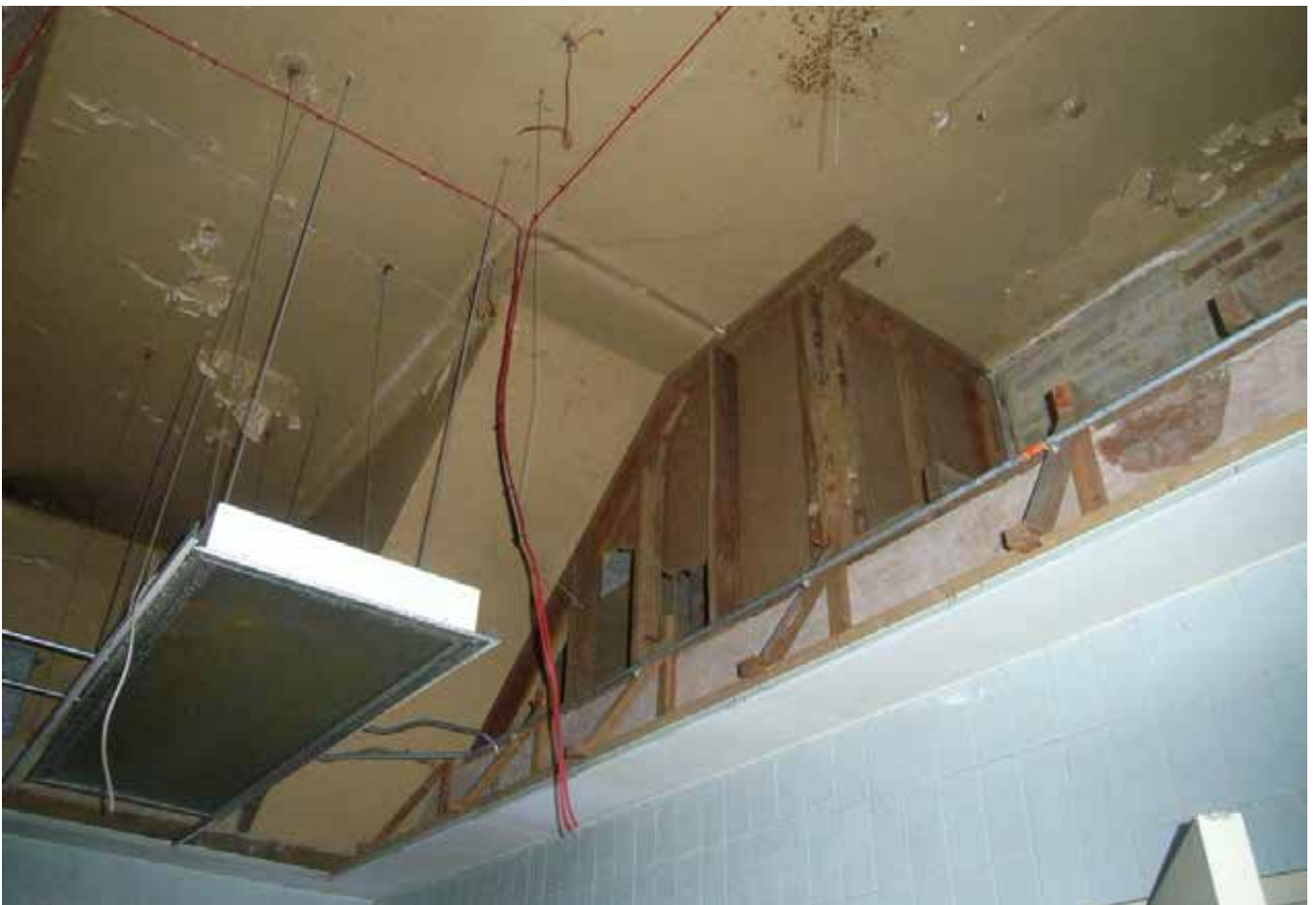
Plate 488.28 The former décor in the corridor and blocked-in staircase
