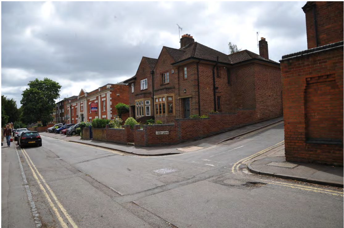
Pl.21: The view east along St. John's Road, with the Old Malthouse in the distance.
