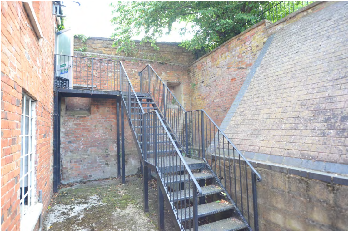
Pl.18: The eastern end of the rear yard with the brick wall and revetment of the terrace to the right. The area beyond the sloping section was once infilled with a building.
