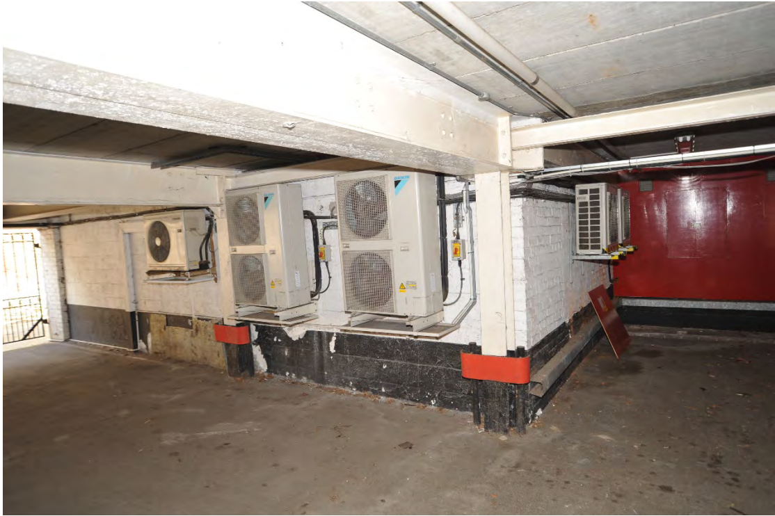
Pl.15: Another modernised portion of the ground floor.
