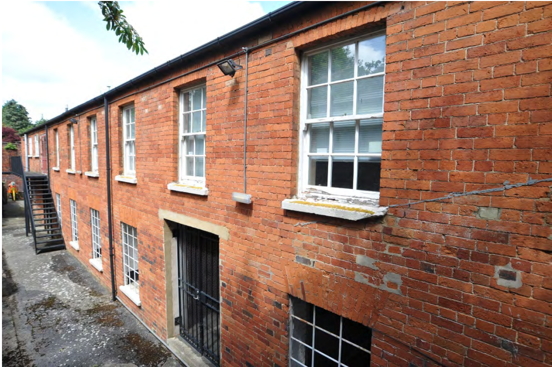
Pl.4: The rear elevation from the south-east.
