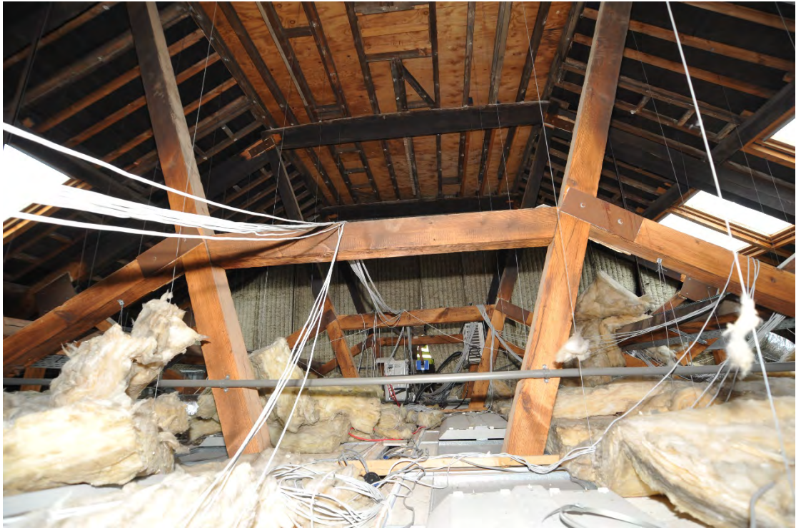
Pl.11: The tops of trusses visible above the ceiling in the main body of the building.
