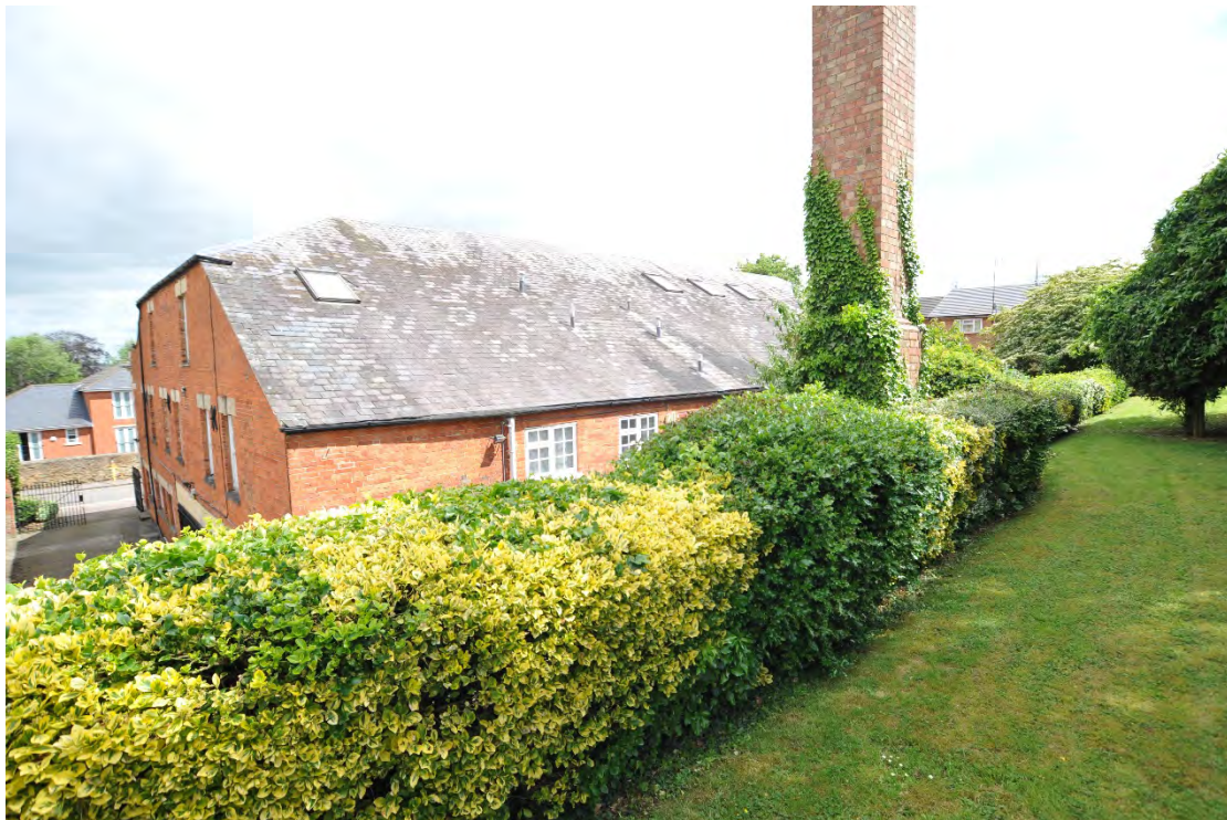
Pl.17: Main building from terrace, looking north-east; note mid-20 th century chimney.
