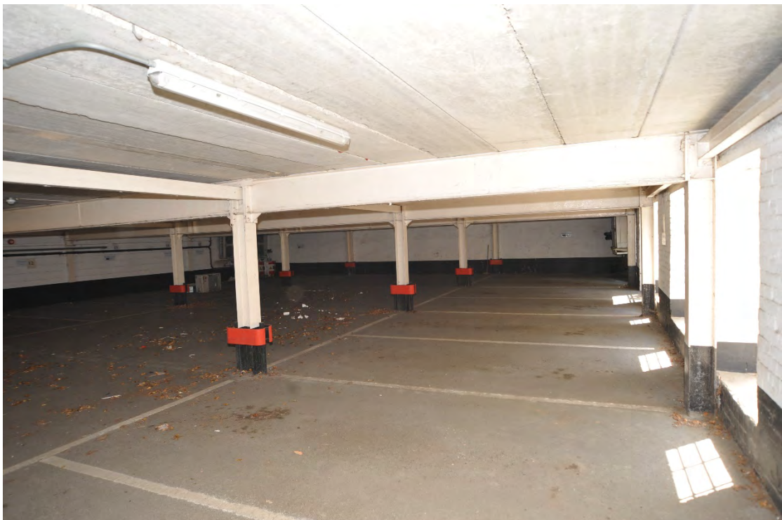
Pl.14: The bulk of the ground floor of the building is a covered car park; note the RSJ stanchions and concrete first floor, presumably dating to the engineering works phase.
