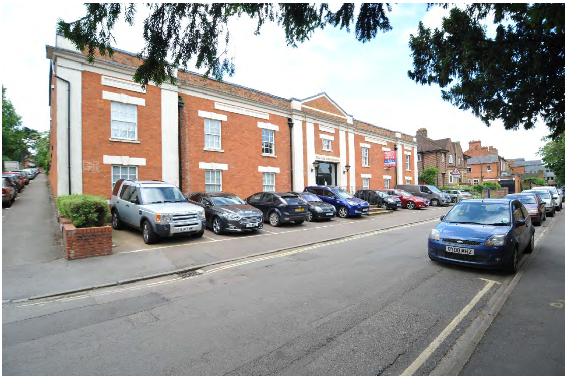
Pl.3: The front elevation from the north-east.
