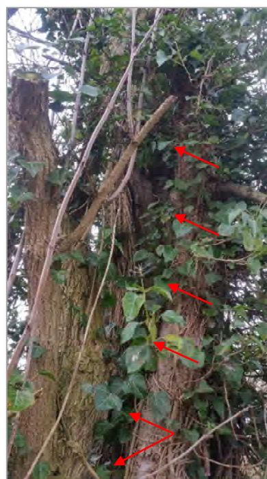
Figure 2 - Close up of stem of T16. The arrows indicate a large cavity partially hidden by ivy
