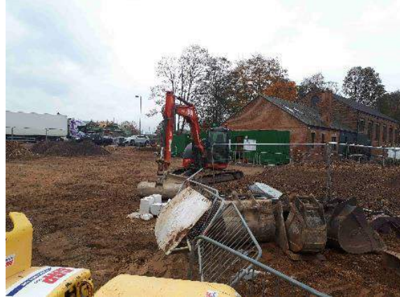
06.11.18 – View southwest from centre-west of northern boundary.
