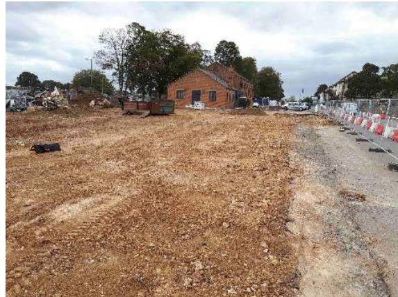
19.09.18 – View west from centre of northern boundary.
