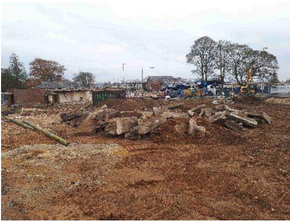
06.11.18 – View southeast from centre of northern boundary.
