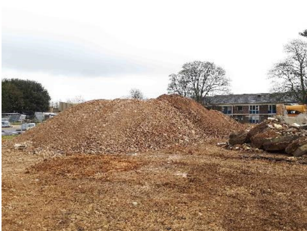
Stockpile of site-generated aggregate
