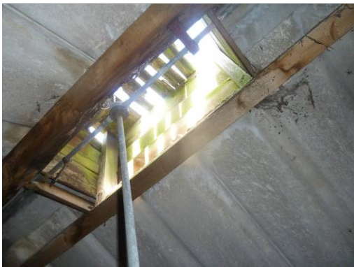
Open air vent in roof
