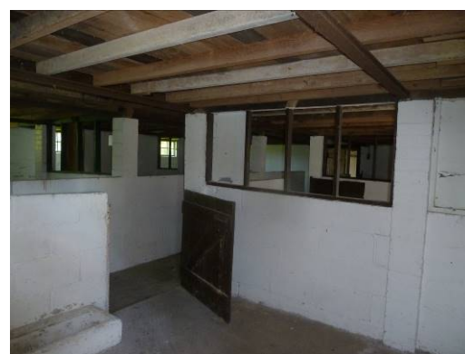
Ground floor showing flighted access and concrete floor
