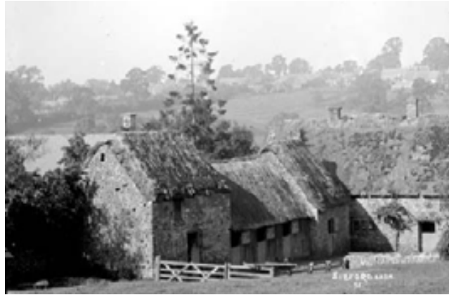
10.2 Outbuildings/barns to the Old House, viewed from Back Lane, looking towards Burdrop
