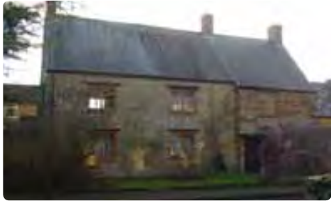
• The Old Post Office
