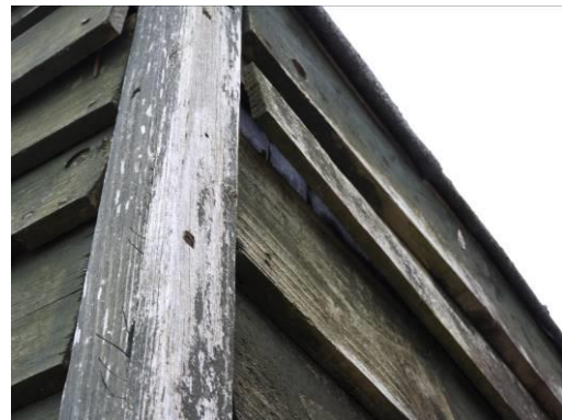
Fig. 17 Eaves and raised board
