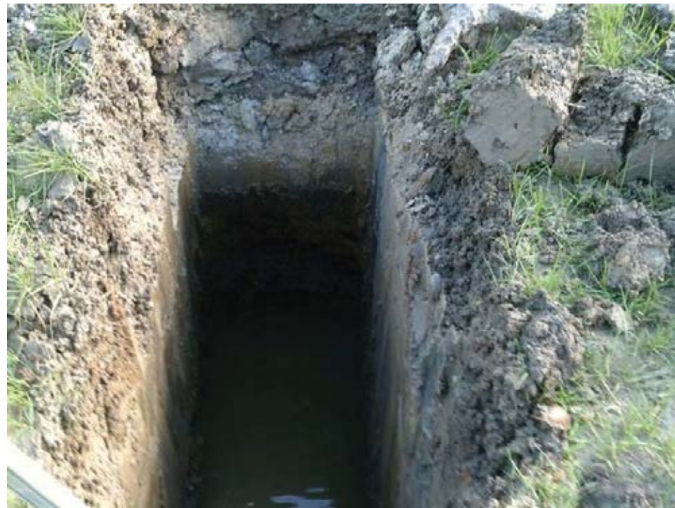
Trial pit 10 south face
