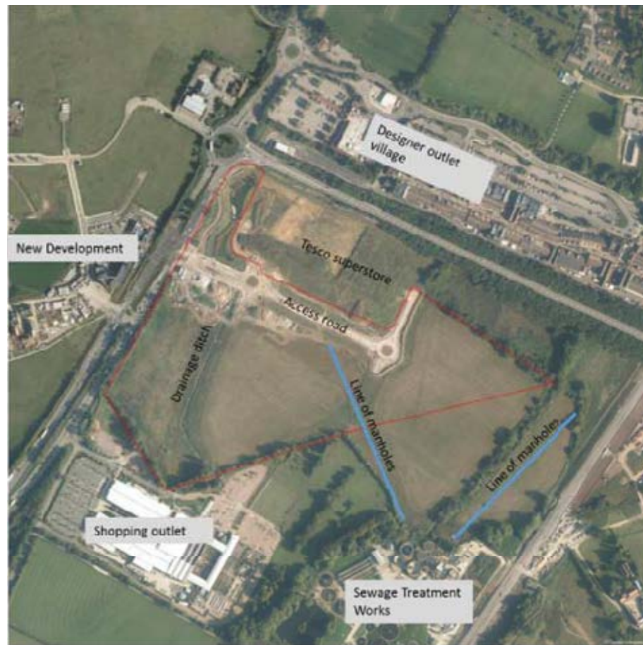
Figure 2-1 Annotated aerial photograph (base photograph dated 2015)
