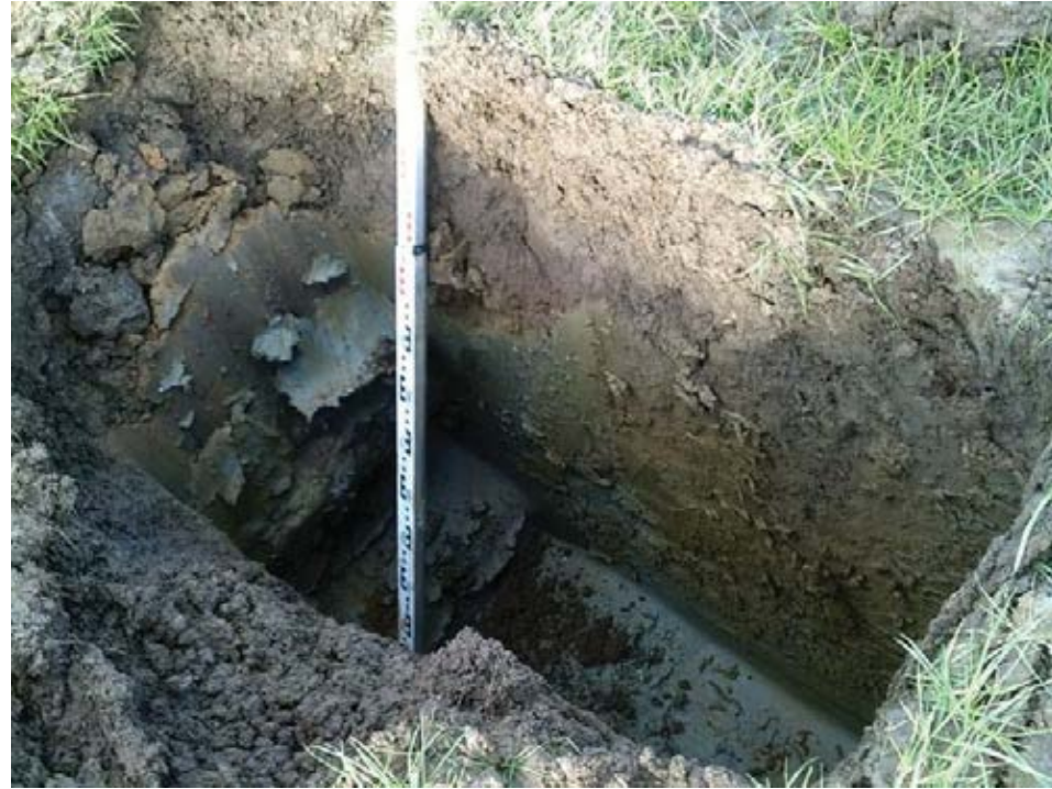
Trial pit 08 north face
