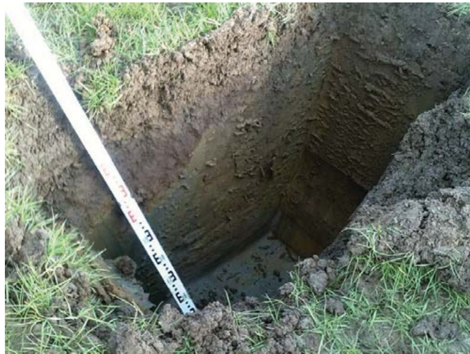
Trial pit 08 east face
