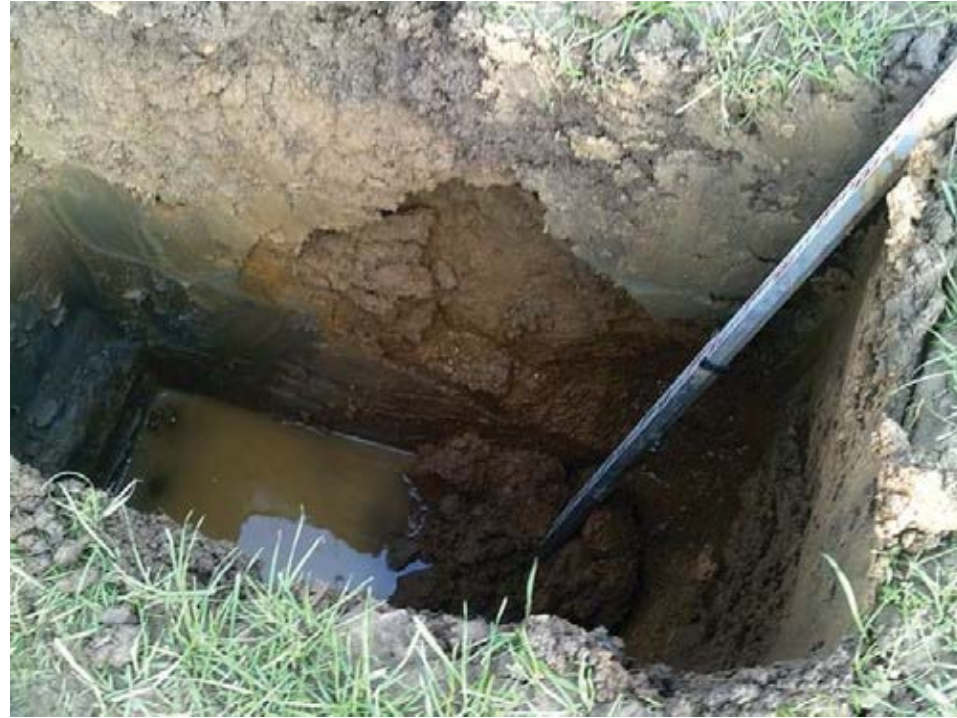
Trial pit 07 north face
