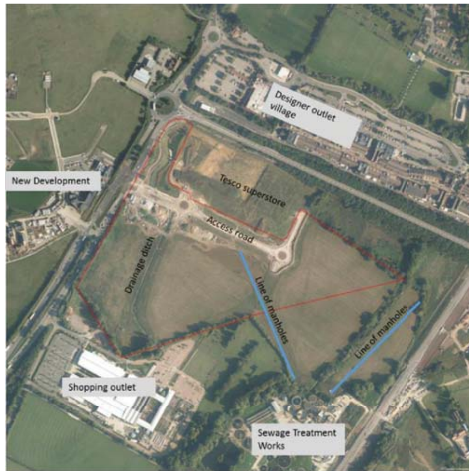
Figure 2-1 Annotated aerial photograph (base photograph dated 2015)
